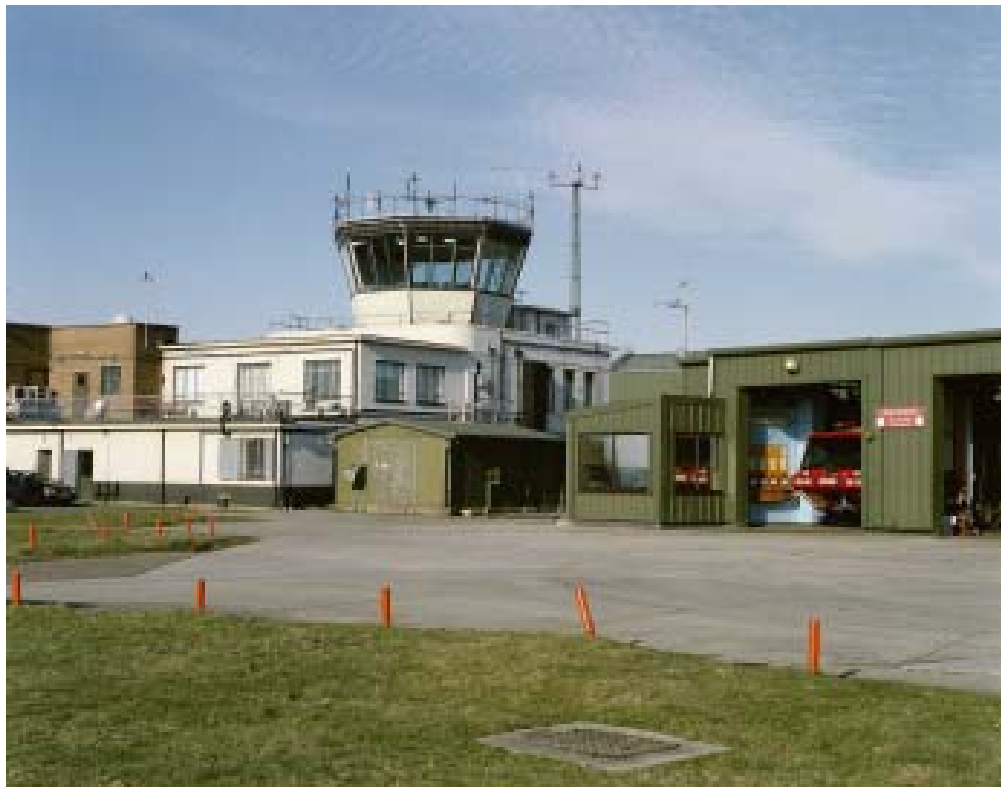
Figure 231 The Watch Office is a standard Air Ministry 2328/39 design constructed from 14 inch thick reinforced concrete walls. Originally on the ground floor were telecommunications and teleprinter rooms and a pilots' rest room, on the first floor, the meteorological officer's bedroom, control officer's rest room, and the signals office and in the front of the building the control room. It was also equipped with hydrogen bottles for weather balloons. Post-war modifications include the meteorological section and a briefing room to the left, an extension to the front to the front of the structure and the Visual Control Room on the roof. (c) English Heritage AA054410
