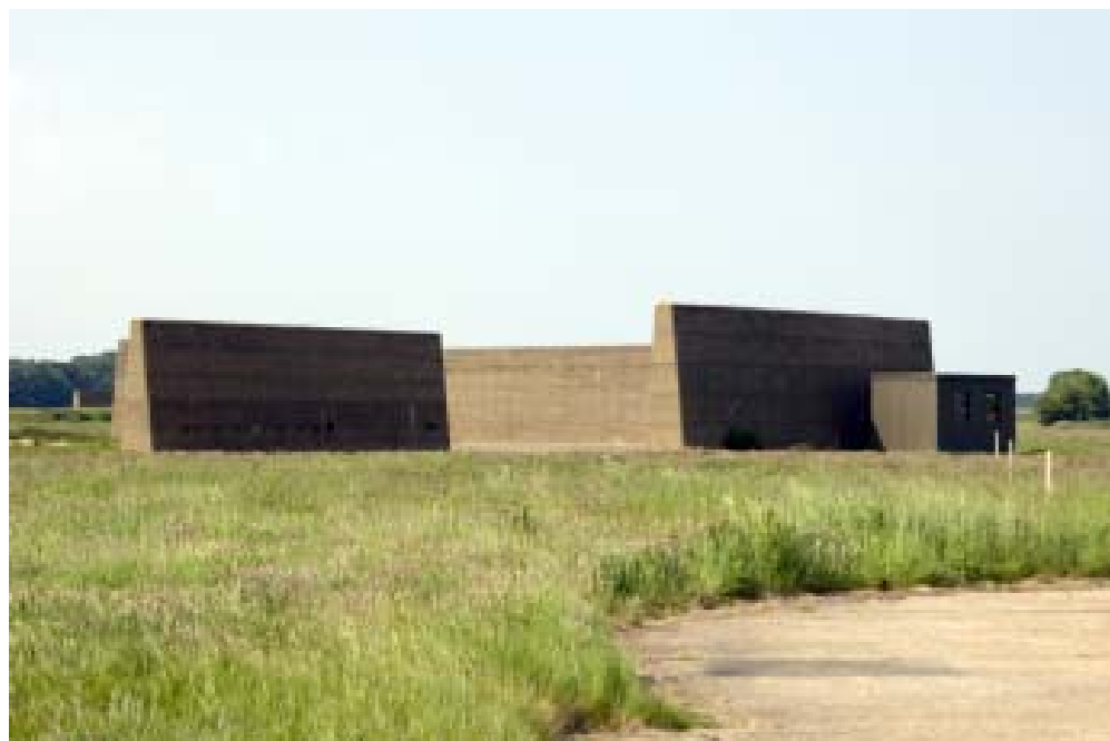
Figure 264 Late 1950s blast protection wall. (c) English Heritage DP027164
