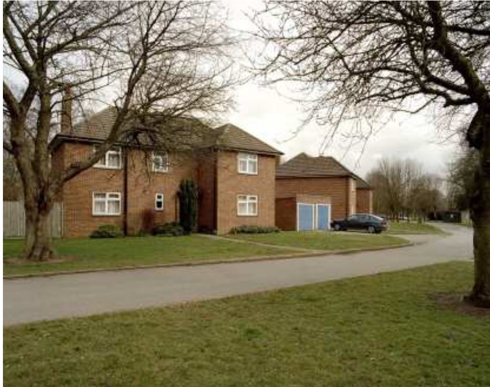
Figure 87 1950s Officers' housing, Barnby Road to rear of Officers' mess. (c) English Heritage AA054373
