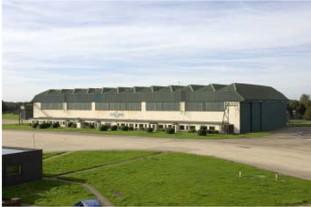
Figure 196 Hangar 3, C Type hangar from the Watch Office. (c) English Heritage DP035652
