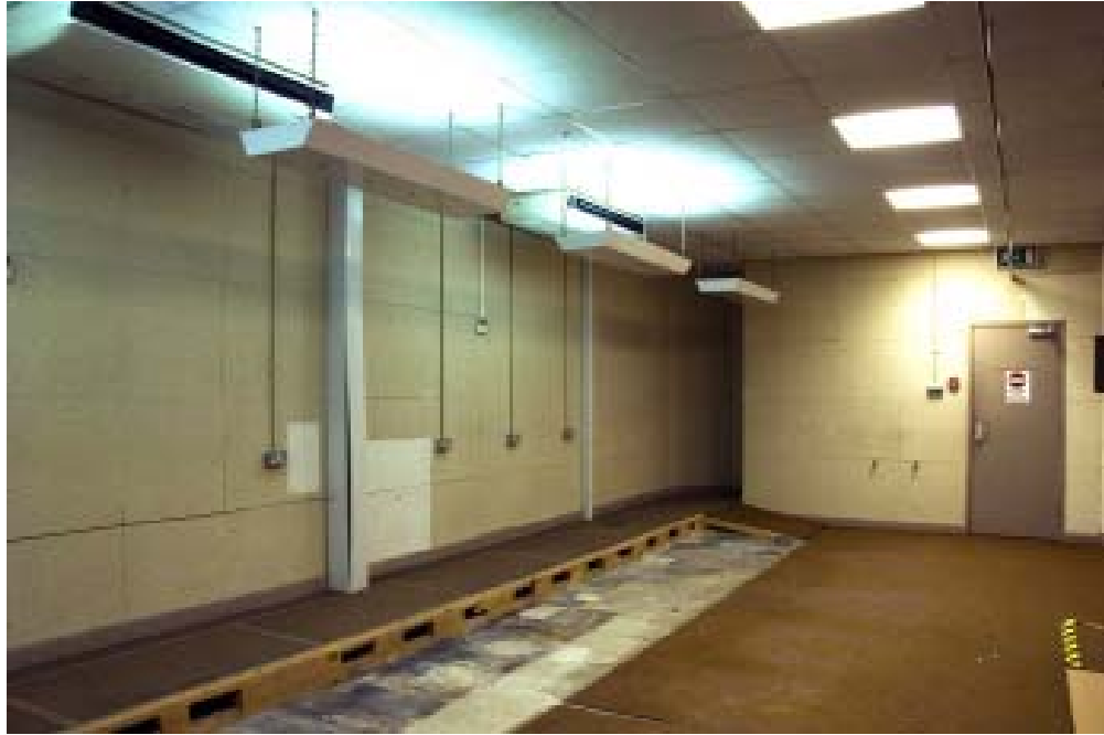
Figure 238 Watch Office, October 2006, stripped middle floor, formerly occupied by the approach controllers. (c) English Heritage DP035644
