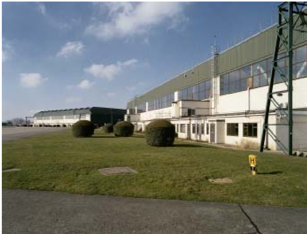
Figure 195 Hangar 2 and to the rear Hangar 3. All the hangars at Coltishall are standard Air Ministry Type C Protected Type, they have concrete lower walls with a glazed panel above and were originally clad in asbestos sheeting. As may be seen in the far hangar the asbestos sheeting roof was left exposed above the doors. (c) English Heritage AA054396
