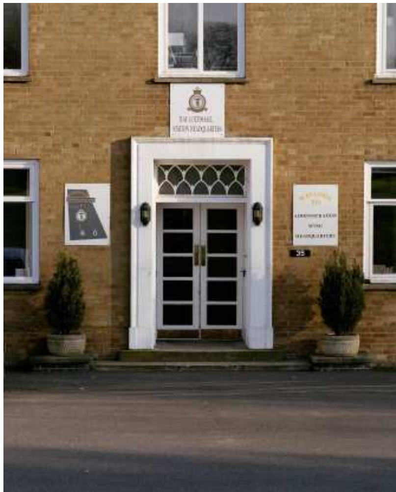
Figure 16 Station Headquarters, main entrance. (c) English Heritage AA054463
