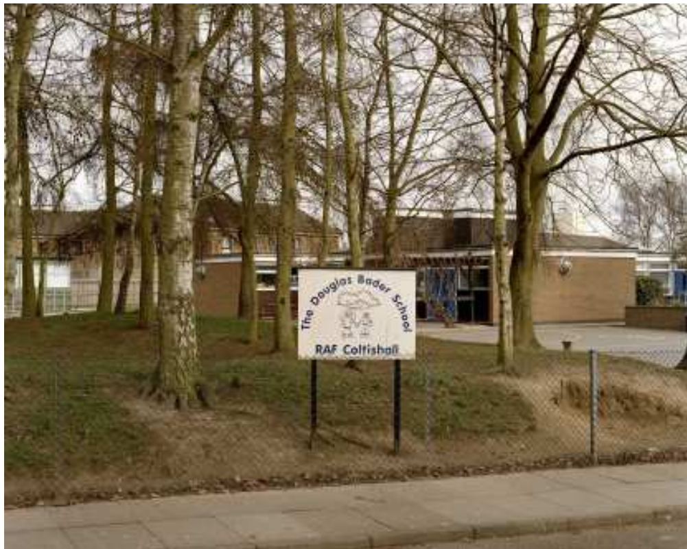
Figure 94 The Douglas Bader School, Filby Road. (c) English Heritage AA054375
