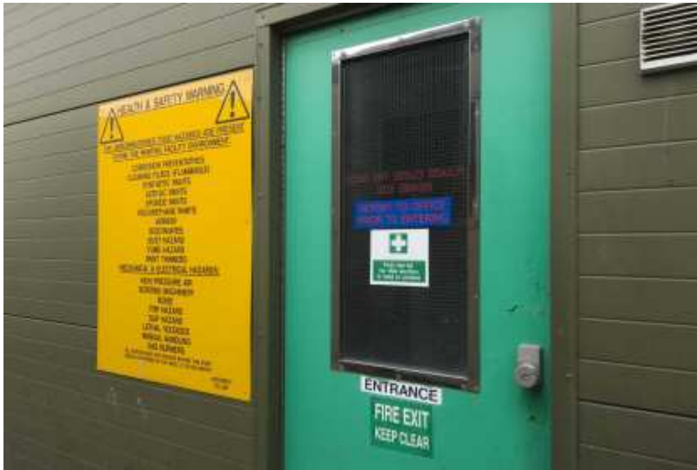
Figure 132 Jaguar Paint Facility, entrance. (c) English Heritage DP027179
