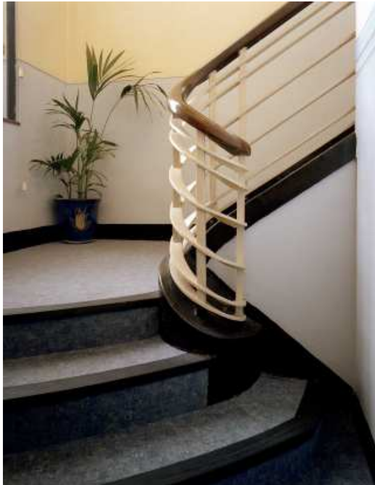
Figure 62 The Junior Ranks Mess, detail of stair rail. (c) English Heritage AA054456
