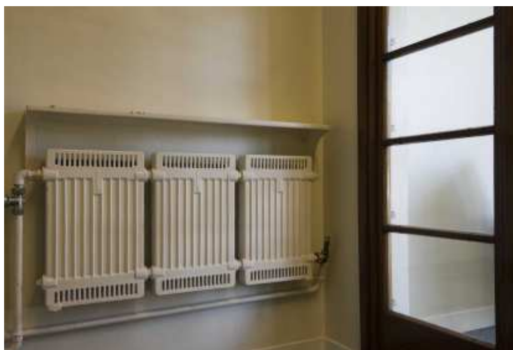
Figure 77 Hanbury block, main entrance, detail of 1950s radiators. (c) English Heritage DP027333
