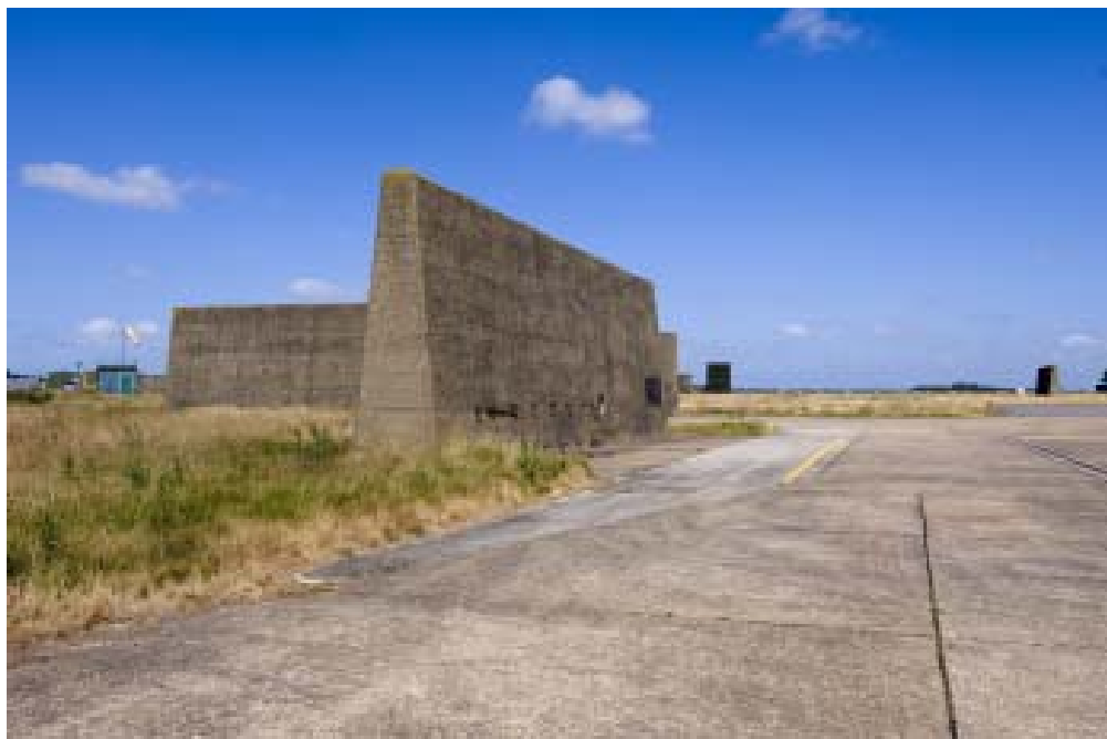
Figure 260 Late 1950s blast protection walls. (c) English Heritage DP027355
