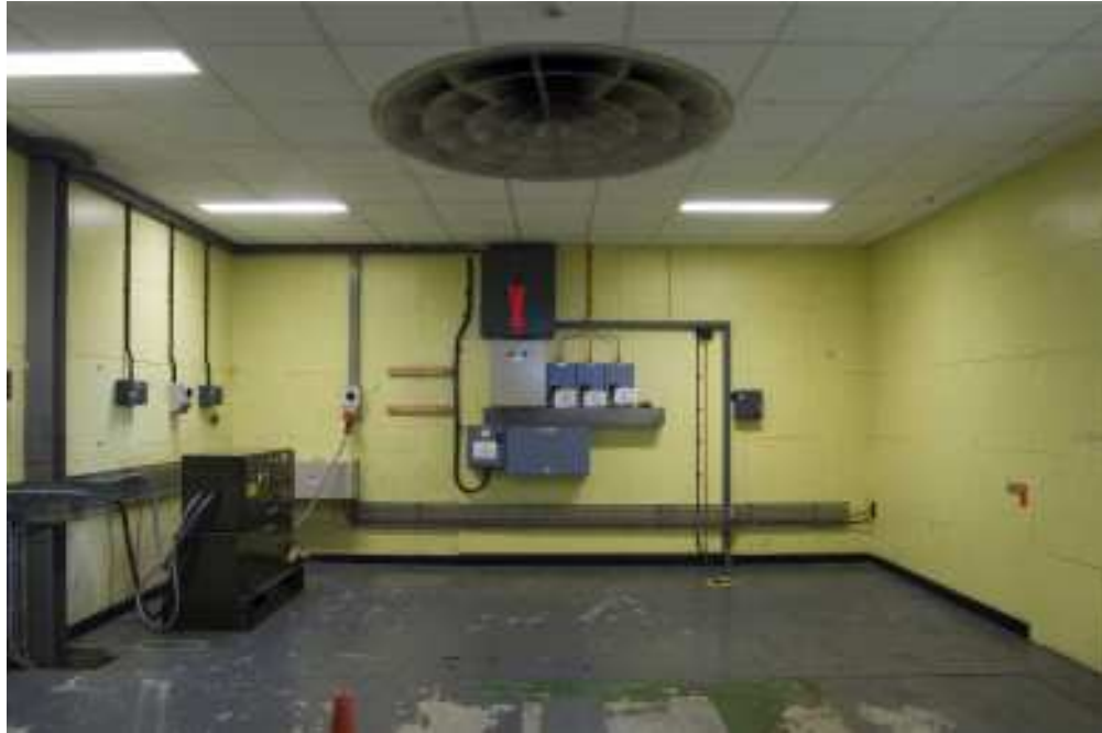
Figure 145 Building 295, Headquarters Electrical Engineering Squadron. (c) English Heritage DP029245
