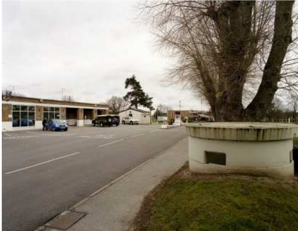
Figure 11 Main gate, showing the original guard room whose open veranda has been partly enclosed. To the right is a prefabricated Yarnold Shelter, these were constructed in the 1980s to guard against possible terrorist attack. (c) English Heritage AA054382
