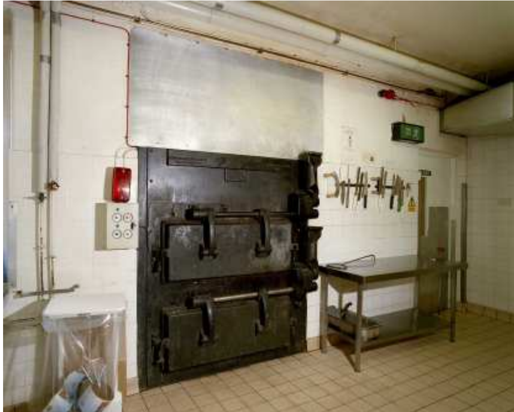
Figure 65 The Junior Ranks Mess, kitchen, west end, late 1930s Collins Cantilever Oven by Thomas Collins Co Ltd, Telephone Bristol 57061, it was originally coal fired oven. (c) English Heritage AA054452
