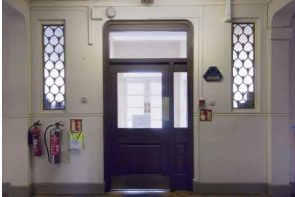
Figure 17 Station Headquarters, main door from rear. (c) English Heritage DP027352
