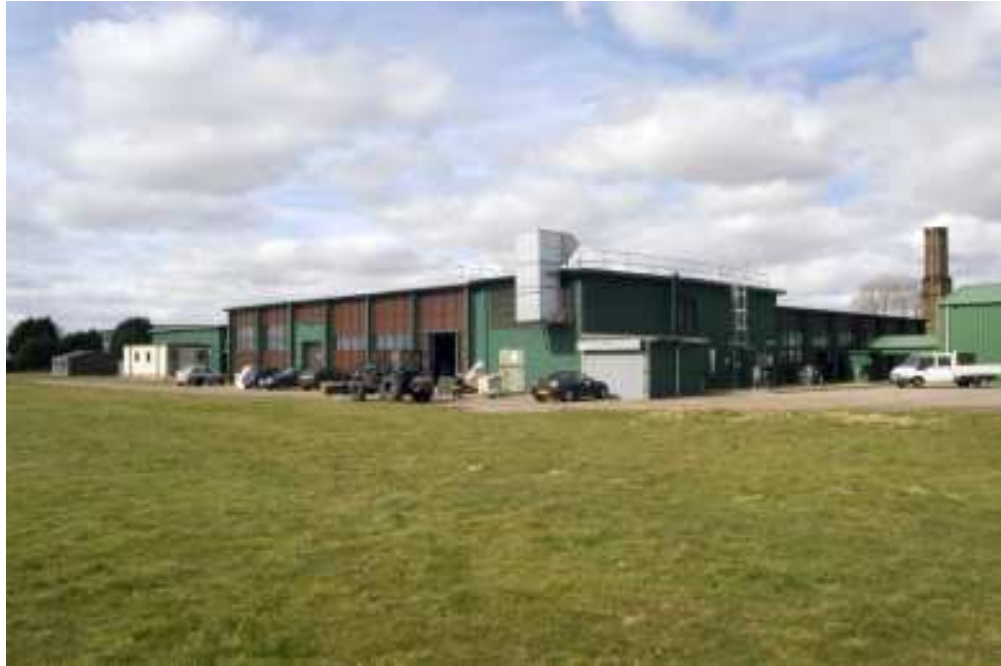
Figure 137 Building 295, Headquarters Electrical Engineering Squadron. This building was constructed at the beginning of the 1950s to maintain and service the increasingly complex electronic equipment carried by post-war jet aircraft. (c) English Heritage DP029240
