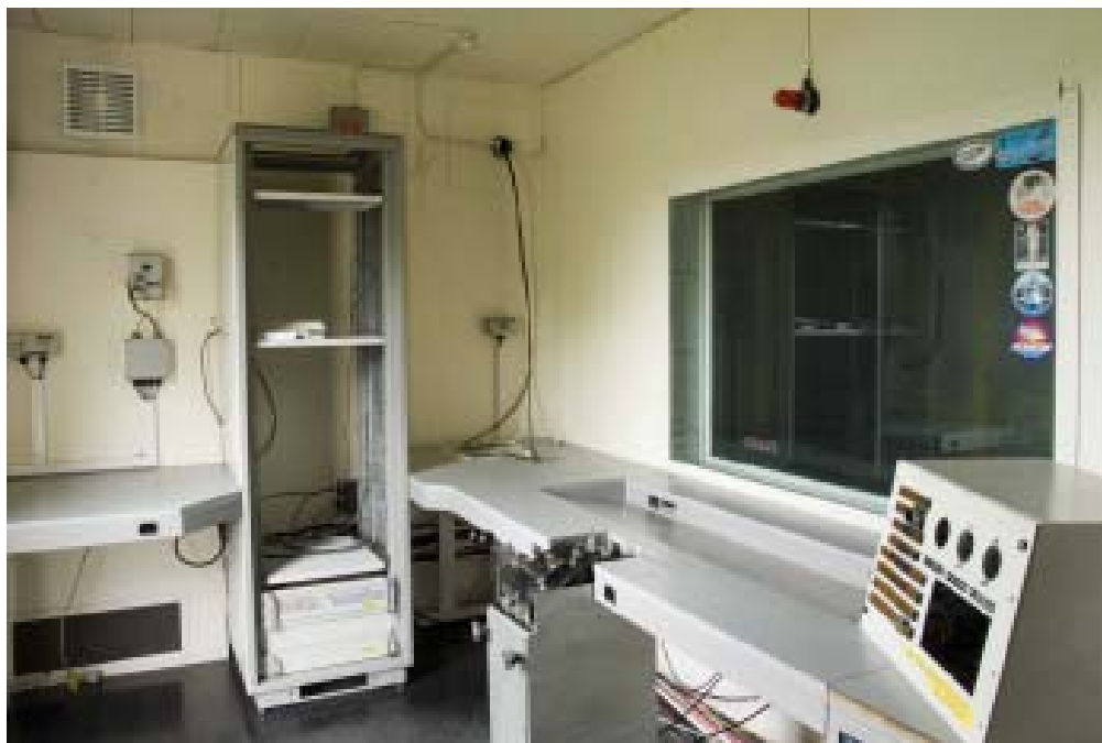
Figure 161 Uninstalled Engine Test Facility (UETF), control room. (c) English Heritage DP027323
