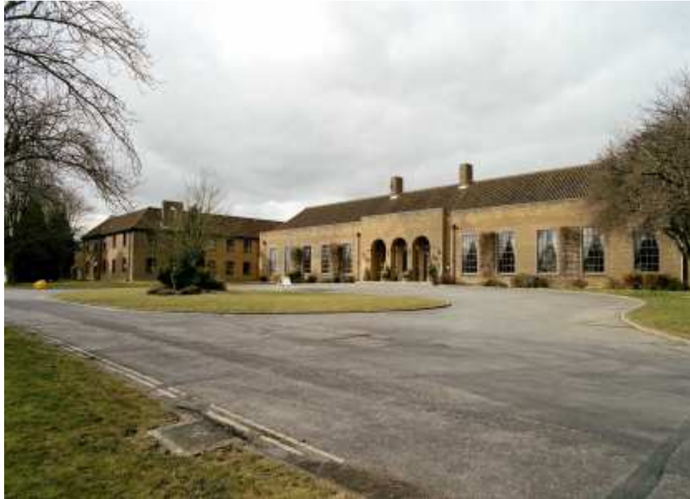
Figure 30 Building 50, The officers' mess, this fine neo-Georgian style building is typical of the care taken over the design of many permanent RAF airfields during the late 1930s. Traces of wartime camouflage may still be seen on its walls. (c) English Heritage AA054416
