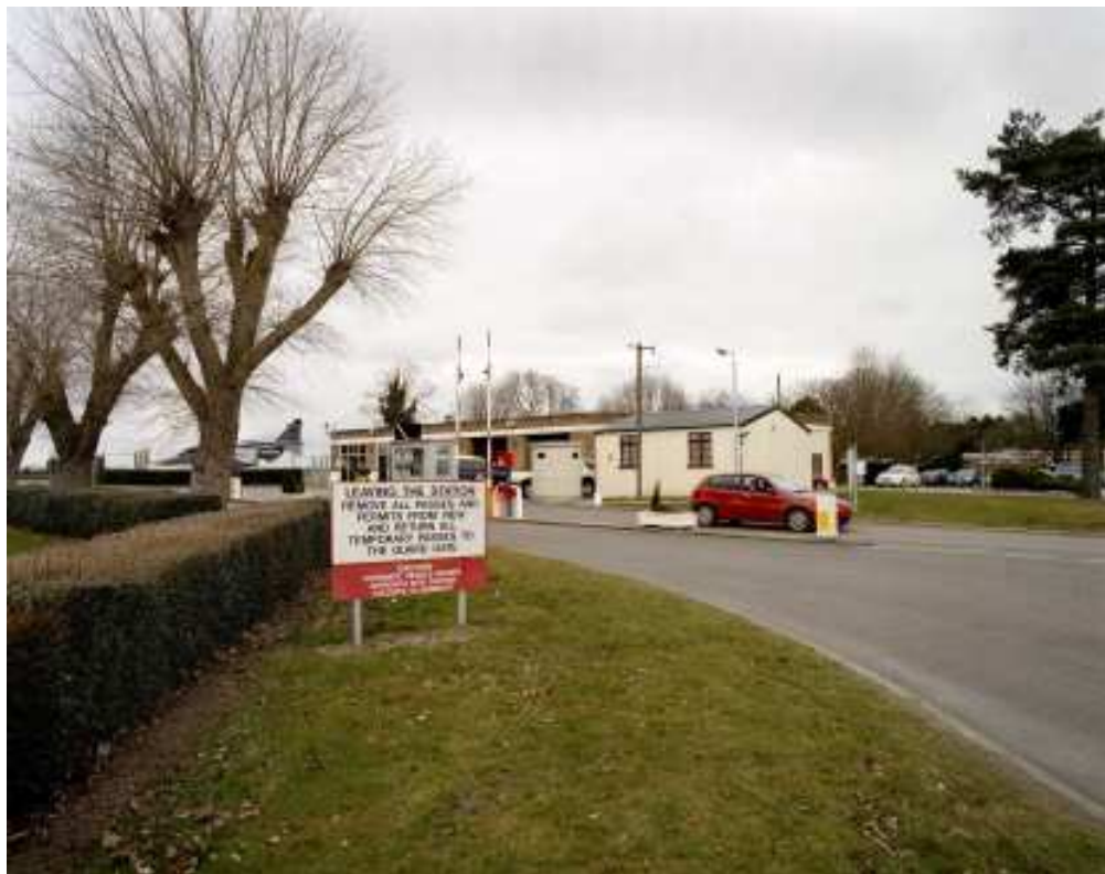
Figure 12 Main gate, looking outwards. (c) English Heritage AA054383
