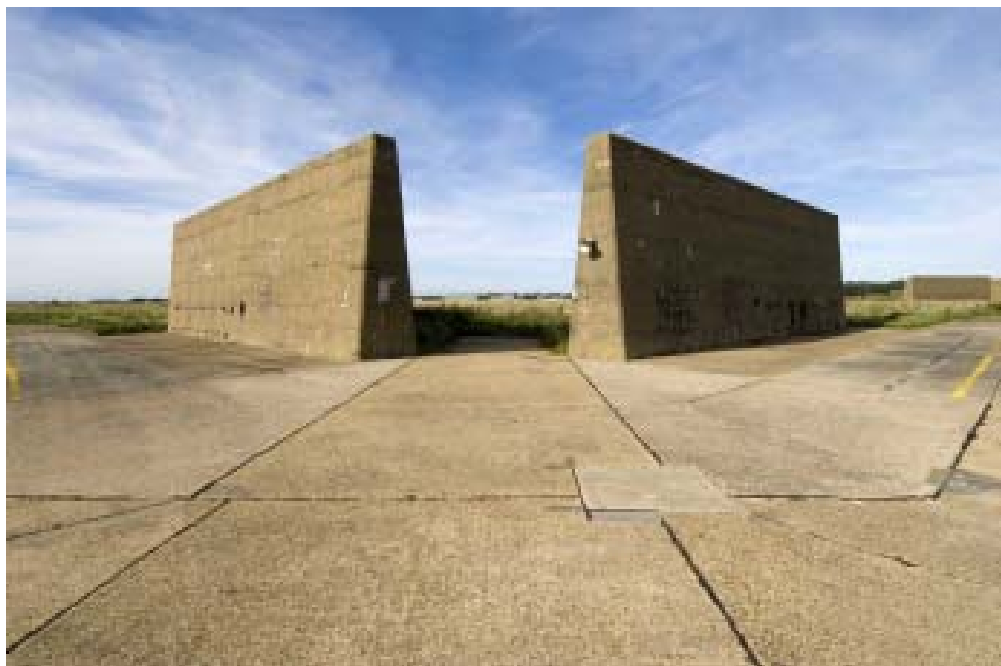
Figure 253 Blast walls 48 and 49. Late 1950s blast protection wall, between each blast wall is rectangular hardstanding that was used for parking a fuel bowser. This was connected to refuelling hoses through the circular hole in the centre of the blast walls, the hoses were supported on steels hoops set into the wall. (c) English Heritage DP035647
