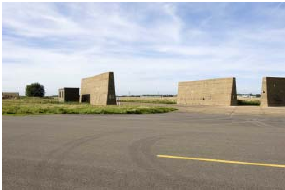
Figure 255 Late 1950s blast protection walls, eastern group walls 48 and 49 looking west. (c) English Heritage DP035649
