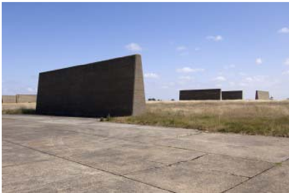
Figure 263 Late 1950s blast protection walls. (c) English Heritage DP027357
