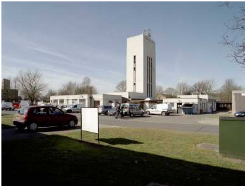
Figure 29 Station water tower. (c) English Heritage AA054435
