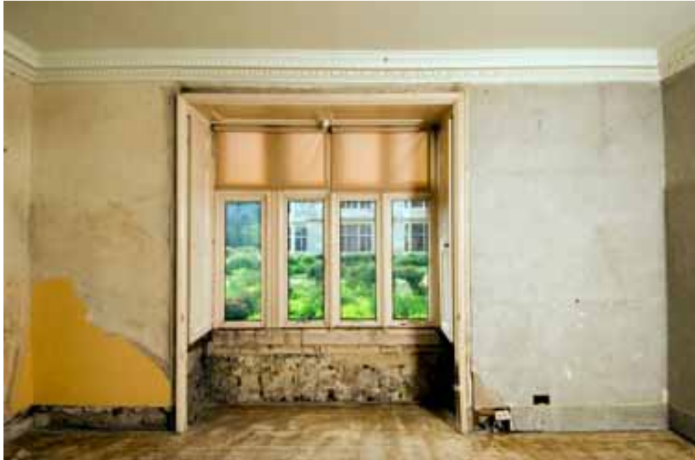
Figure 9 A photograph of the south wall (NMR: DP029537)
