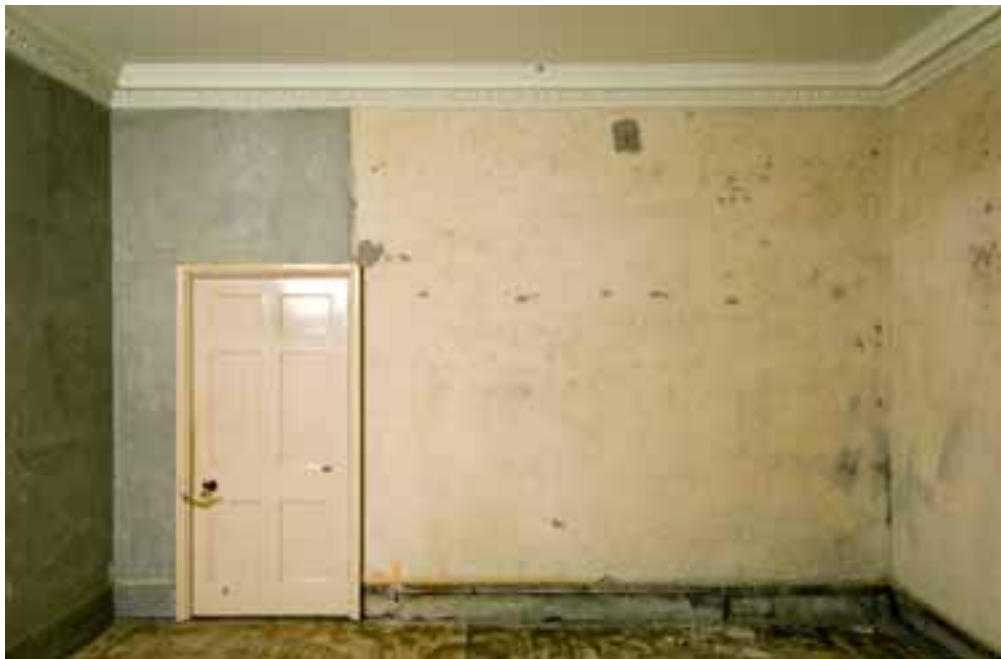
Figure 10 A photograph of the west wall (NMR: DPO29536)
