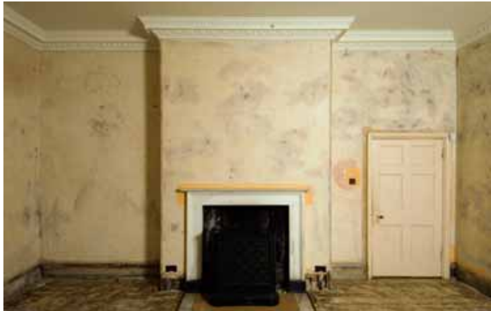
Figure 11 A photograph of the north wall (NMR: DP029539)
