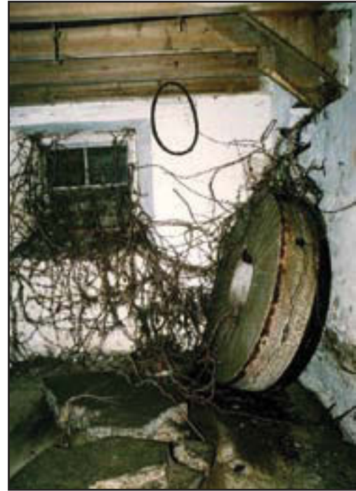
Figure 21. Interior, first floor of mill from east south east, showing composition runner-stone with fragments of another lying on the floor. [OP04338]
