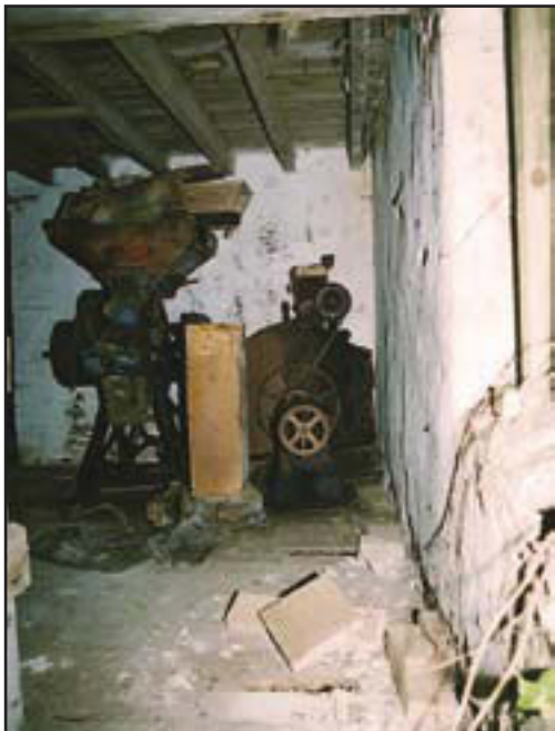
Figure 22. Interior, first floor of mill, from south, showing machines in the north-east corner. The oats crusher is to the left. [OP04339]
