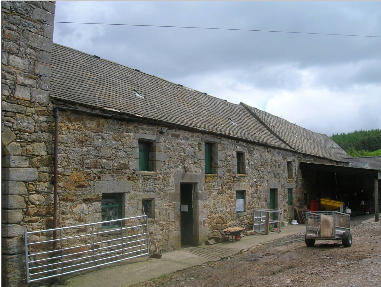
Figure 5: East range; taken from the north-west
