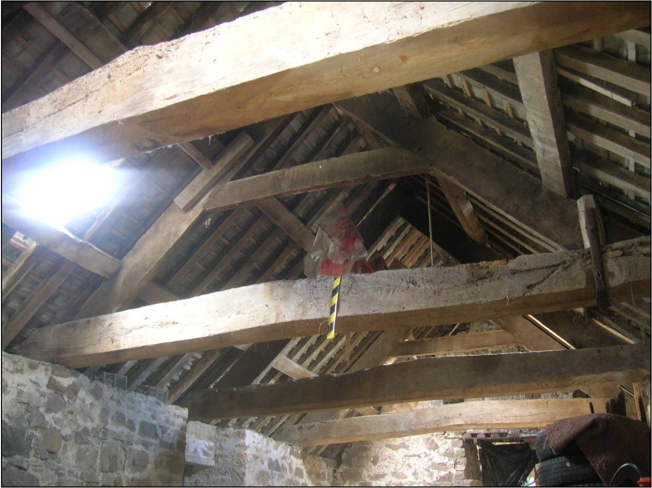
Figure 9: East range (north); truss 3 in foreground
