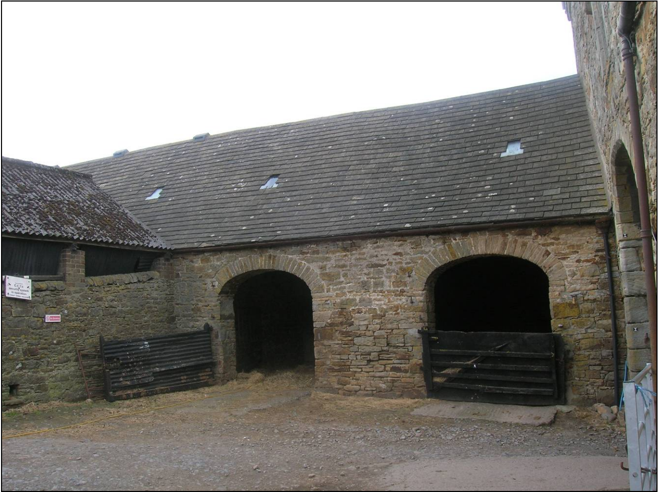
Figure 6: North range; taken from the south-east
