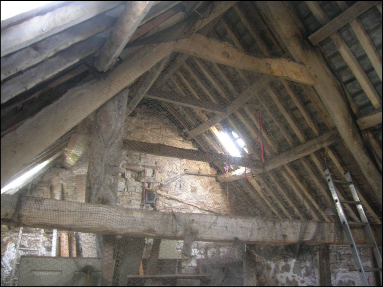
Figure 7: East range (south); truss 10
