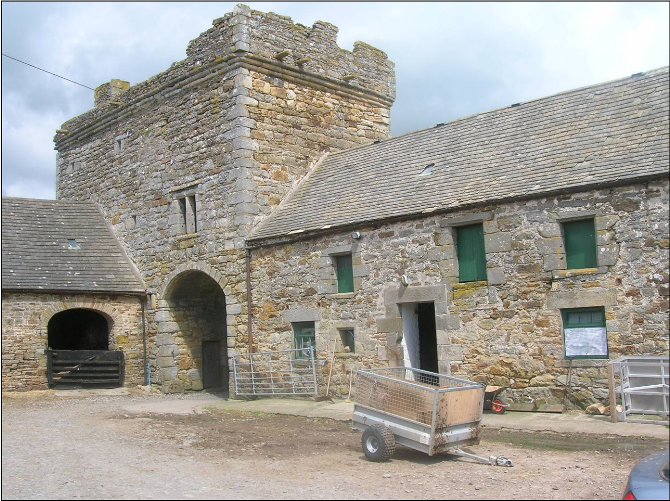
Figure 4: The gatehouse; taken from the south-west
