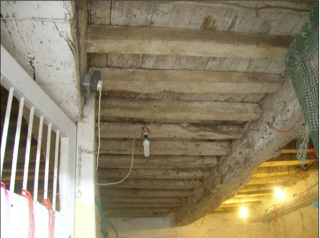
Figure 8: East range (south); ground-floor ceiling
