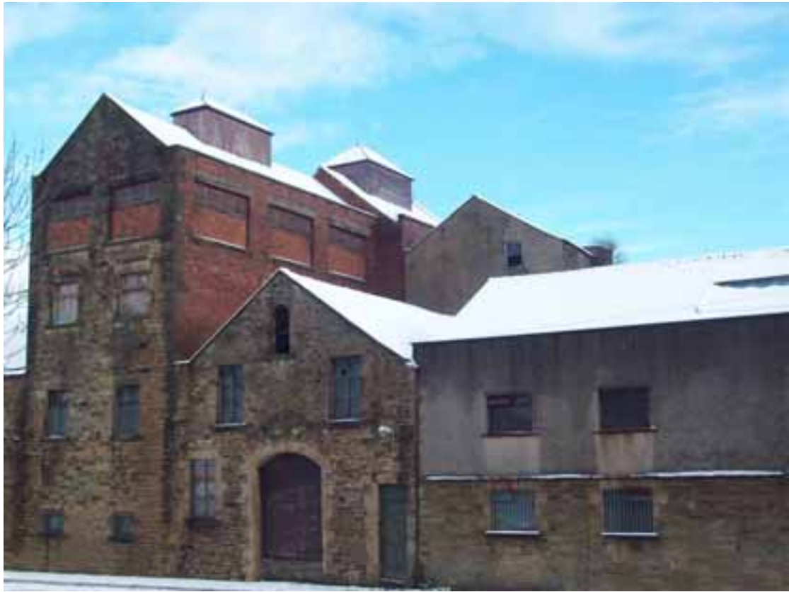
Figure 4: View of Mitchell's Brewery from Brewery Lane. To the left (north) rises the brick-built, partially stone-fronted, nineteenth-century building. In the middle, with its arched double door, is the stone-built north wing. To the rear of this rises the 'tower', the west window of which is just visible. To the right is the position of the eighteenth-century stables and the former courtyard, demolished and then enclosed in 1969 by the stone-block and rendered building
