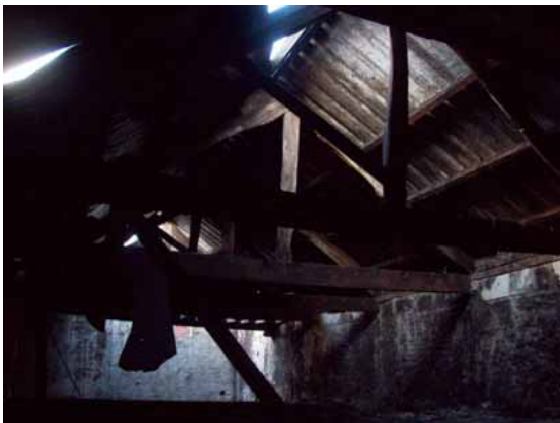
Figure 6: View of the roof trusses to the malthouse
