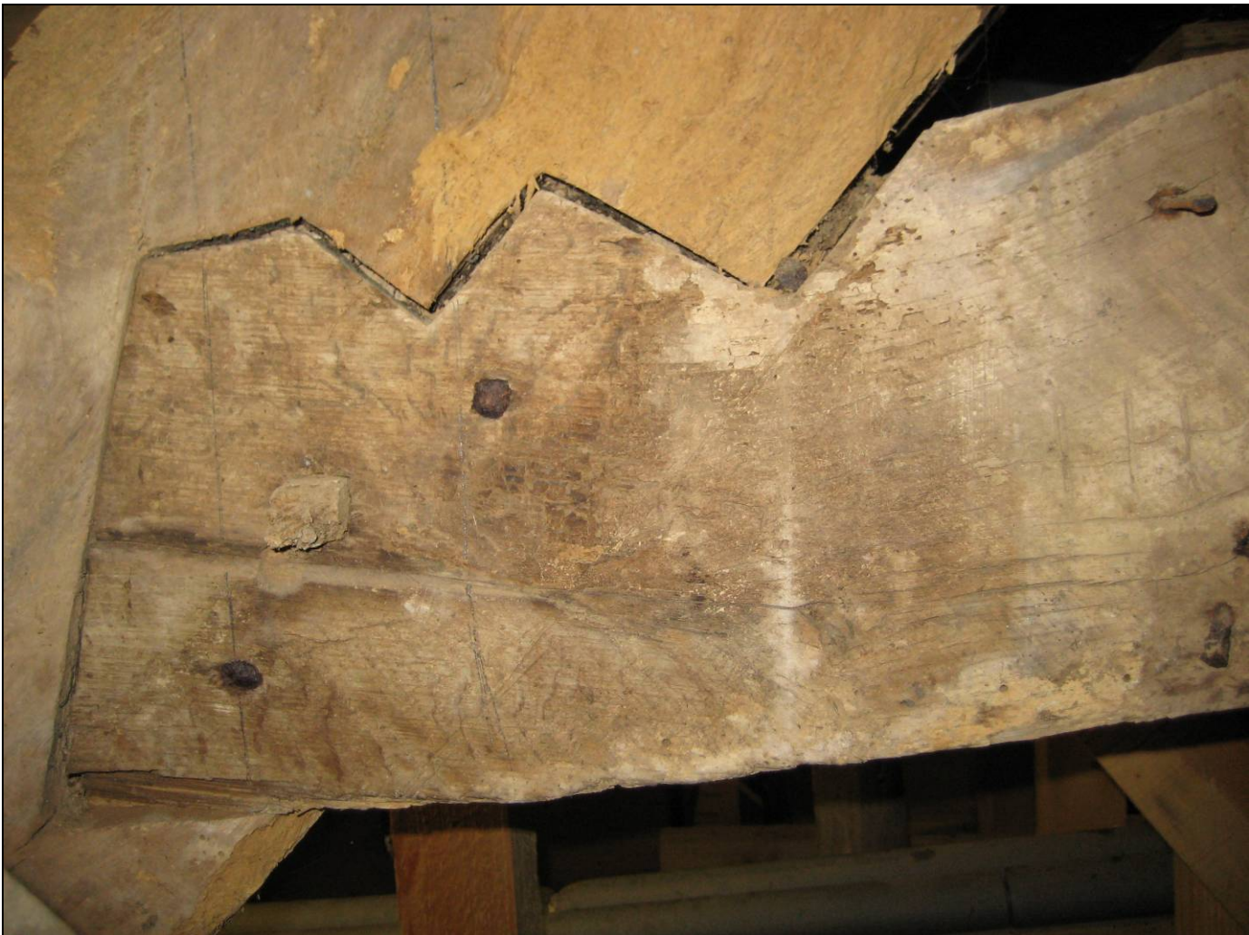
Figure 6: North-south range; truss 1, taken from the north-east
