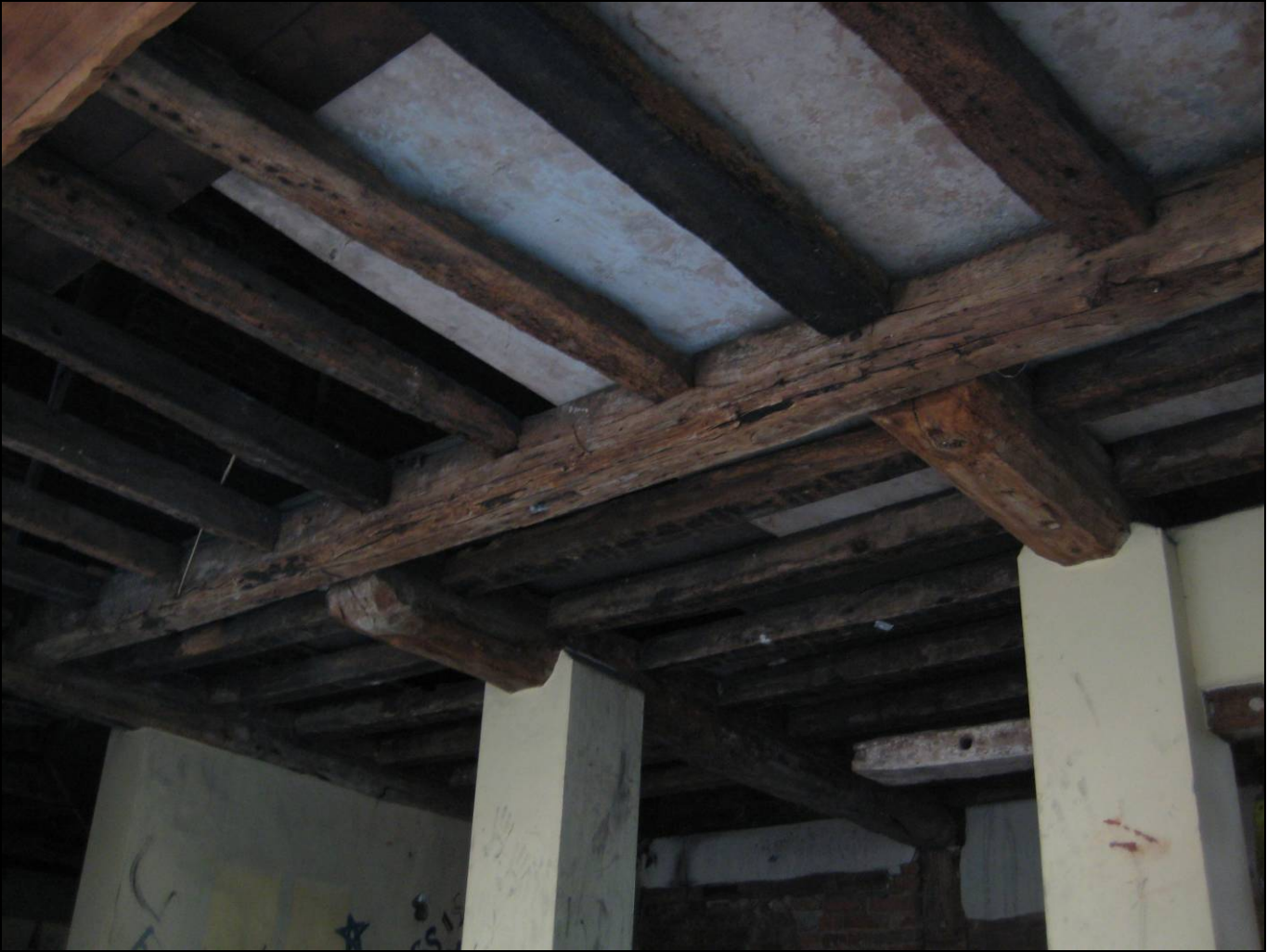
Figure 7: Ground-floor ceiling, northern wing, photograph taken from the north-west
