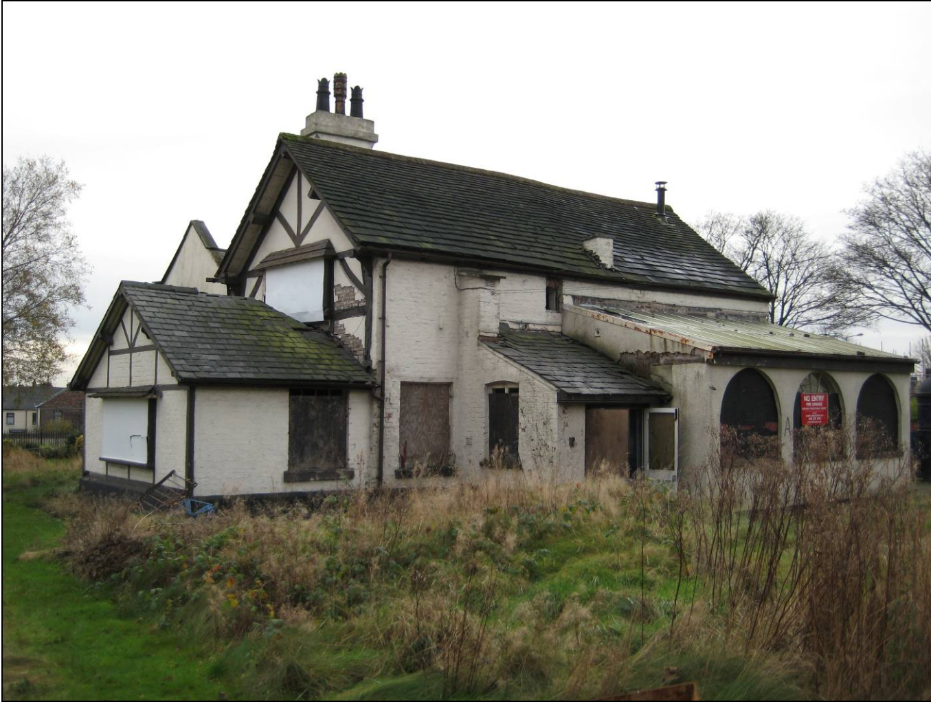
Figure 5: Two-storey northern range, photograph taken from the north-east
