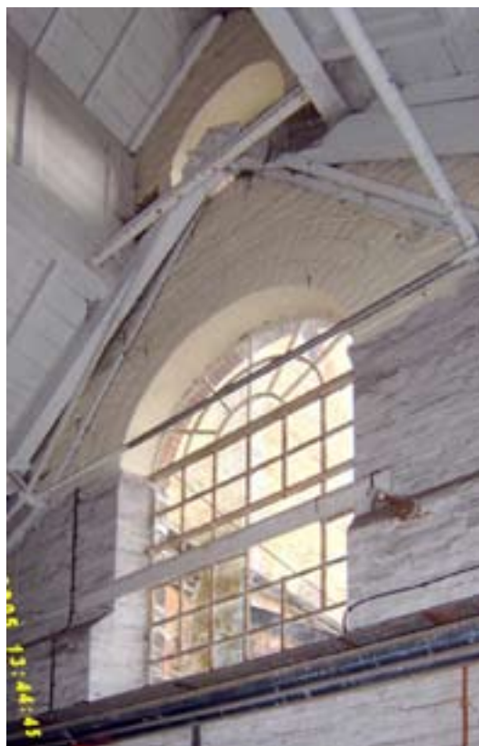
Figure 33: c.1854 element of Building 9, south internal elevation. Note the Polonceau trusses (photograph: Andrew Barber, B&DBC).
