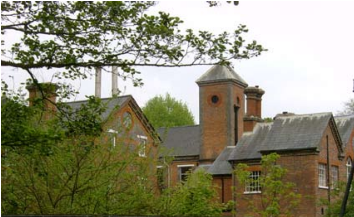
Figure 7: View of the site from the west (photograph: Andrew Barber, B&DBC).
