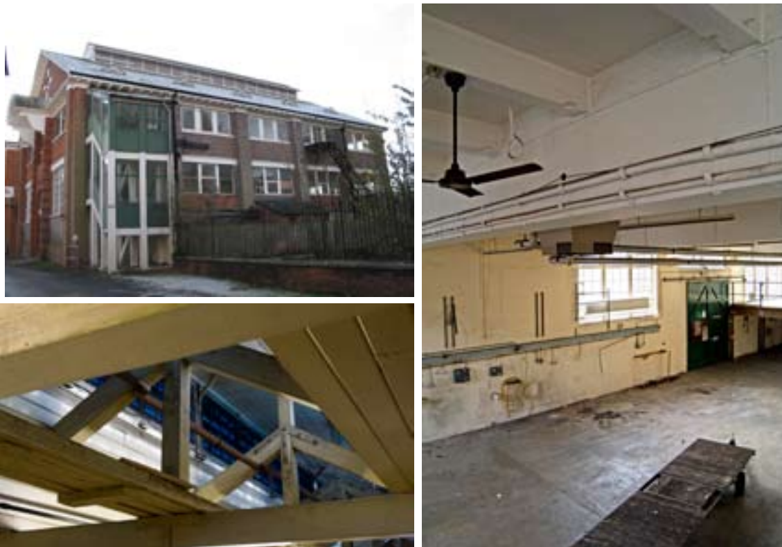
Figure 70 (top left): Building 14, north elevation (DP098894).
