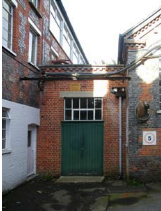
Figure 38: Building 10, south elevation (DP098886).
