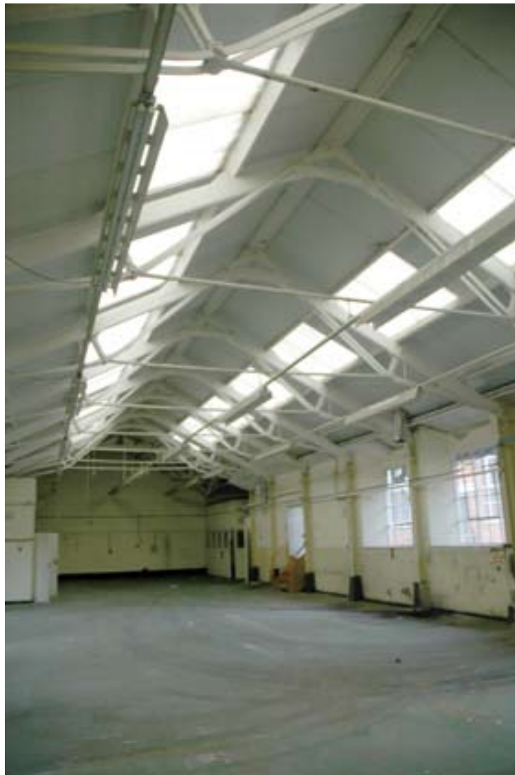
Figure 27: Building 5, (east-west wing), view to the west. (photograph: Jon Clarke, DP098883).
