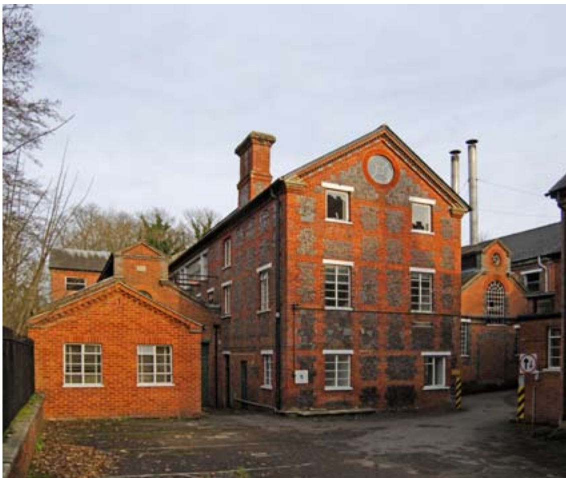
Figure 36: Building 11, south elevation (photograph: Derek Kendall; DP017461).
