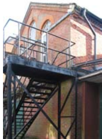
Figure 40: Building 4: north elevation (DP098887).
