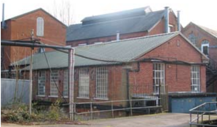
Figure 60: Building 27, north elevation (DP098893).
