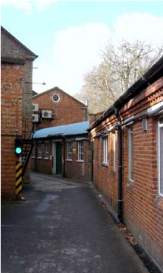
Figure 65: South elevation of Building 25 (to the right). In the background is Building 26 (photograph: Andrew Barber, B&DBC).
