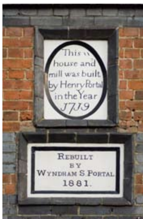
Figure 1: 1719 datestone reset on Building 1 (photograph: Derek Kendall; DP017538).
