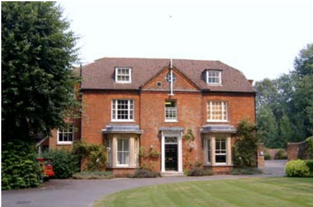
Figure 10: Mill House, west elevation (photograph: Andrew Barber, B&DBC).
