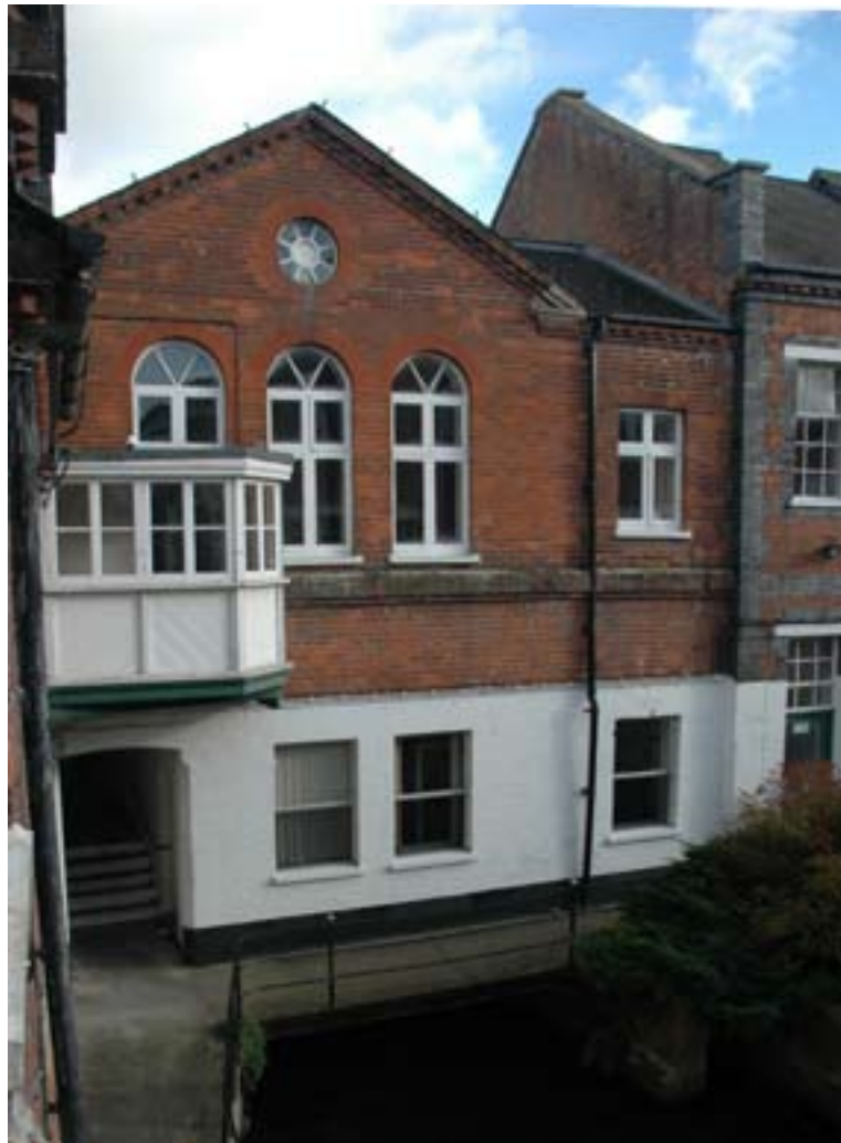
Figure 24: Building 5 (south wing): west elevation (photograph: Jon Clarke; DP098881).
