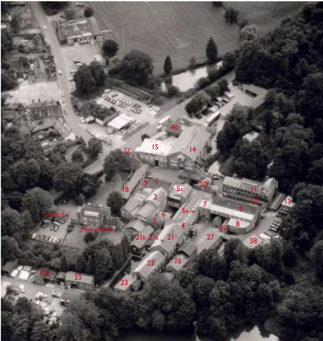
Figure 8: 1994 aerial photograph of Laverstoke Mill from the north east. The lake is visible at the bottom of the photograph. Buildings discussed in this report are numbered (NMR15154 ; © Crown copyright. NMR).
