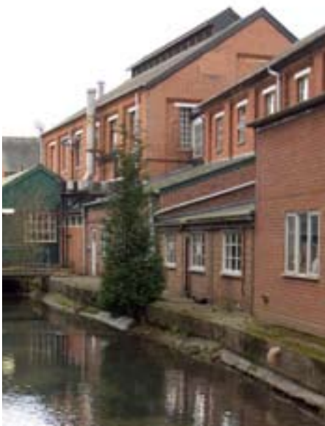
Figure 43: Building 21, south elevation (photograph: Derek Kendall; (DP017533)).
