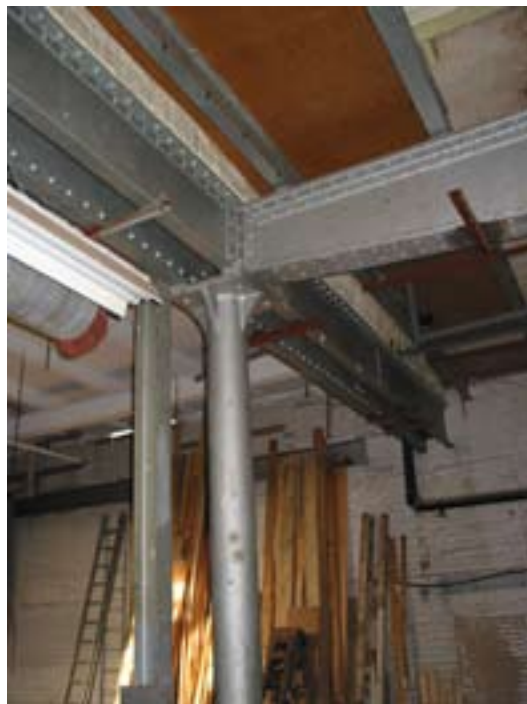
Figure 32 Building 9: fish-bellied beams (DP098884).
