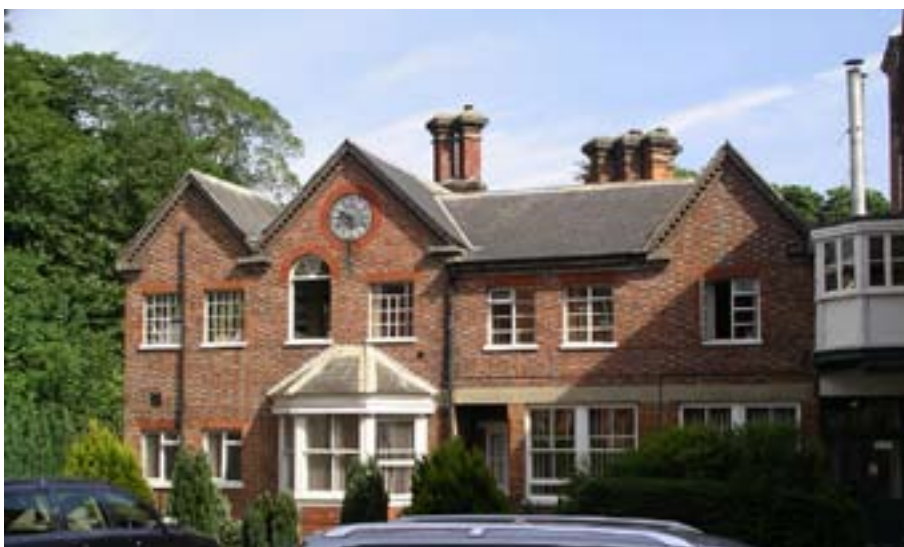
Figure 22: Mill offices, south elevation (photograph: Andrew Barber, B&DBC).
