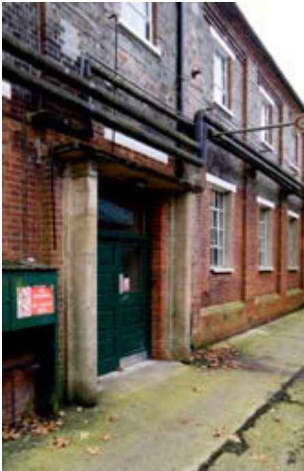
Figure 67: Building 22, north elevation (photograph: Derek Kendall; DP017525).
