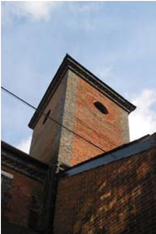
Figure 56: Building 7, watertower (DP098891).
