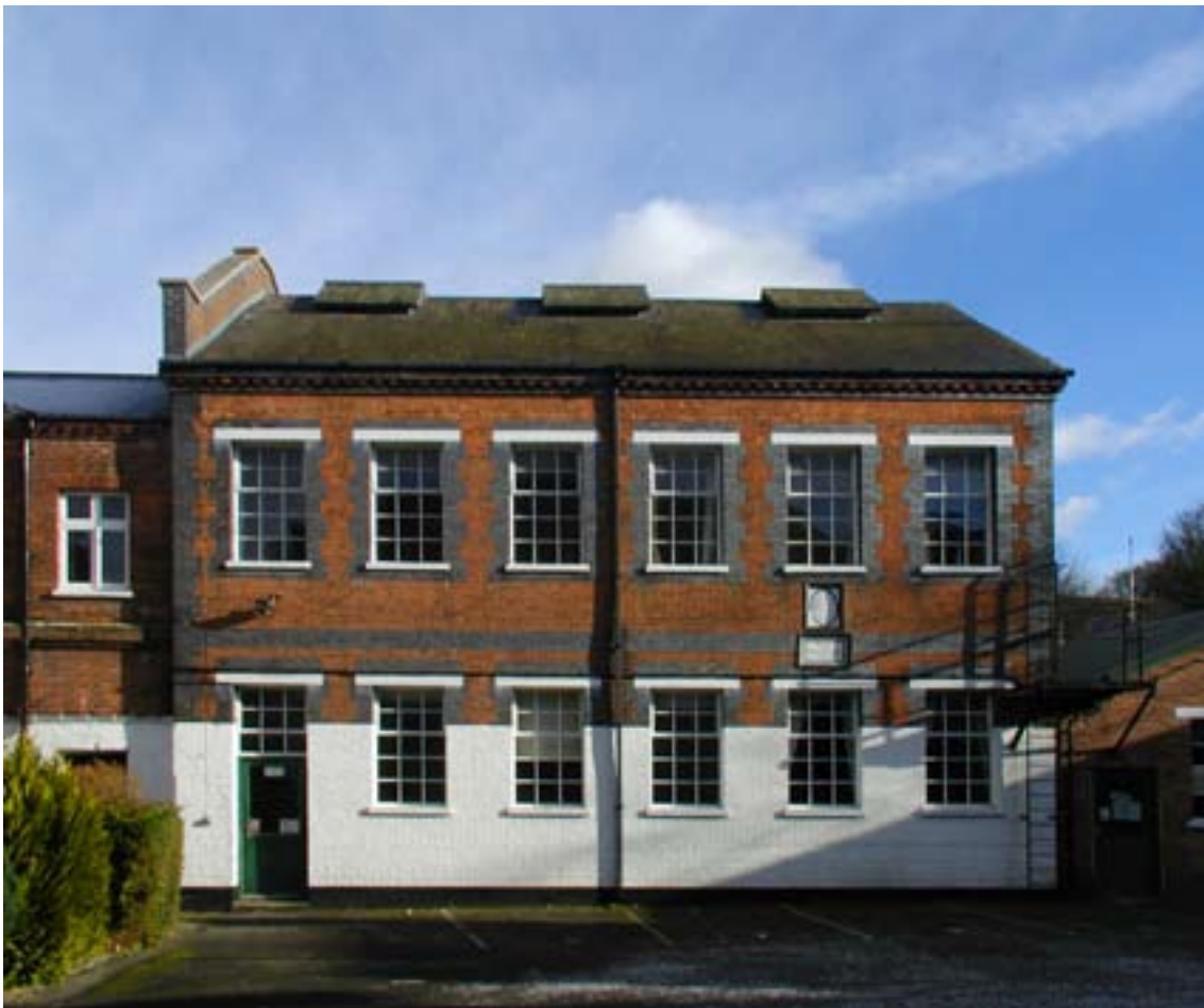
Figure 58: Building I, west elevation (DP098892).
