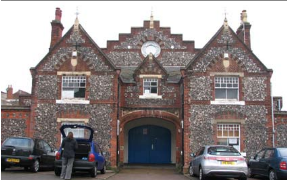
Figure 2. Southern facade of the drill hall.
