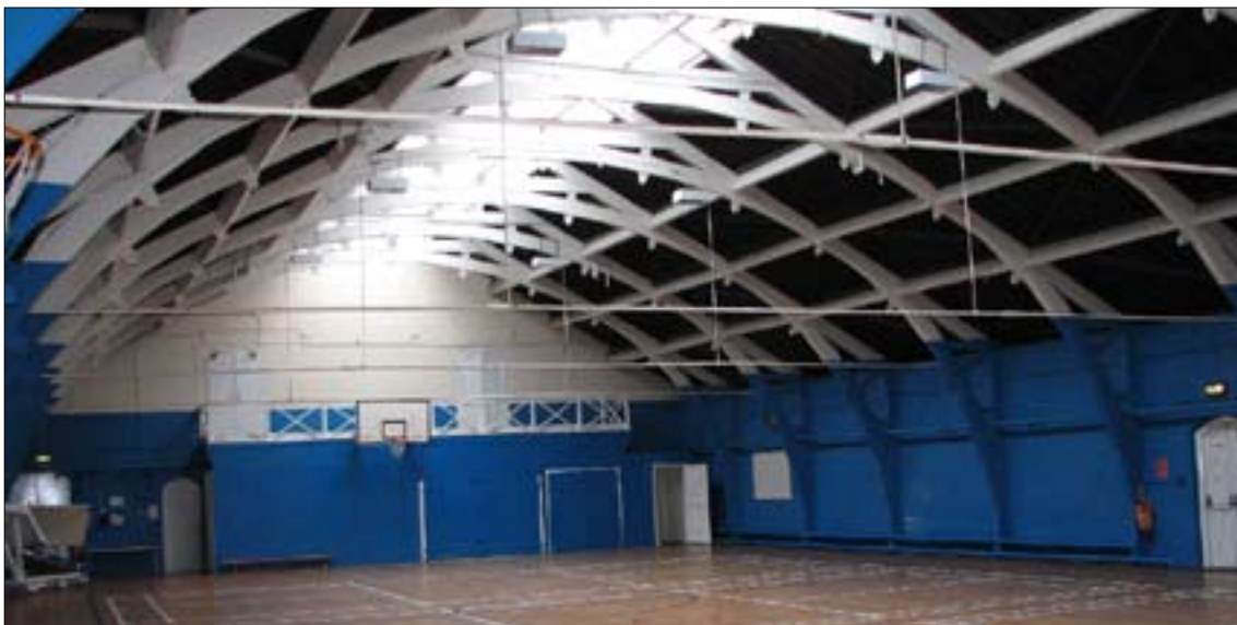
Figure 7. Interior of the drill hall looking north.
