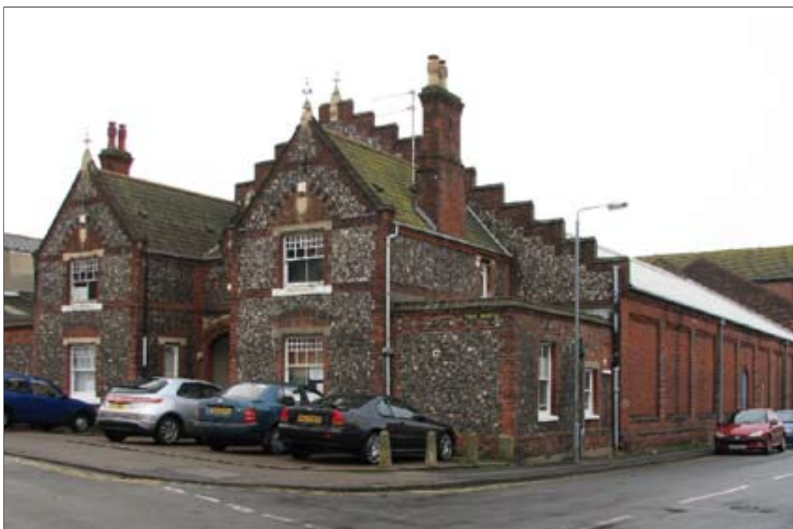
Figure 6. Front block with the drill hall behind.
