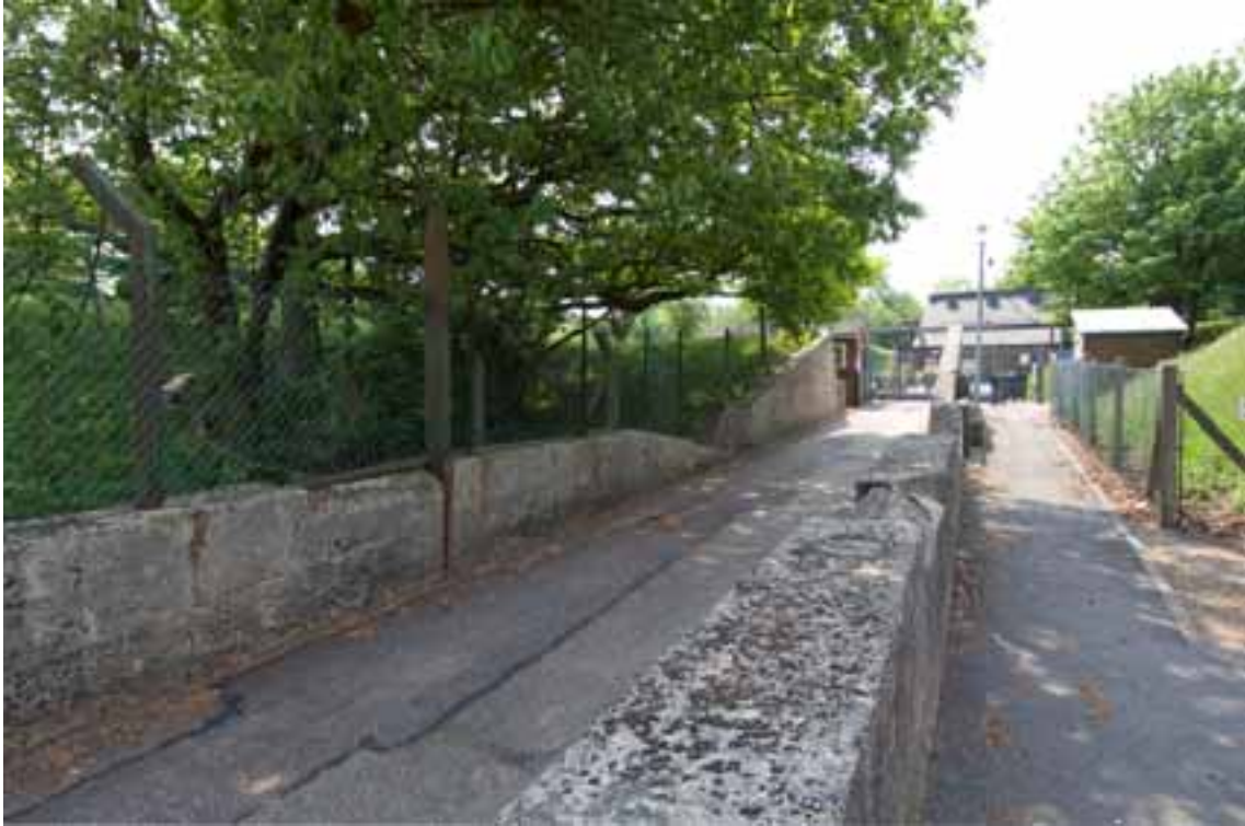
Figure 3: The main entrance to the Mobilisation Centre, to the left are traces of the fortress fencing and to the right part of the rampart has been removed to create a separate pedestrian entrance. © English Heritage DP060613
