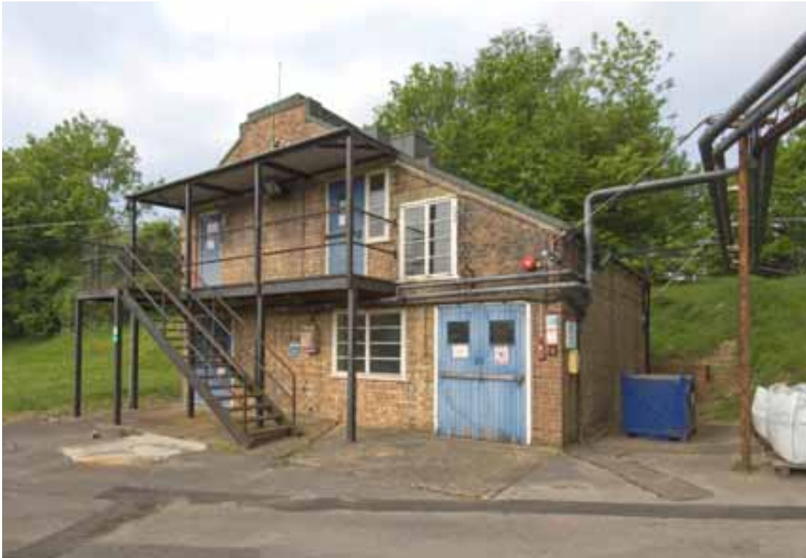
Figure 4: Experimental filling shed F11 erected in 1938 for filling cordite rocket motors. © English Heritage DP060536
