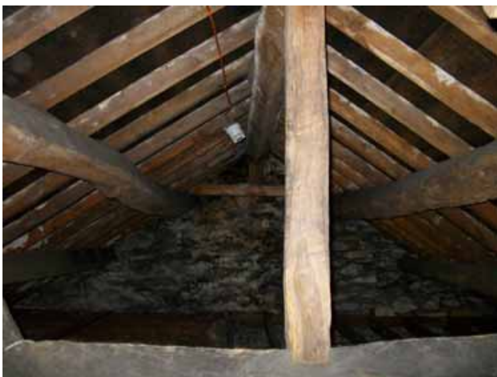
Figure 3a/b: Front (top) and rear (bottom) roofs of the house range
