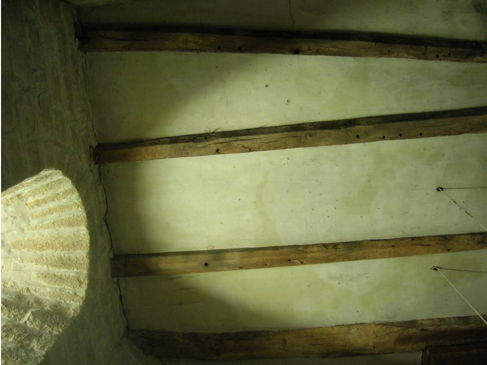
Figure 9: The floor of the 'winding chamber'
