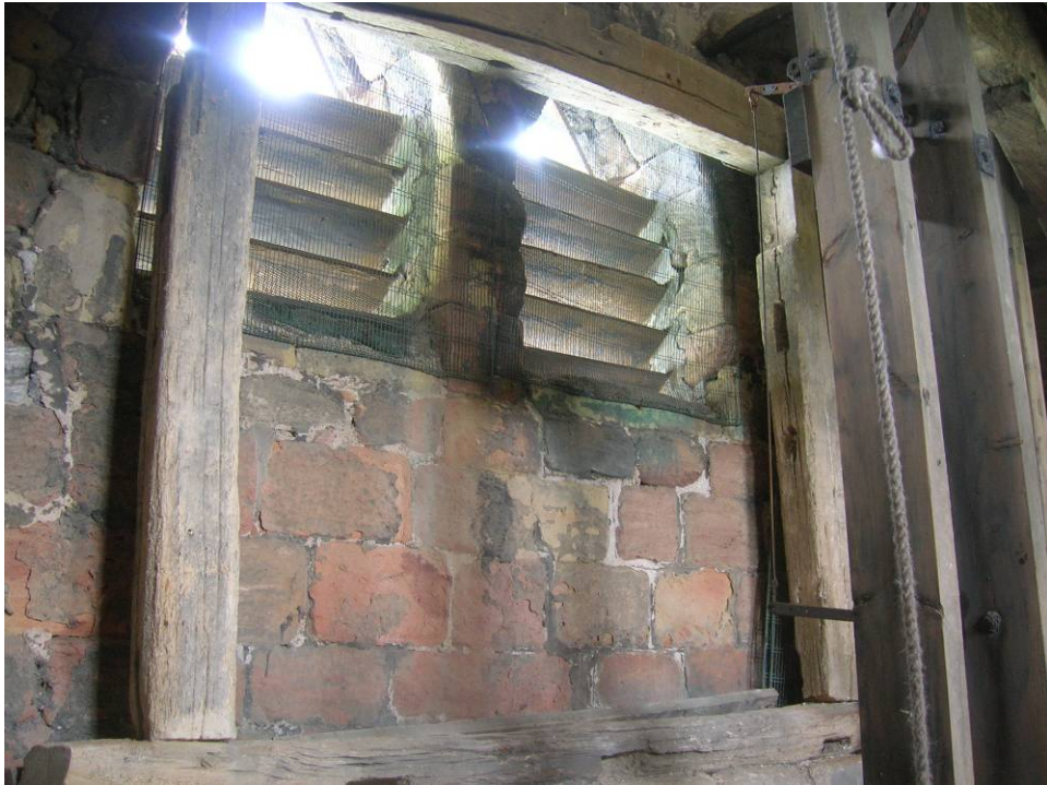
Figure 7: Truss 4, the 'bell-cote' in the bell chamber
