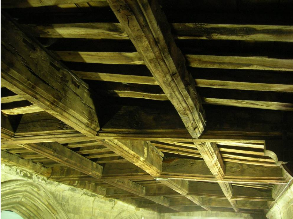
Figure 3: View of the lower or inner roof to the south aisle
