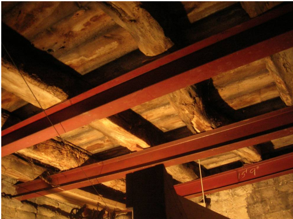
Figure 8: The ceiling beams of the 'winding chamber'
