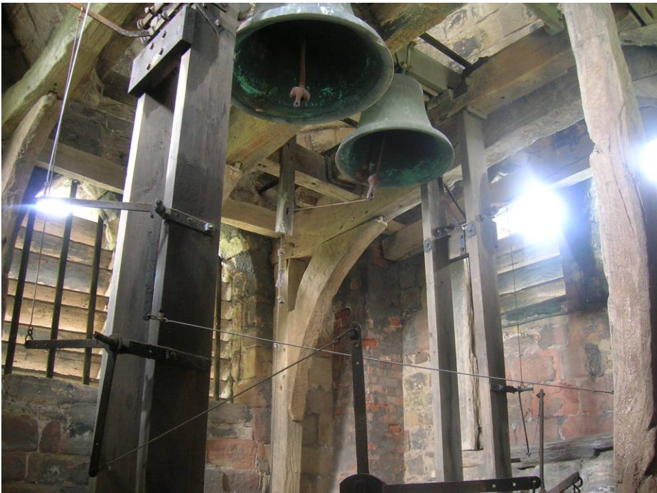
Figure 6: View of the bell frame
