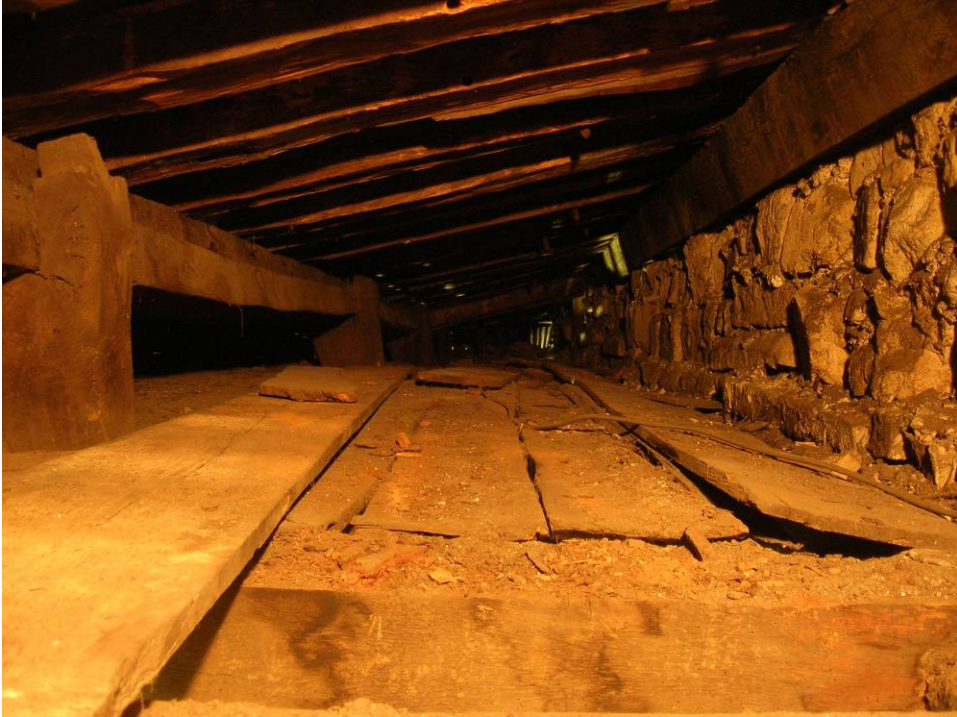
Figure 5: View of the upper or outer roof looking east to west
