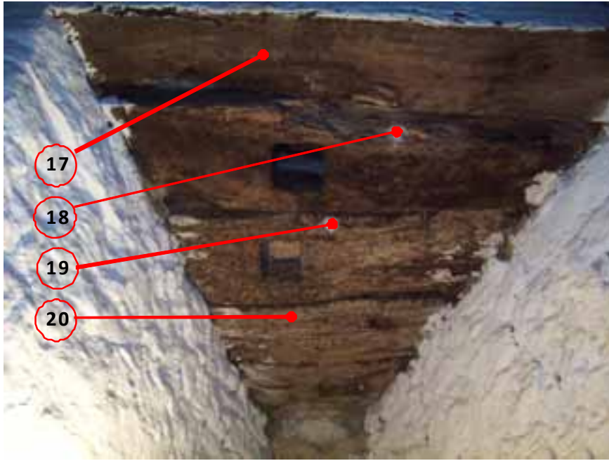
Figure 10: Photograph of the west window lintels to show sampled timbers
