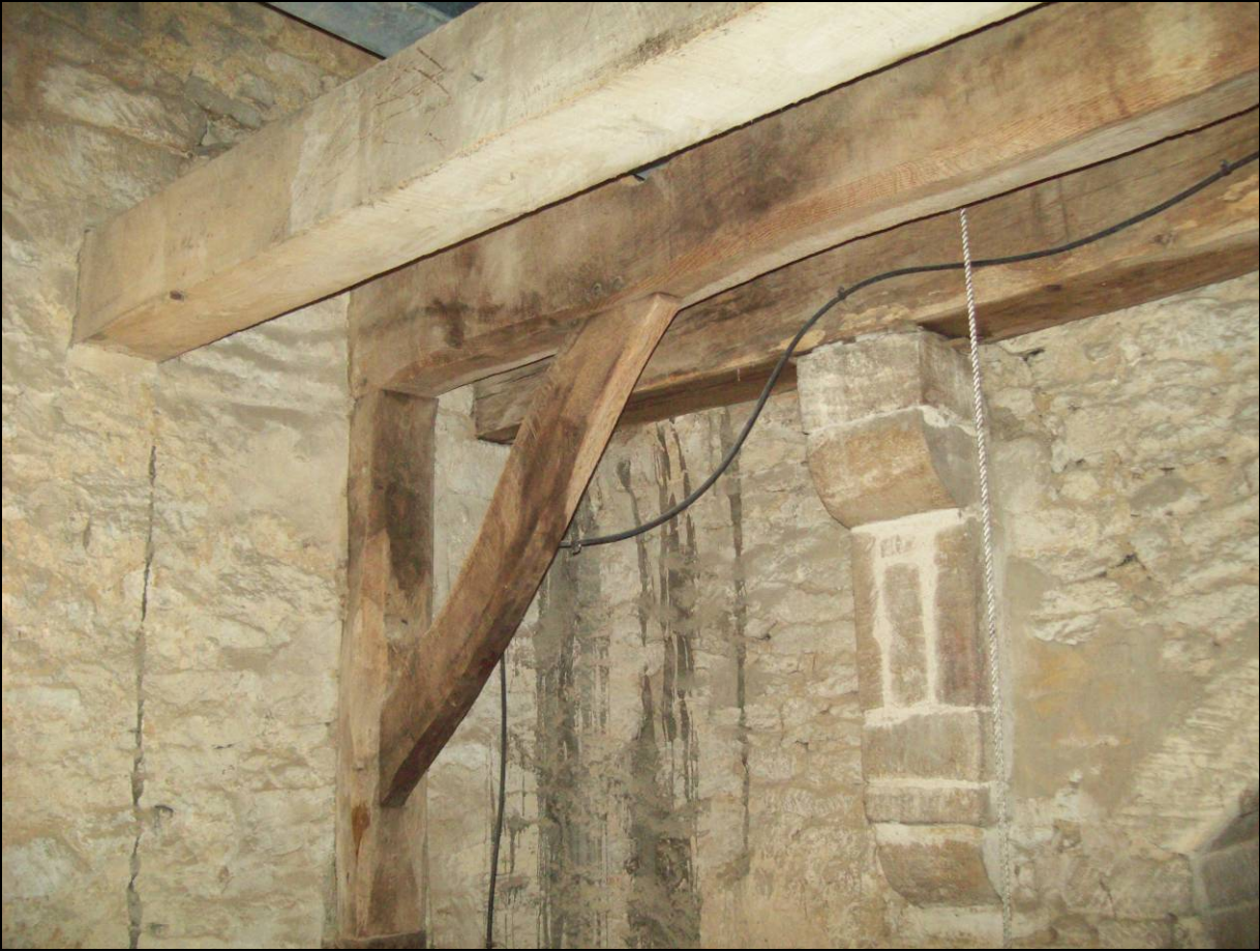
Figure 5: Lower in-situ timbers (east truss, north side)
