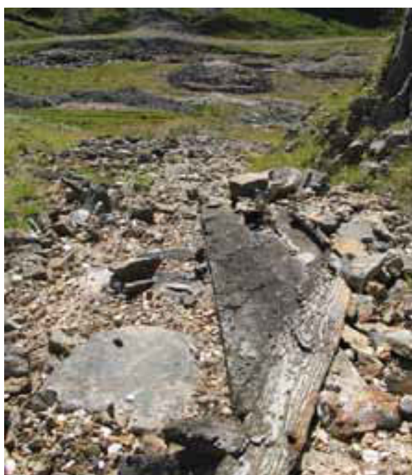
Figure 61 View down the route of chute 295; surviving timbers can be seen in the foreground. The remains of mill 29 can be seen at the end of the chute.
