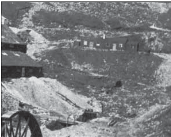
Figure 91 Extract from late 19th century photograph showing the possible mine shop (40) situated on spoil heap 41. Crushing mill 29 is at the left of the photograph and culvert 35 can be seen below the building.
