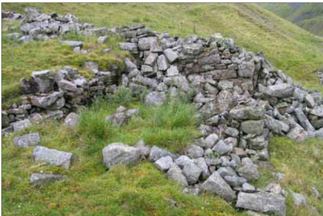
Figure 81 Remains of structure 363, possibly the early smithy close to High Shop. The collapsed supporting buttress can be seen at the right-hand side of the photograph.
