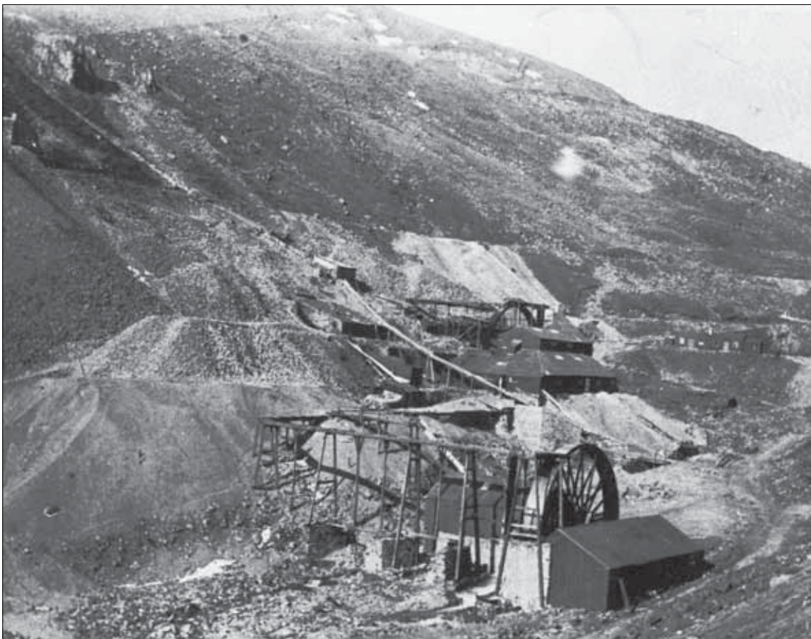
Figure 34 Late 19th-century photograph of the processing area at the confluence of Scordale Beck and Great Augill. Mill 27 is in the foreground. The timber launders visible in the photograph transported water around the site, supplying both overshot waterwheels.
