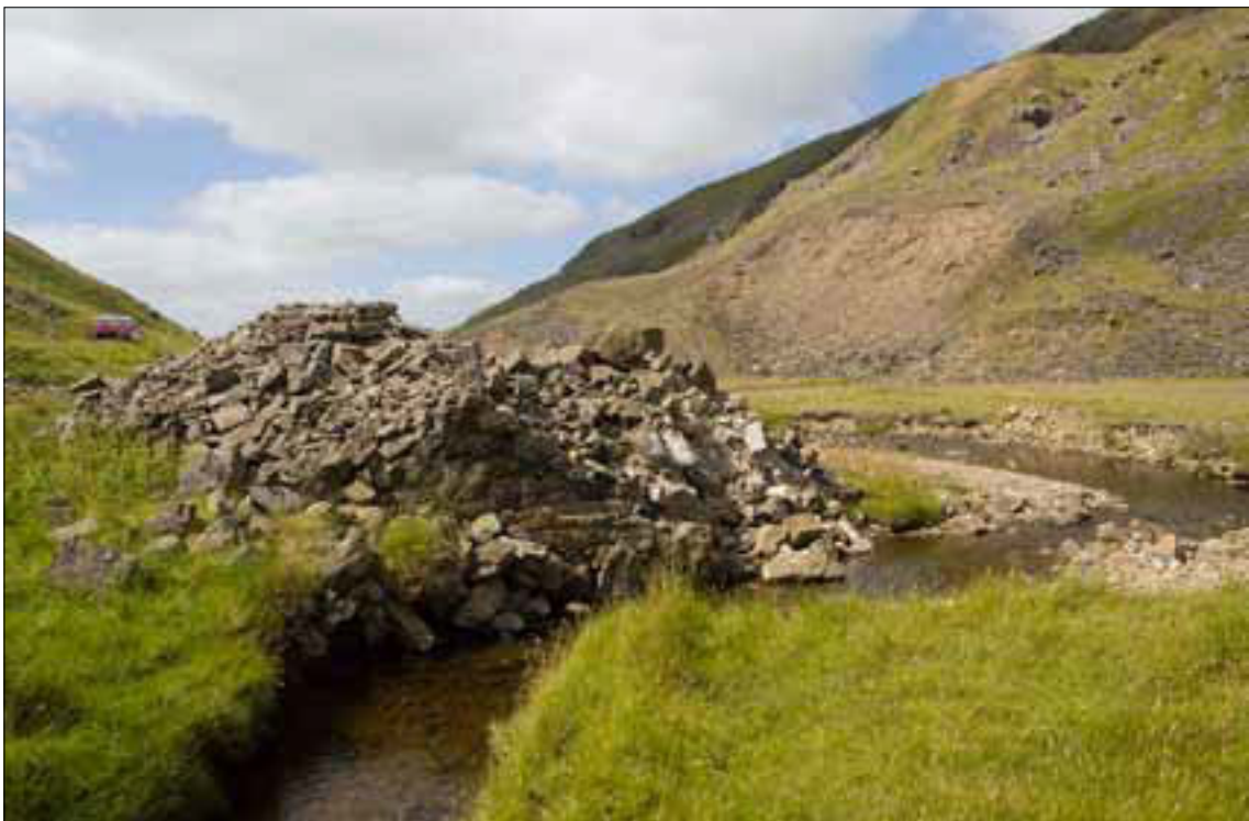
Figure 69 The tumbledown remains of mill 81. The mill race (871) approaching the structure can be seen in the foreground.
