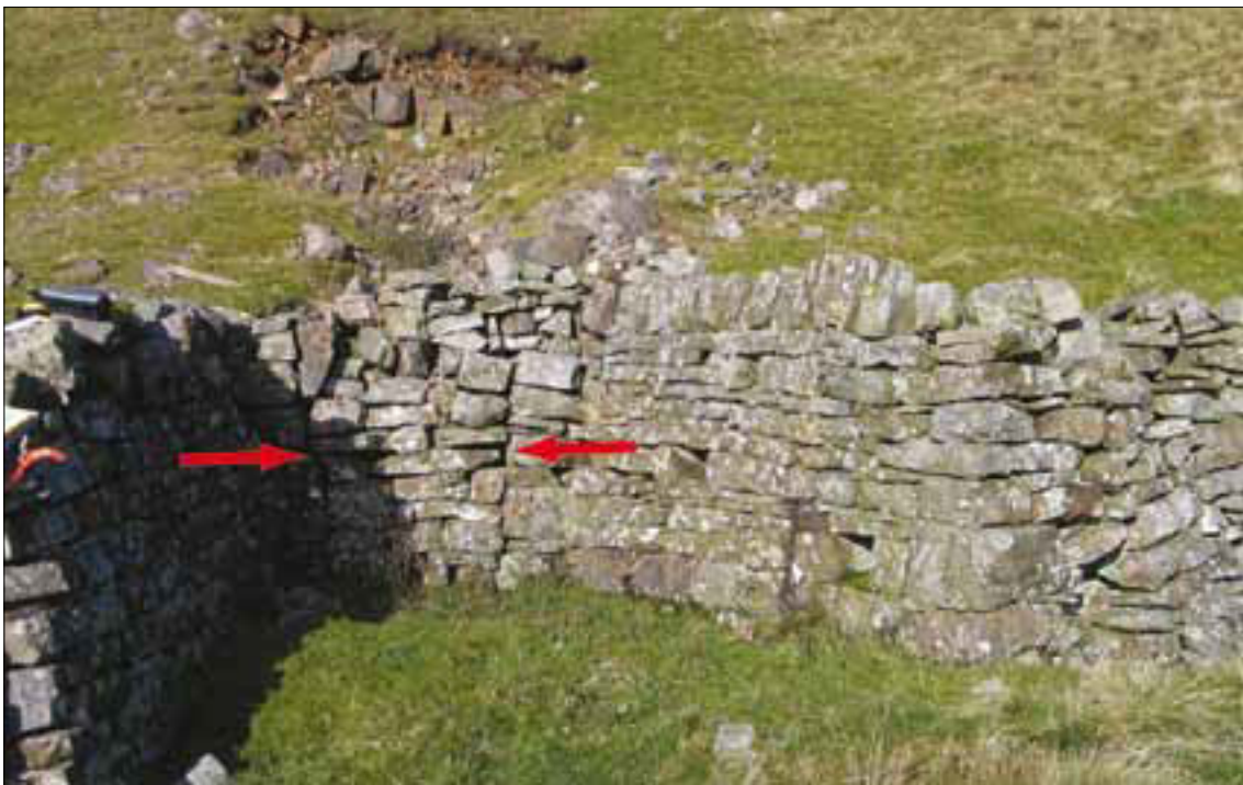
Figure 49 Entrance to level 540. The straight joins in the drystone wall (indicated by the arrows) show where the gap allowing access to the level has subsequently been blocked.
