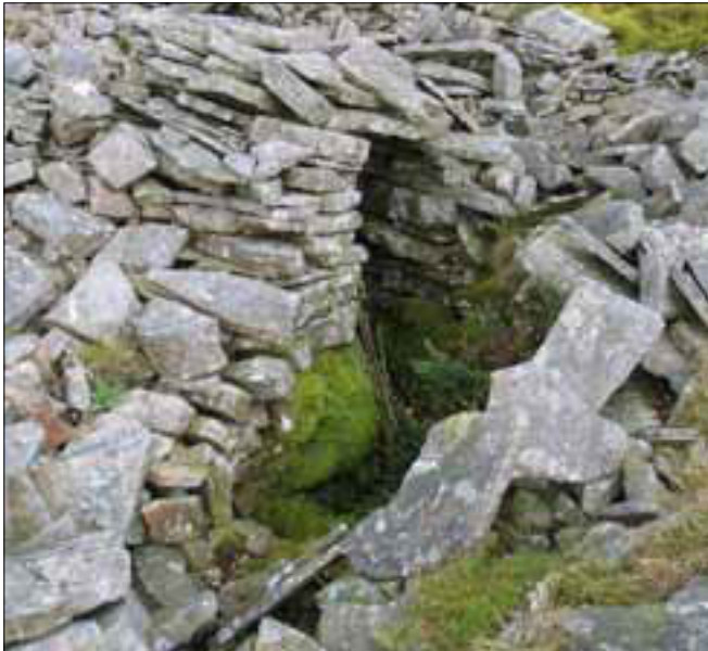
Figure 38 Entrance to shaft capped with drystone beehive-like structure. It is not possible to be certain of the date of this feature, but it is likely to be relatively early.
