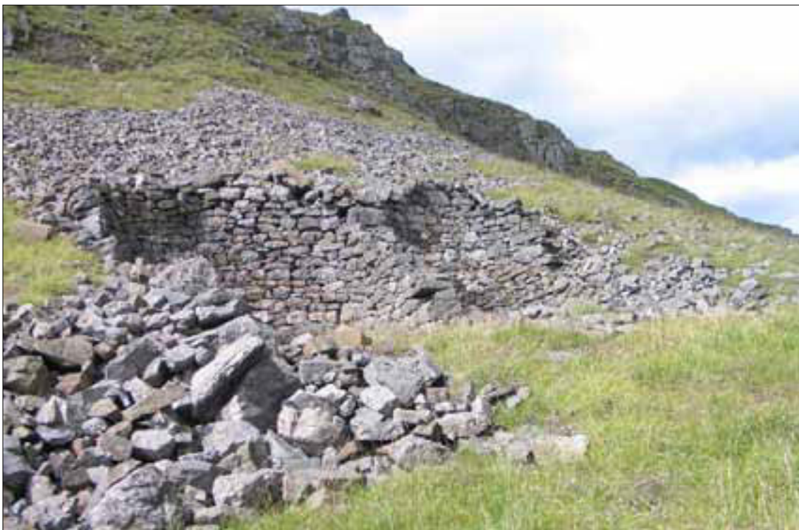
Figure 55 A well-preserved pair of ore bins (380) on the lower slopes to the north-east of Mason Holes
