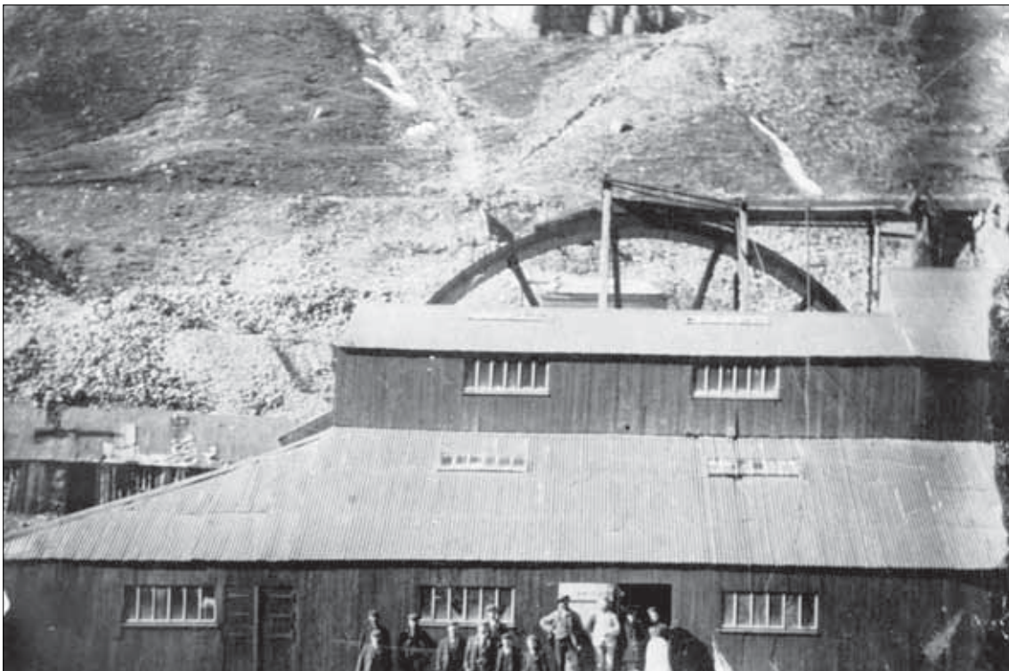
Figure 33 Late 19th-century photograph of the principal crushing mill (feature 29), illustrating the overshot waterwheel powering the mill.
