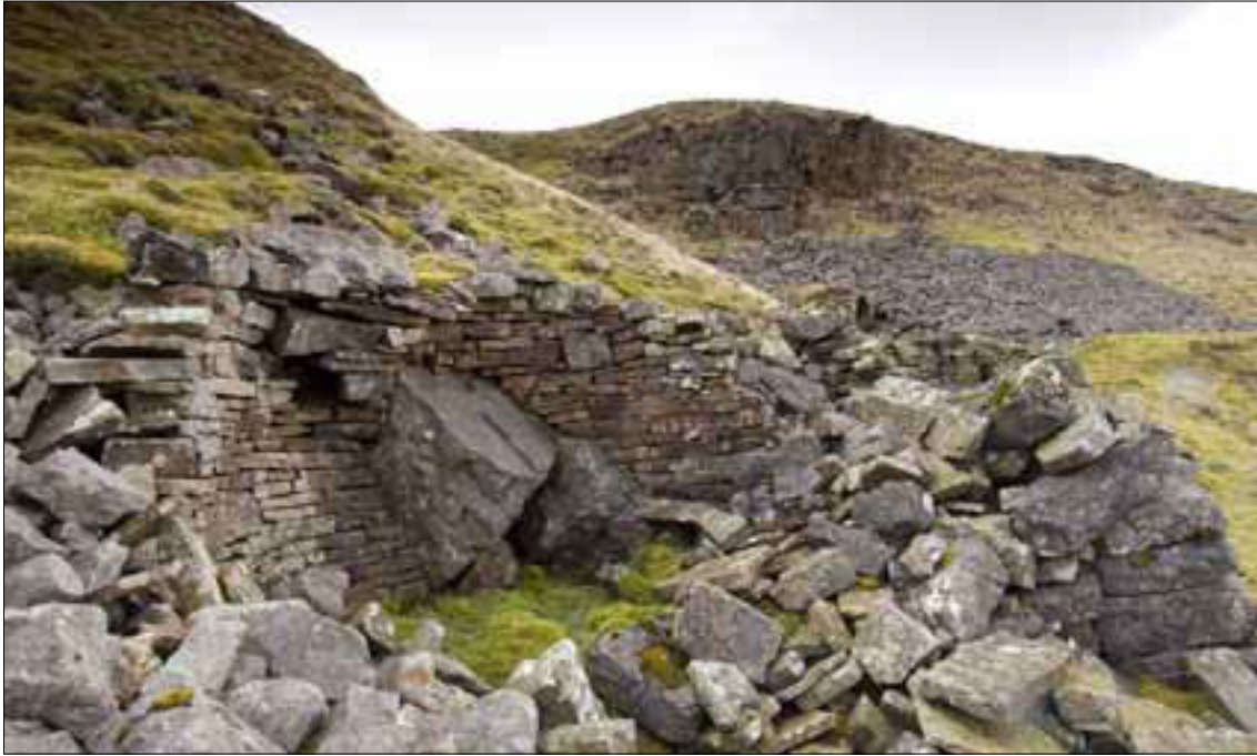
Figure 54 The series of ore bins to the north of Jacques Level. The ore bin with the large boulder incorporated into its rear wall can be seen in the foreground.
