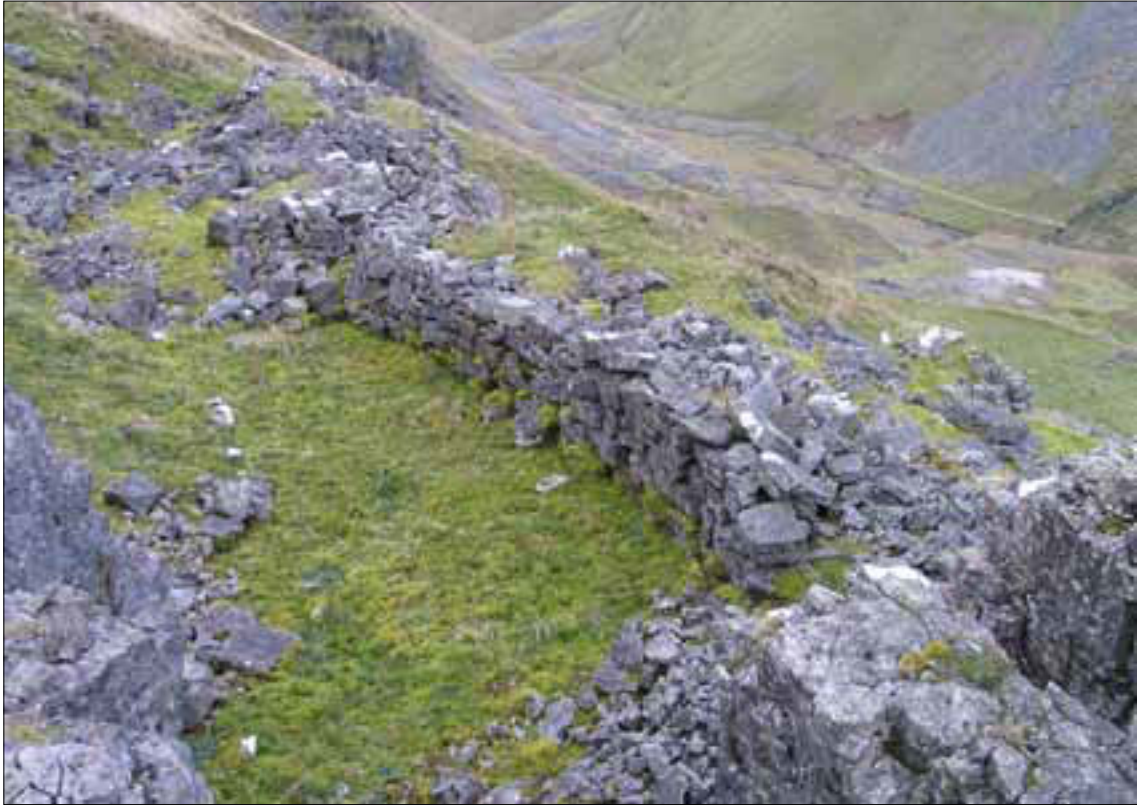
Figure 42 Revetment wall (549) lining and revetting the downslope side of hush channel 560
