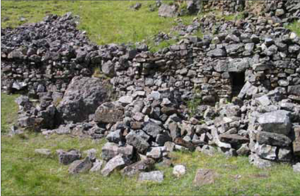
Figure 85 Remains of a shelter (624), built into the pre-existing field wall. The aperture with a lintel, at the right-hand side of the photograph, is the fireplace.
