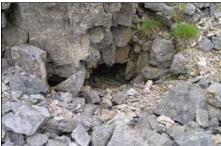
Figure 47 The entrance to Hardside Low Level (49), deliberately blocked
