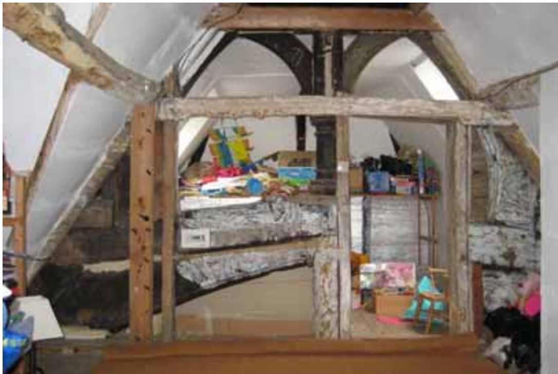
Figure 6: Truss B viewed looking east
