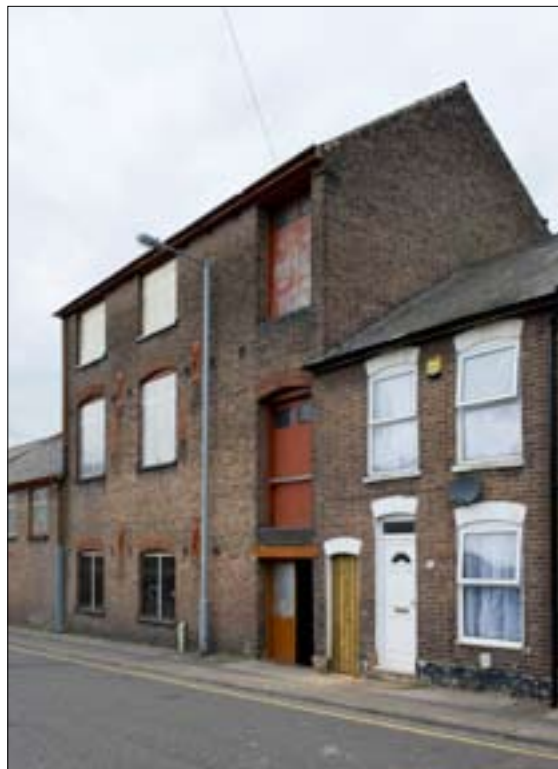
Figure 26 Block E and 113 North Street. © English Heritage NMR DPI10764
