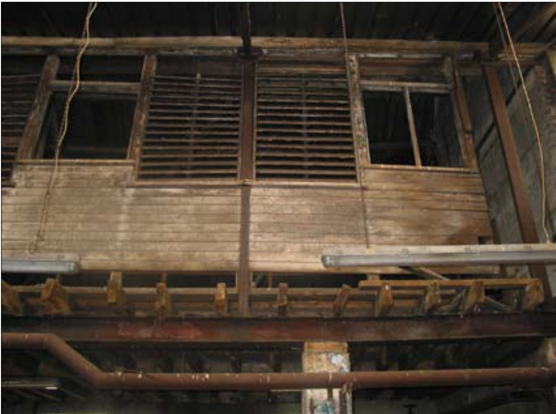
Figure 38 Wooden louvres on the southern elevation of room 50.
