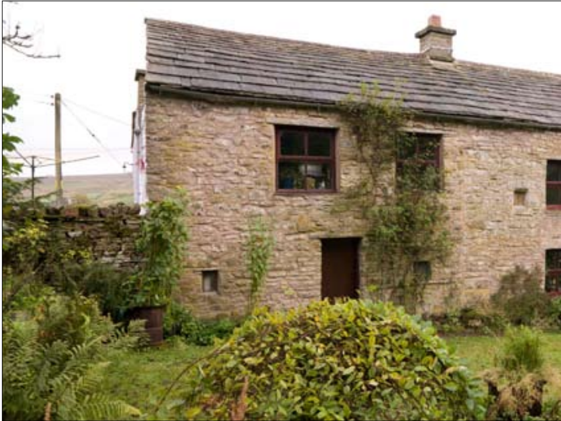
Fig. 16: The 2-storey western addition to the bastle, entirely refenestrated in the 19th century. [DP072081]
