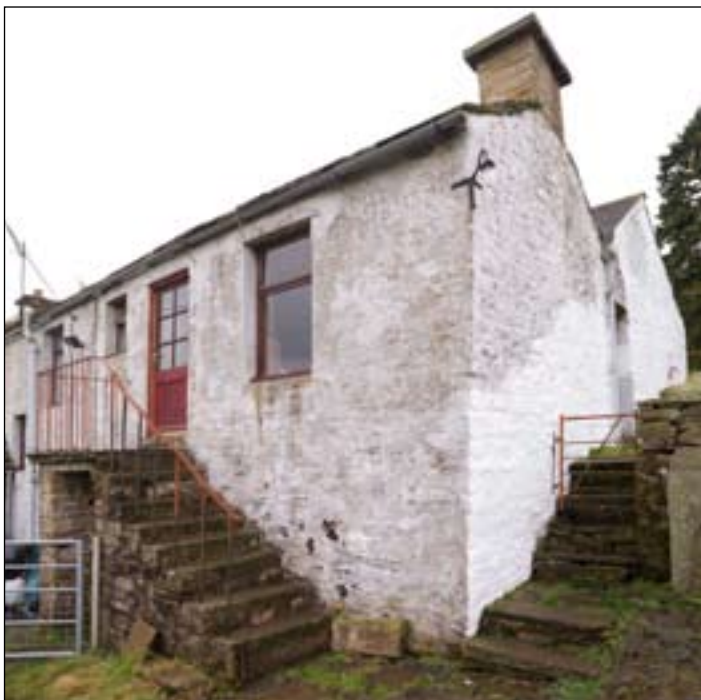
Fig. 19: The western half of the two-storeyed northern addition, showing the external stair to the 1st-floor dwelling. [DP072087]
