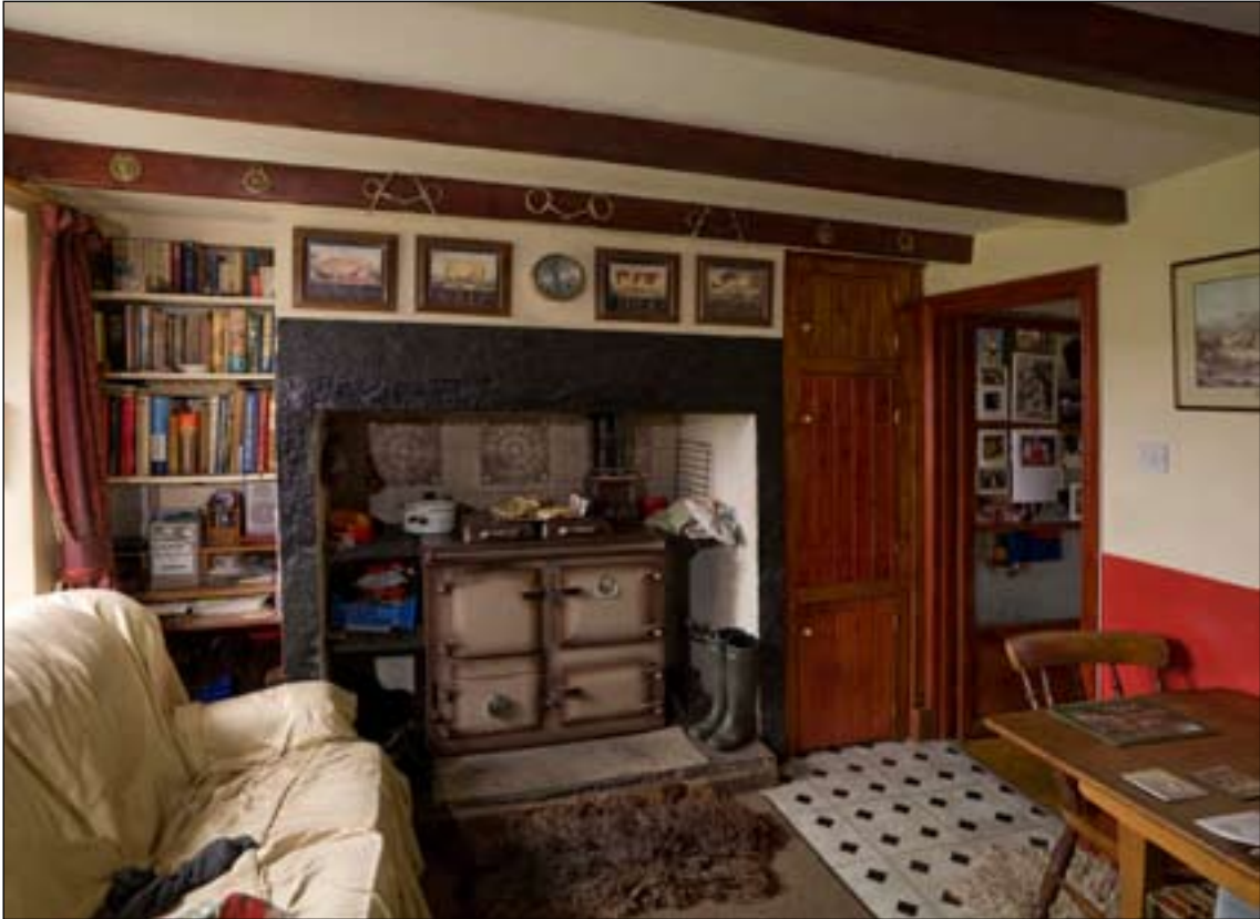
Fig. 18 The early 19th-century back kitchen with its monolithic-jambed fireplace, located at the eastern end of the northern addition. The addition now communicates with both rooms in the ground floor of the bastle, although the date at which they were connected is unknown. [DP072092]
