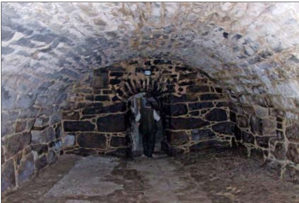
Fig. 5: The stone barrel-vaulted ground-floor byre of the bastle at The Raw, Hepple, Northumberland, showing the central, gable-entry byre doorway. [DPI35347]
