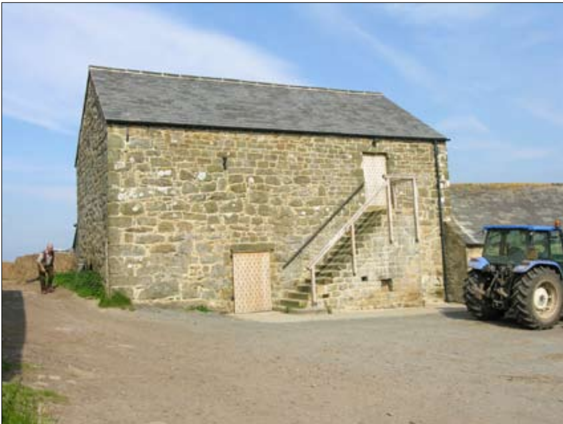
Fig. 4: Bastle at The Raw, Hepple, Northumberland, demonstrating the basic rectangular form of the bastle, with its later external stair to the first-floor door and the limited fenestration of both storeys. The upper storey has been largely rebuilt. [DPI35346]
