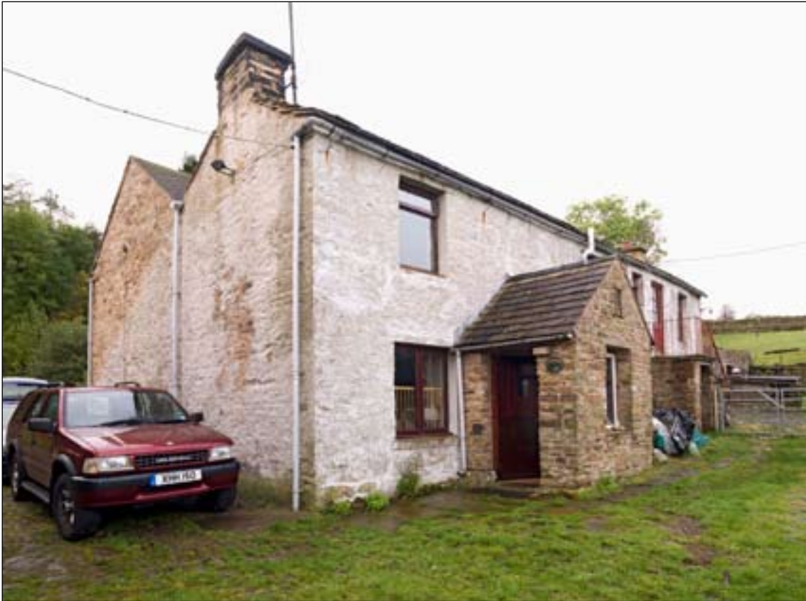
Fig. 17: The two-storeyed northern extension, providing additional accommodation for the bastle and creating a new, one-room first-floor dwelling. [DP072085]
