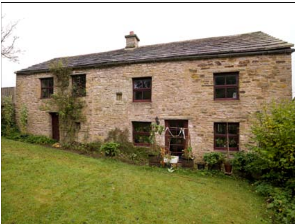
Fig. 6: The south elevation of Nettle Hall, showing the straight joint following a line from the left of the present chimney stack. The bastle core of the house lies to the east of the masonry break, with a small fire window evident on the first floor. To the west is the first addition to the farmstead: this linear addition is probably an agricultural range of the 18th century. [DP072080].
