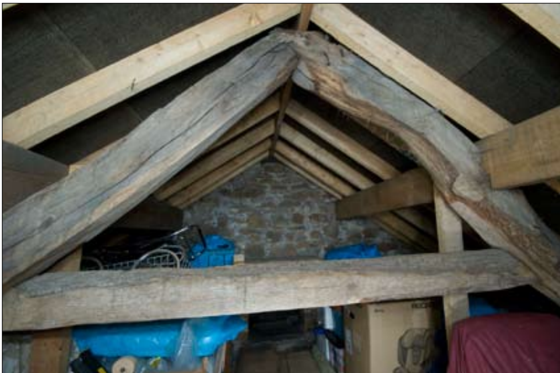
Fig. 13: The surviving truss, viewed towards the east, with its wavy principal rafters and replaced collar. [DP072102]
