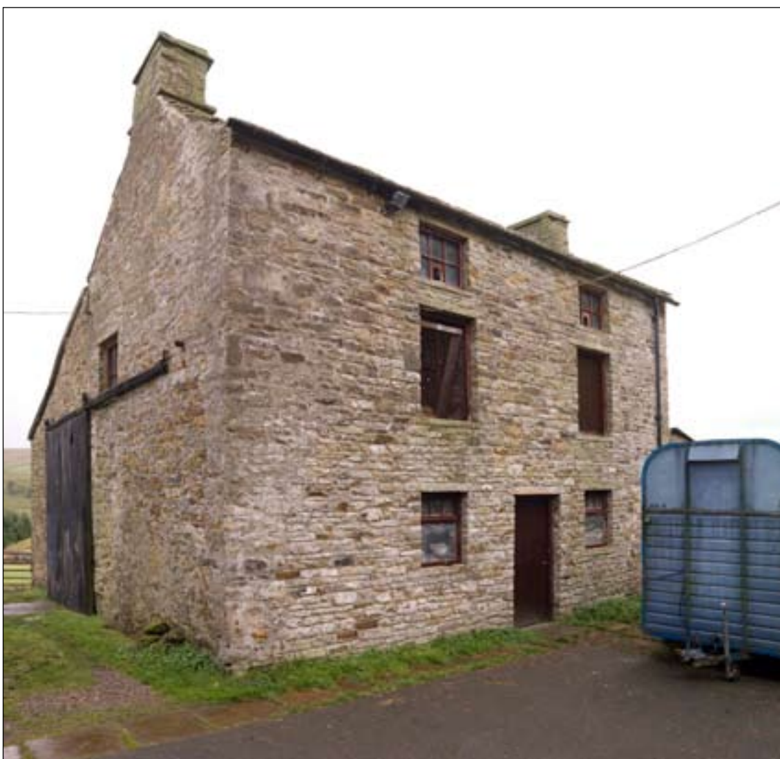
Fig. 21: The mineshop from the south-west. [DP072083]
