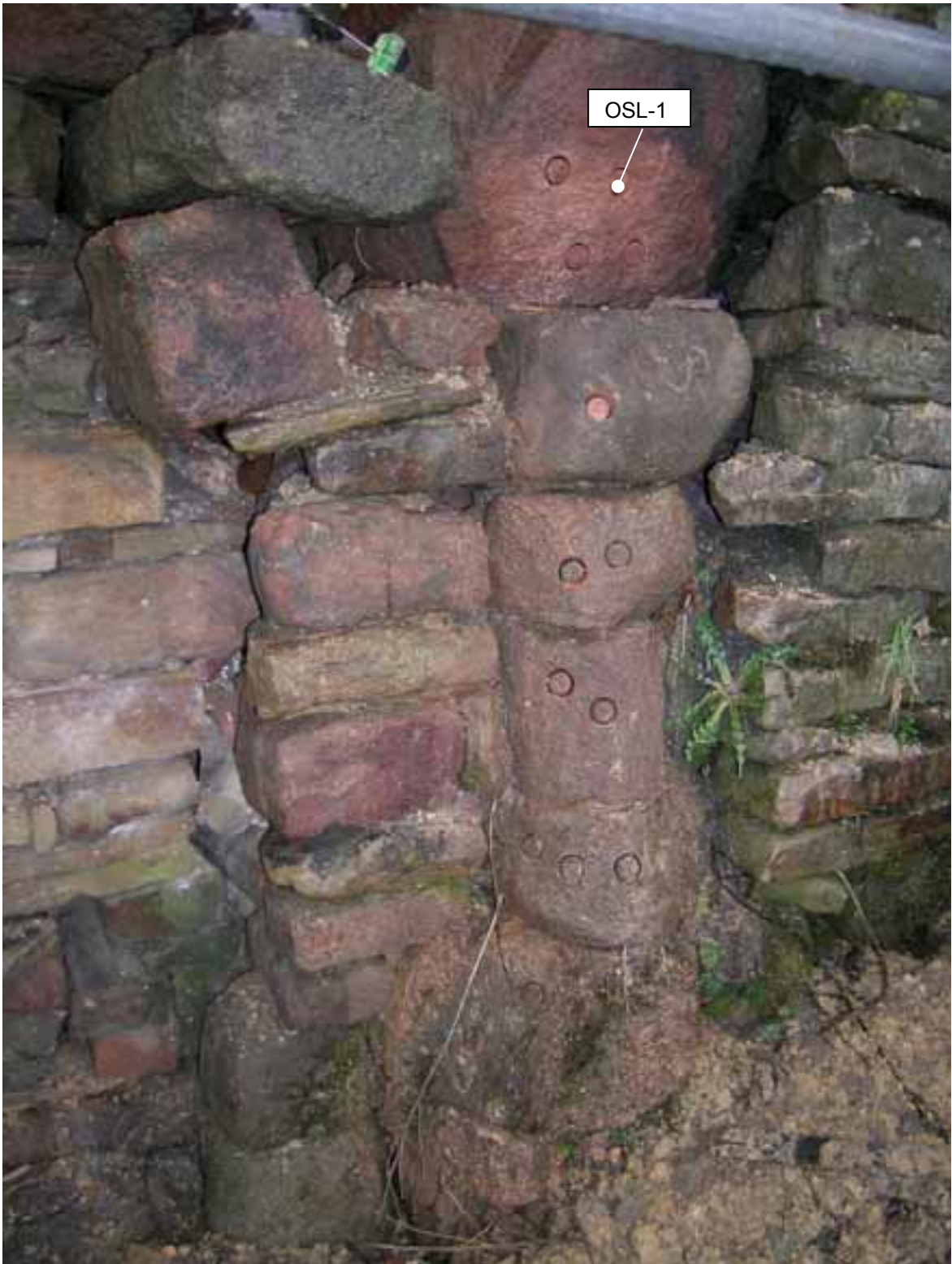
Figure 2a. Close-up of external wall containing the annealing furnace flues showing the locations of cores within feature 'BSA' obtained for archaeomagnetic dating, and including sample OSL -1. Samples OSL-3 and -4, located in an adjacent section of the wall, are shown in Fig 3 (reproduced from Karloukovski and Hounslow 2007)
