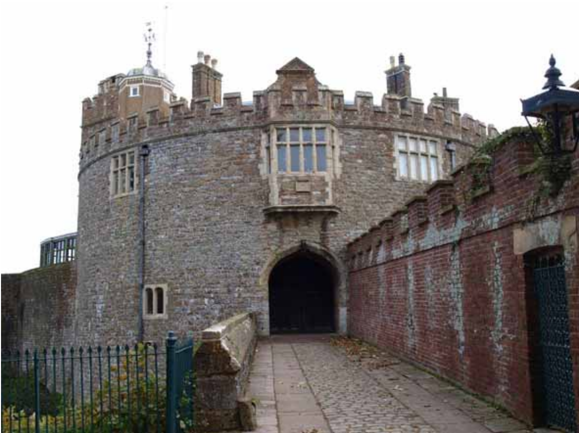
Figure 10. The north-east bastion which was heightened in the 1870s
