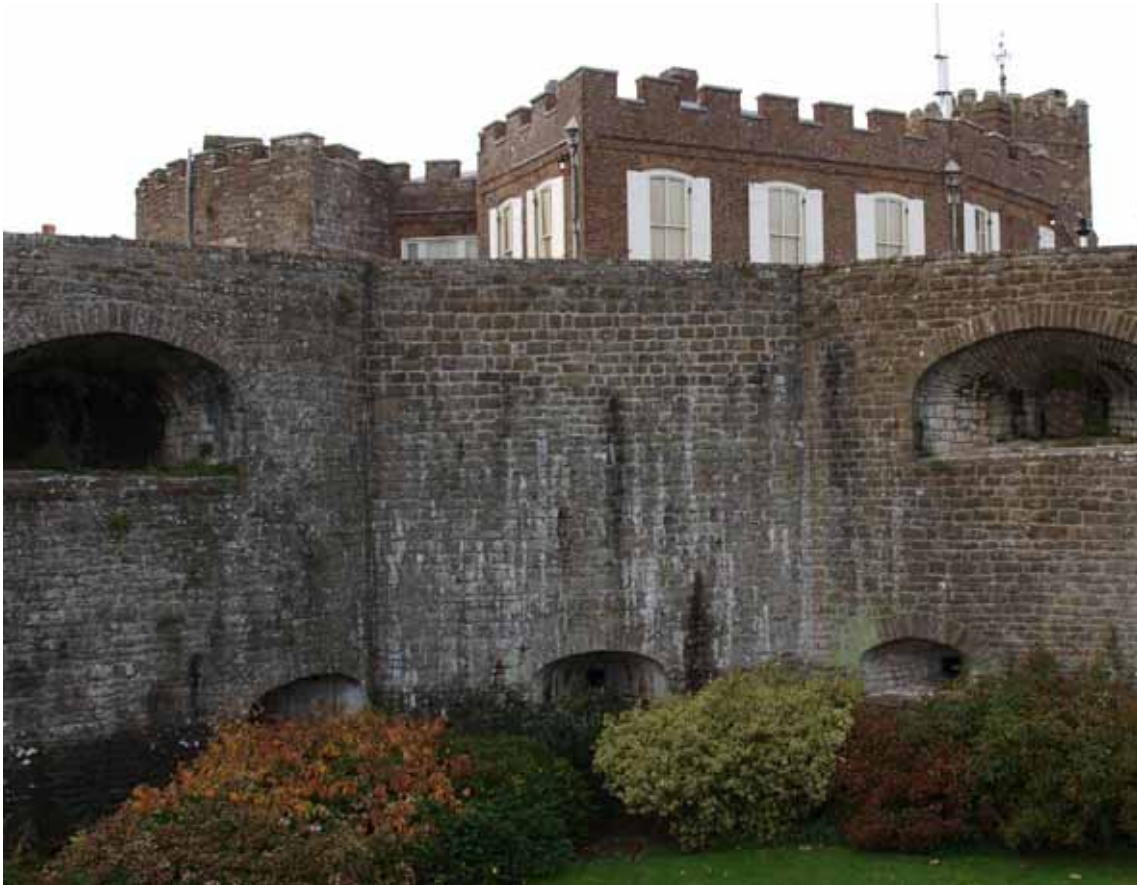
Figure 8. Brick-built rooms (F14 and F15) added to the north-east bastion in the early 18th century
