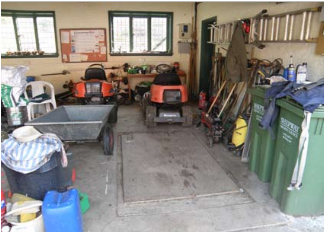
Figure 60. - The inspection pit within the motor house at Horton Court in Kent. Pete Smith P9222505.JPG
