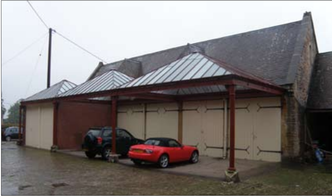
Figure 66. The glazed canopy added to the coach house designed by William Woodyer at Tyntesfield in Somerset when it was converted into a motor house. The two former coach houses to the south-east were extended forwards reputedly in the 1920s. Pete Smith P8252215.JPG
