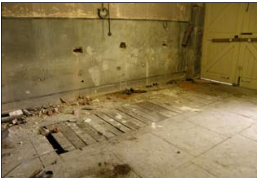
Figure 39. The inspection pit within the motor house at Nostell Priory in South Yorkshire built for Rowland Winn, 2nd Baron St Oswald, by the architect James MacVicar Anderson in 1904.
