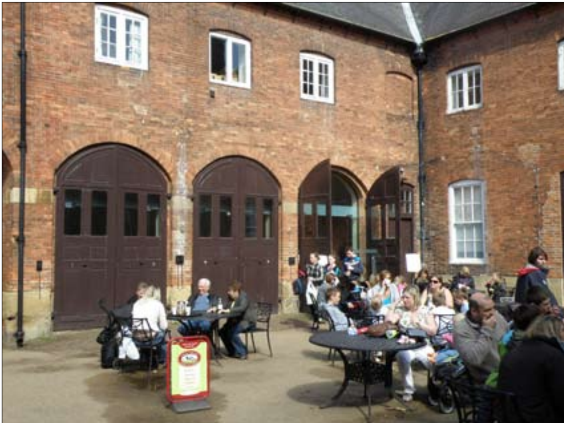
Figure 72. The former coach house at Wollaton Hall in Nottinghamshire built in 1743. The glazed panels inserted into the doors and the scar of a former glazed canopy are all that survives from its conversion into a motor house. Pete Smith P4080352.JPG
