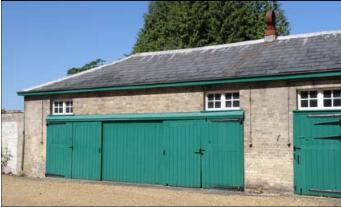
Figure 94. The stable range designed by Humphry Repton at Hoveton Hall in Norfolk, converted into garages with hinged and sliding doors in the early 20th century. Pete Smith P6040757.JPG
