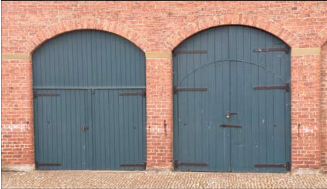
Figure 102. The doors of the former coach houses at Sion Hill Hall in North Yorkshire cut down to accommodate motor cars. Pete Smith P6070885.JPG
