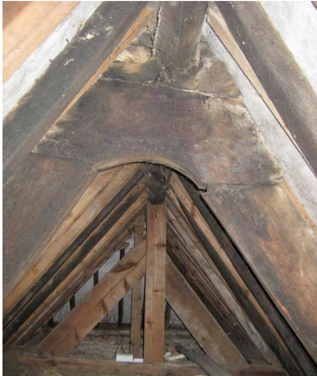
Figure 5: East face of truss A
