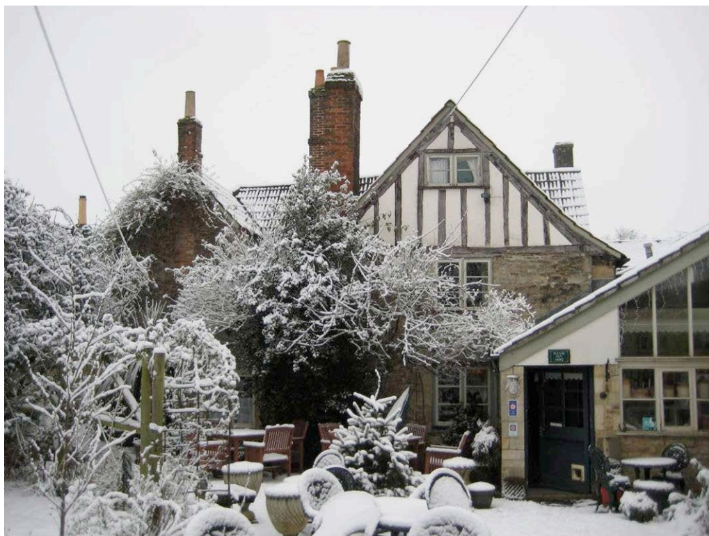
Figure 4: The south-east wing gable of King John's Hunting Lodge viewed looking north
