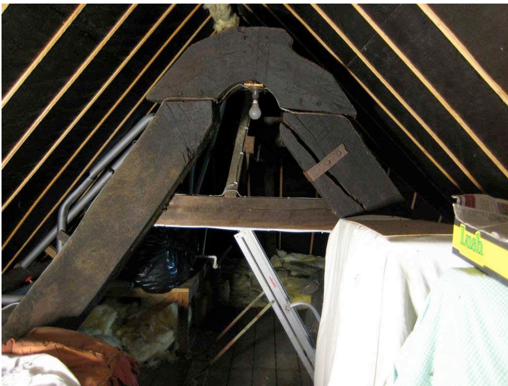
Figure 6: Truss C south face
