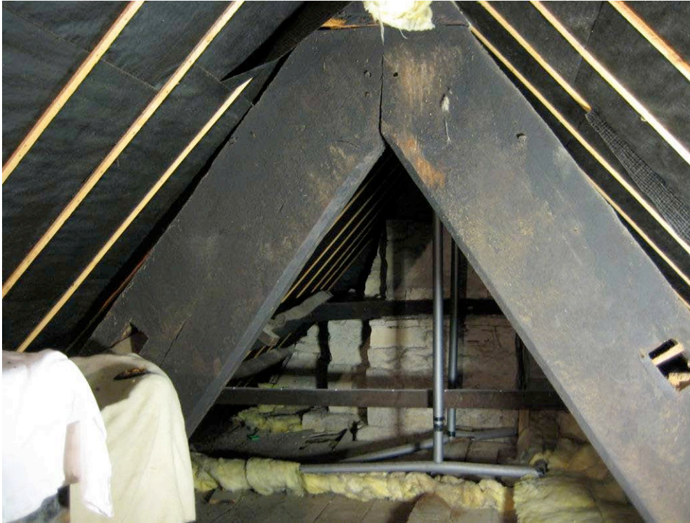
Figure 5: Truss B north face
