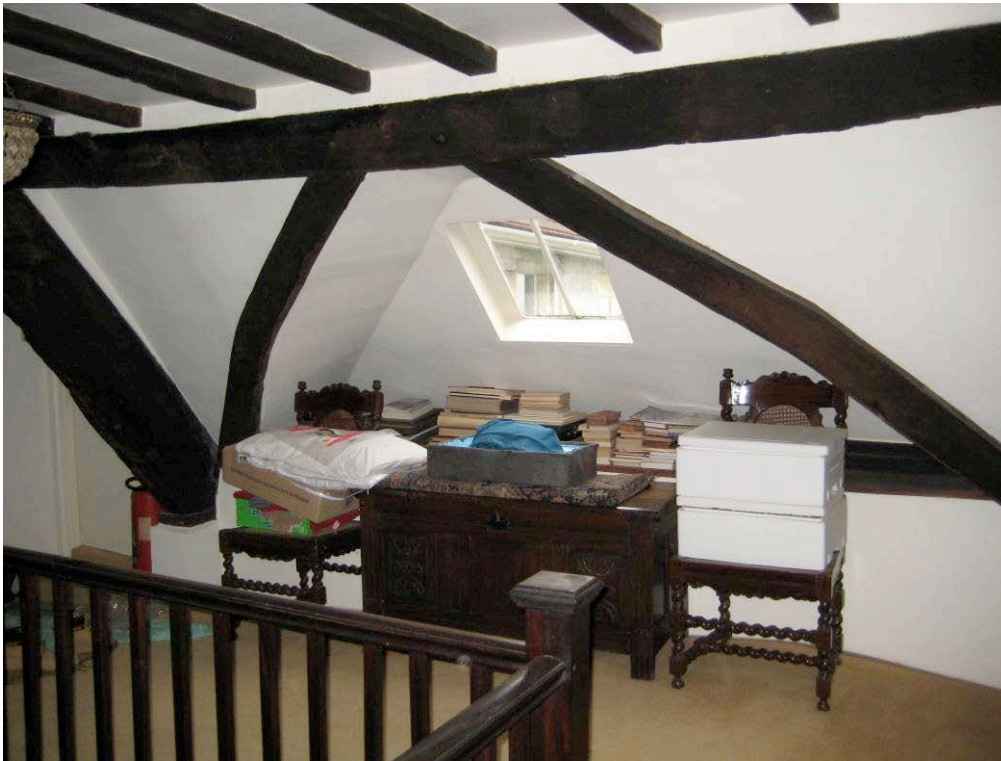
Figure 7: East windbraces in bay 2
