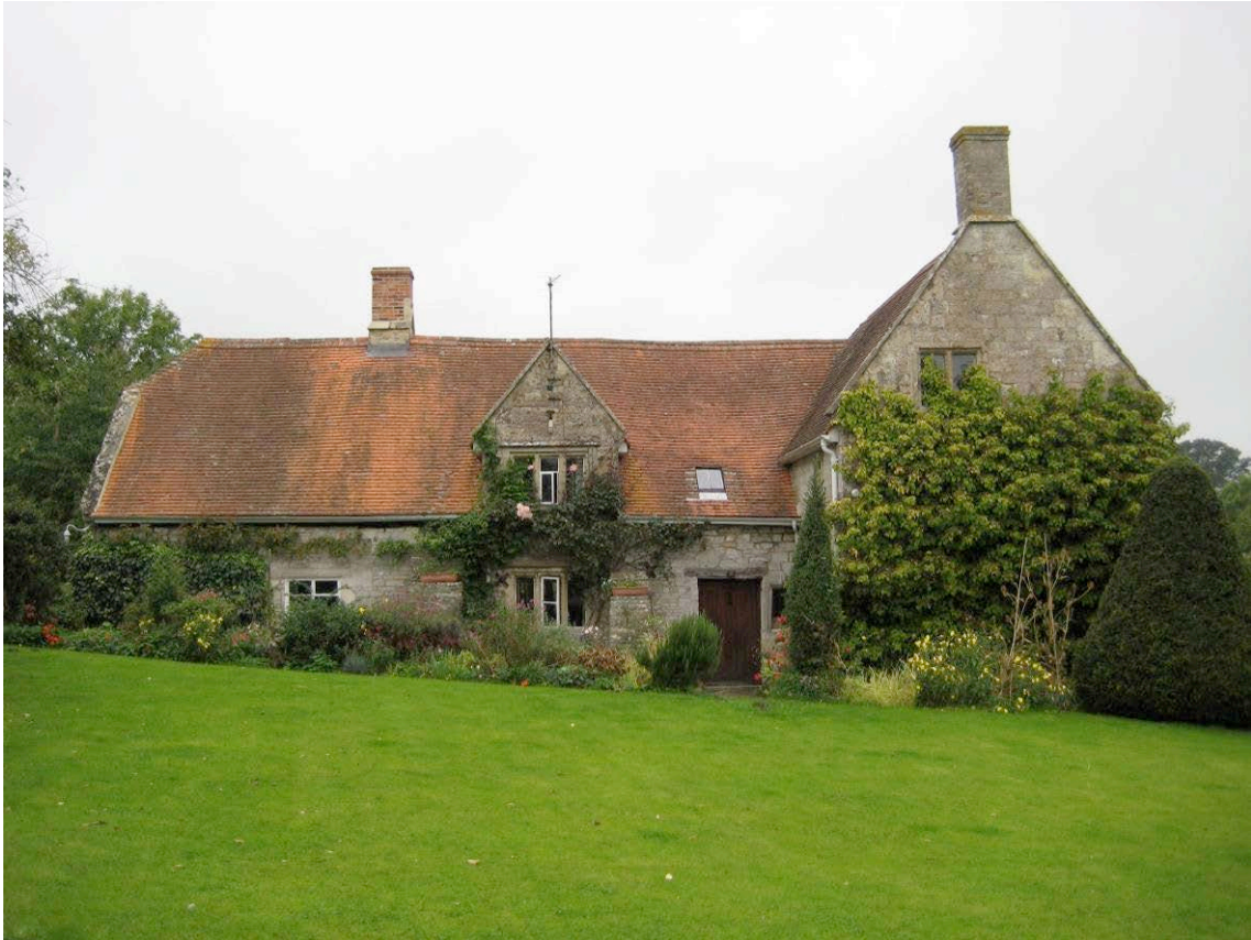
Figure 3: East elevation of Apshill House
