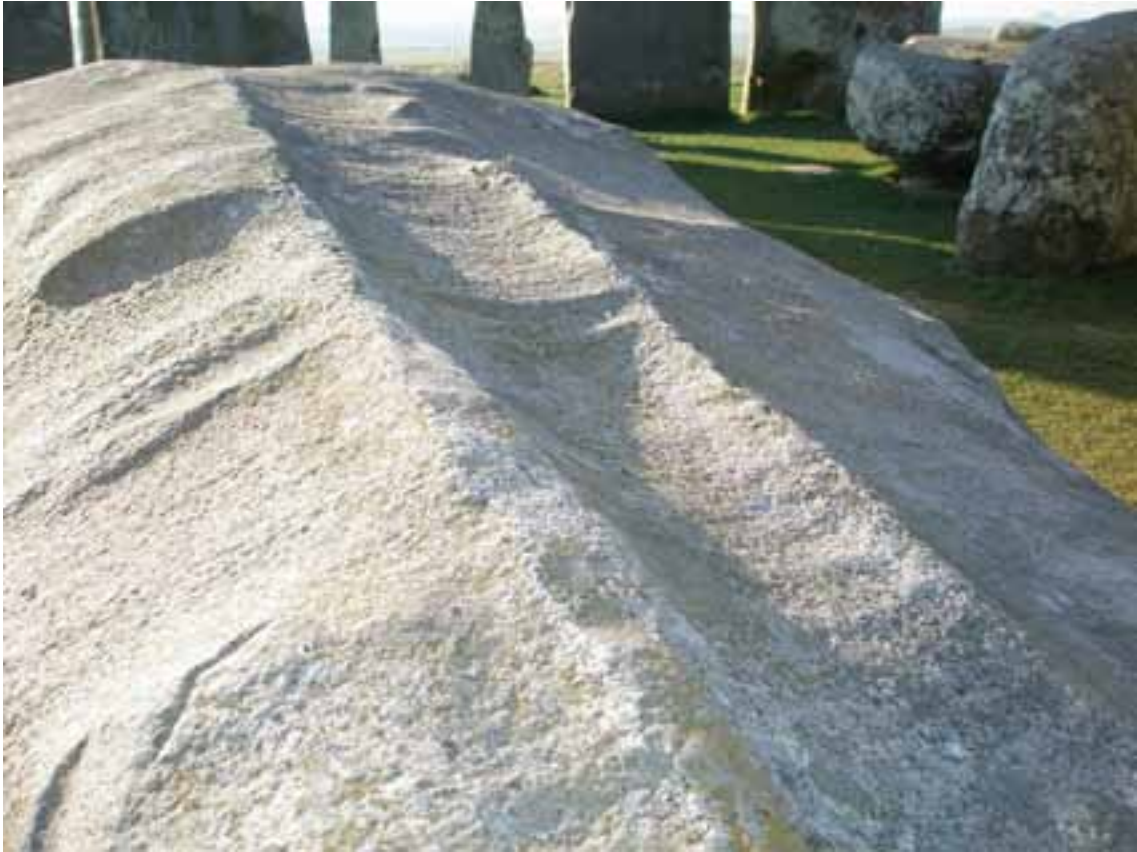
Figure 14. Unfinished stone 59, showing the method of dressing. In an unweathered condition the sarsen can be easily pecked and ground into shape. Here the grinding has been carried out in narrow strips the length of the stone leaving arrises standing proud which could then be ground down in the next stage of the operation. Grinding in this fashion must have been carried out when the stone was flat on the ground, but this stone was broken when it fell so must have been erected in this state. Gaffer Hunt kept a cellar containing 'liquors to entertain the traveller' beneath the stone during the eighteenth century.
