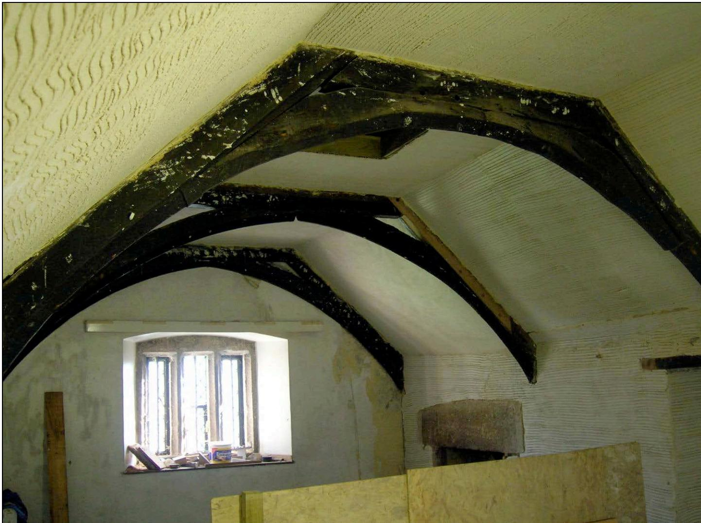
Figure 10: East range roof; trusses 1 and 2 (truss 2 in foreground, truss in gable end is false)
