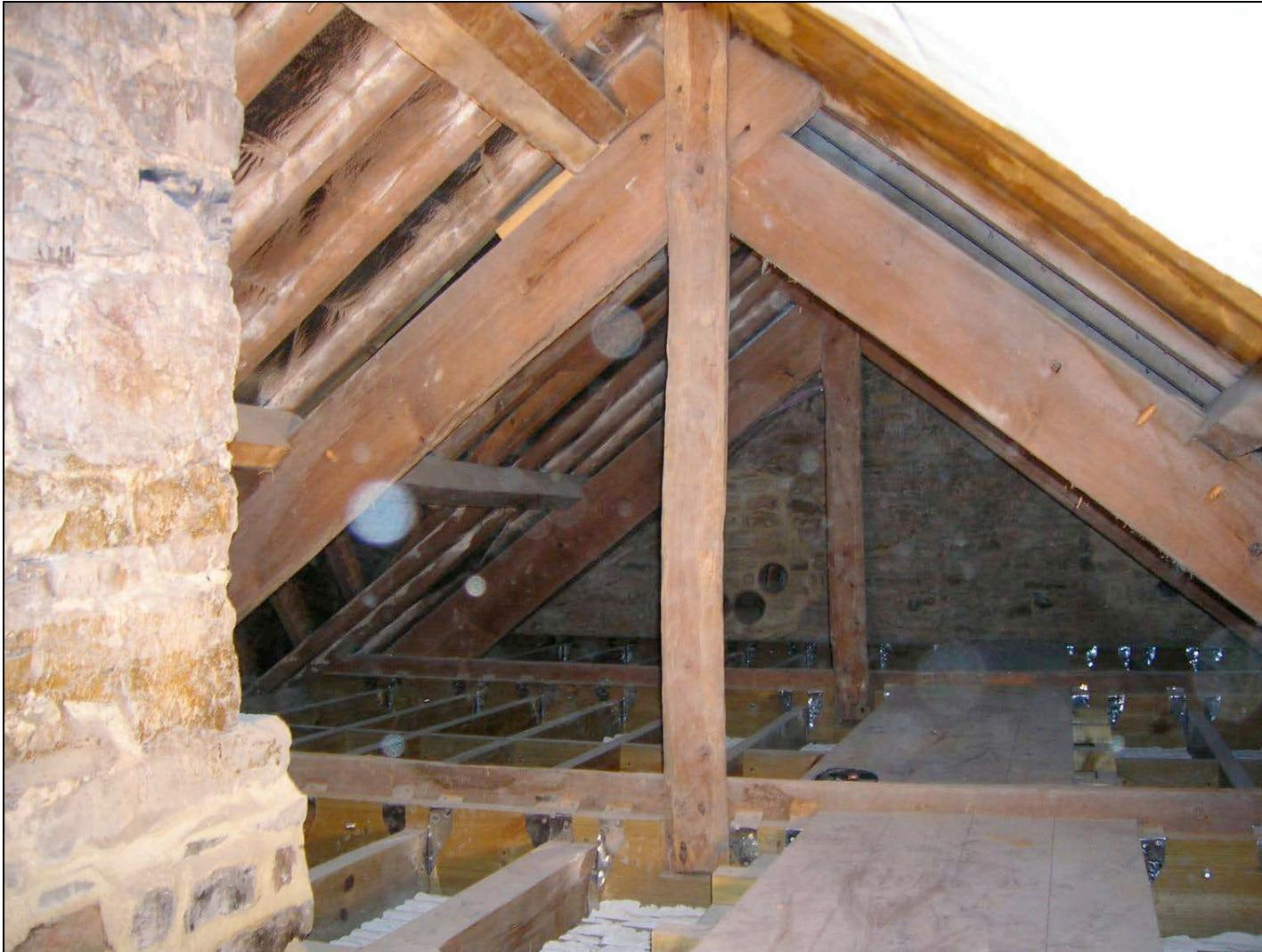
Figure 7: Central range; roof taken from the south-west (truss 2 in foreground)
