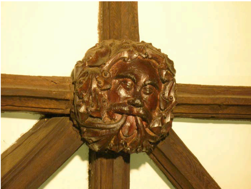
Figure 6a (top): View of Law Library roof
