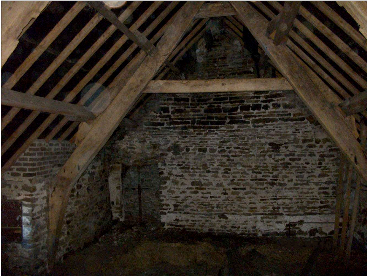
Figure 7: East range; roof (truss 2, photograph taken from the north-east)
