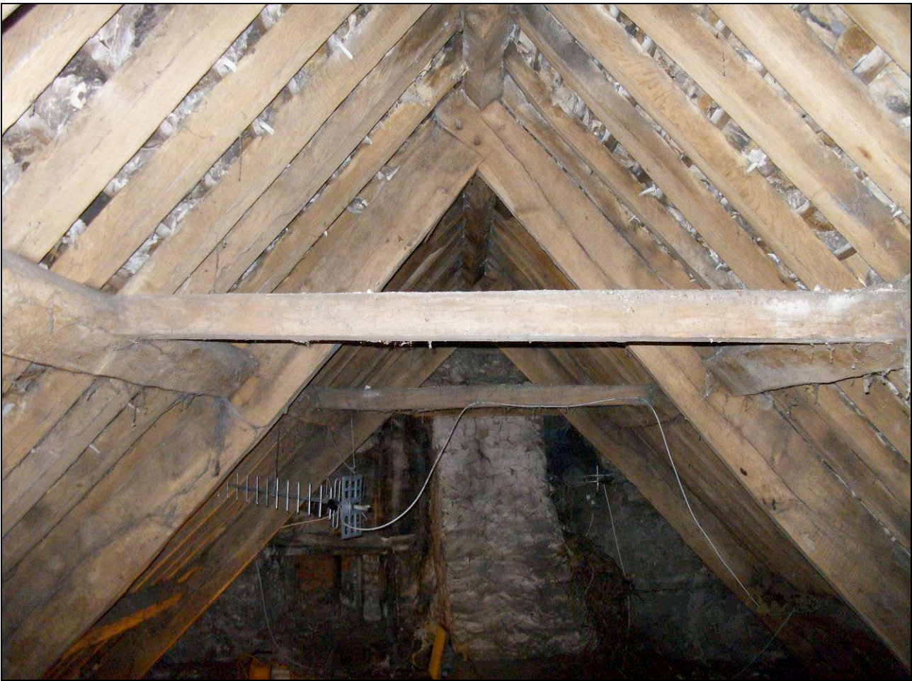
Figure 6: Central hall/parlour range; roof (photograph taken at truss 1, looking south-west)
