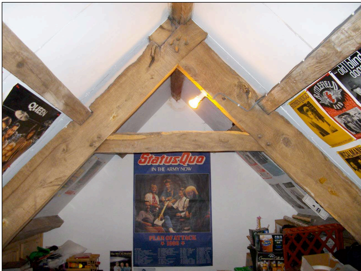
Figure 10: West range; roof (truss 1, photograph taken from the south-west)
