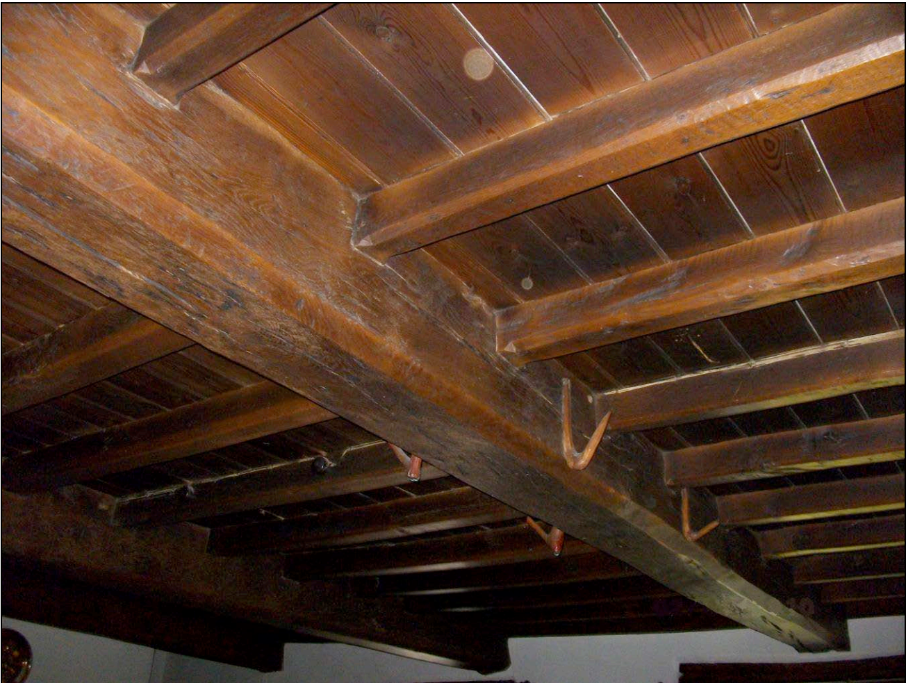
Figure 5: Central hall/parlour range; ceiling (photograph taken from the east)
