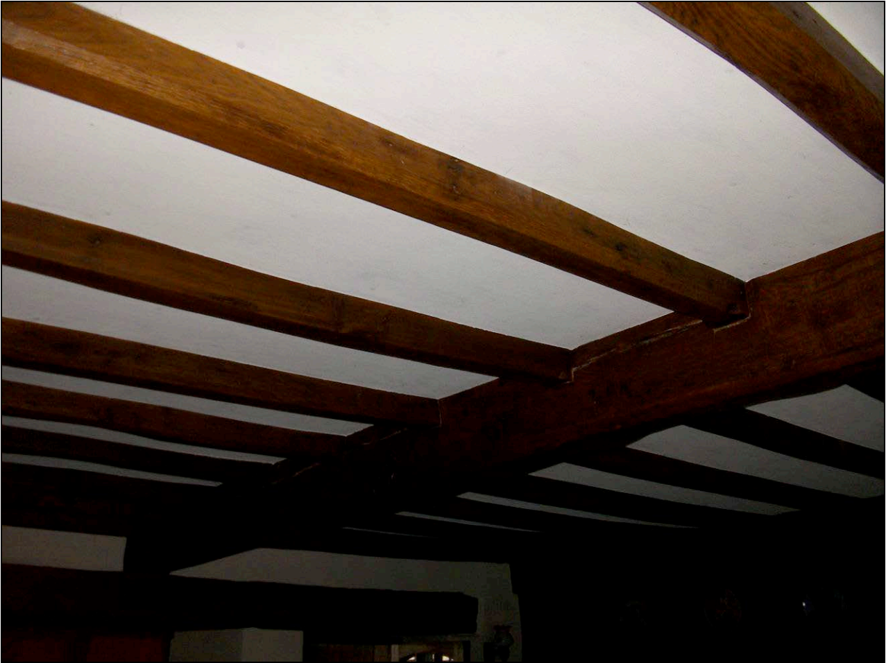
Figure 9: West range; ceiling (photograph taken from the east)
