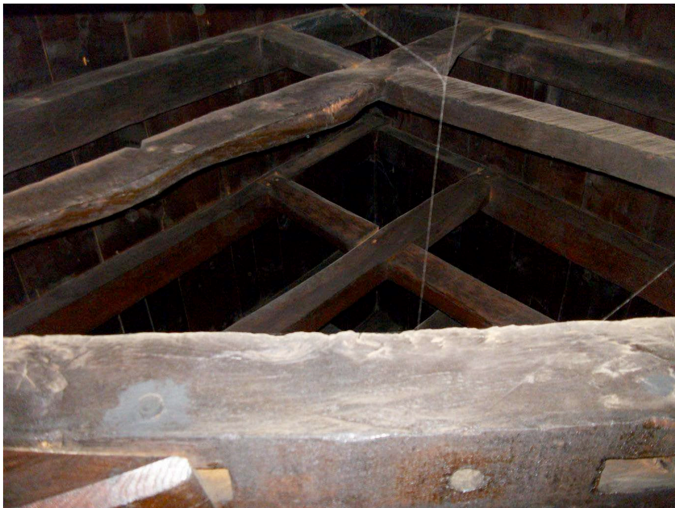
Figure 5: Photograph taken of roof, collar upwards
