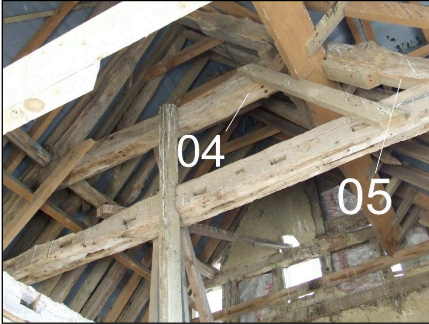
Figure 4. Photograph (by author) of the central truss, showing timbers sampled for dendrochronology
