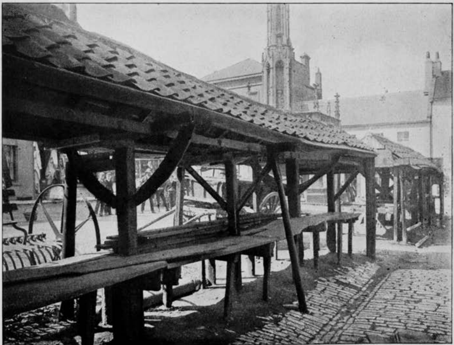
FIG. 2. The Shambles at Shepton Mallet: internal structure.
