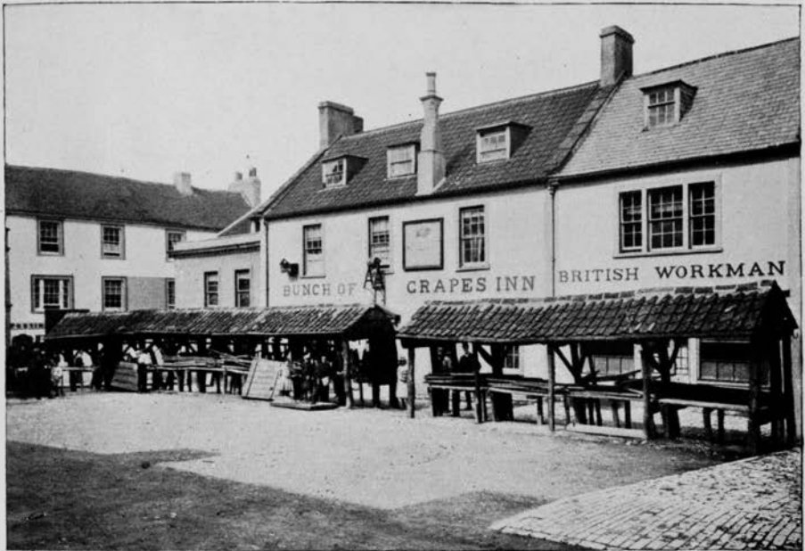
FIG. 1. Medieval Shambles at Shepton Mallet: general view.
