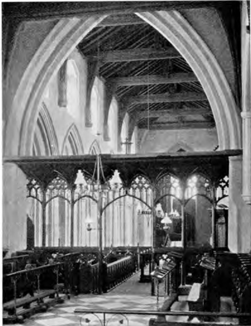
Over. East side of rood screen shewing the vaulting.
