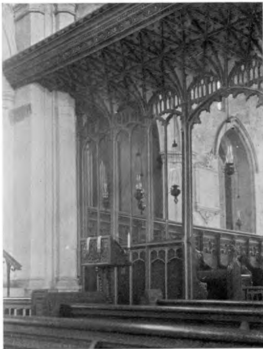
Balsham. Part of west face of rood screen shewing projecting canopy.
