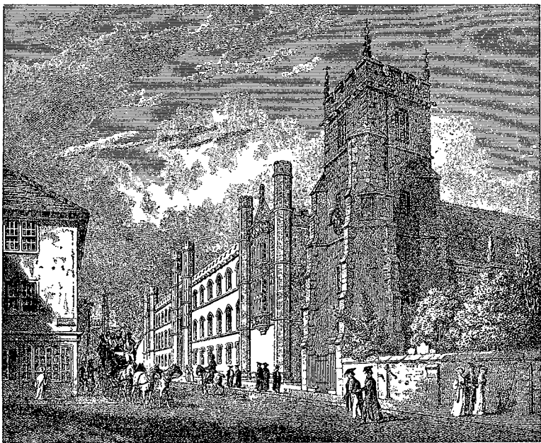
Fig. 6. Cambridge, St Botolph's Church. Compound octagonal buttress irregularly set out (cf. pl. X).
