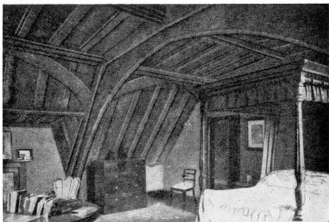
ELY: PRIOR'S HOUSE. The kerb roof of the hall.
