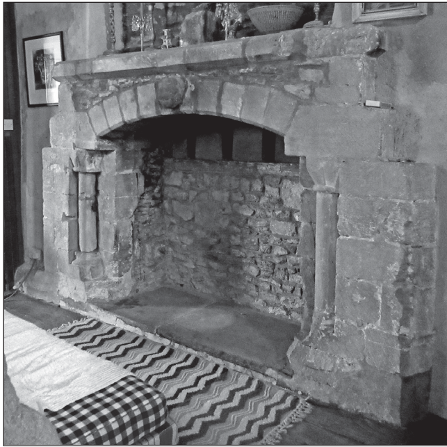
Figure 9. The first-floor fireplace.
