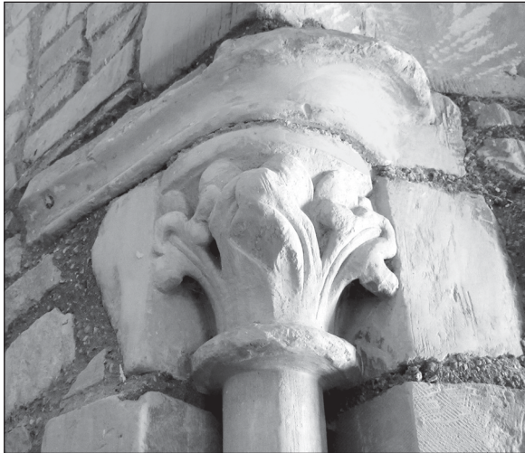
Figure 27. Stiff-leaf capital and moulded impost to interior of northern window.
