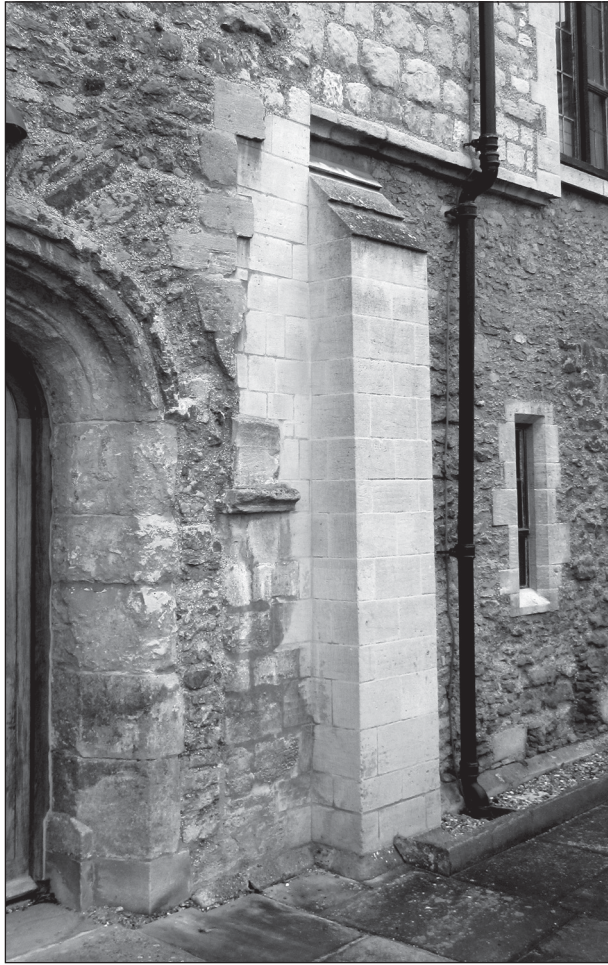
Figure 29. Detail of former archway, with impost block.
