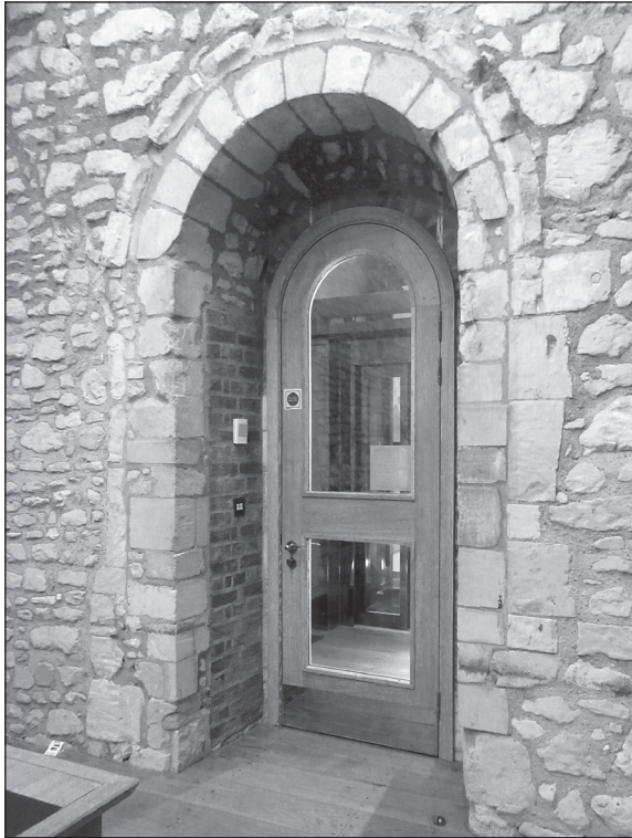
Figure 31. The first-floor doorway into the north wing.
