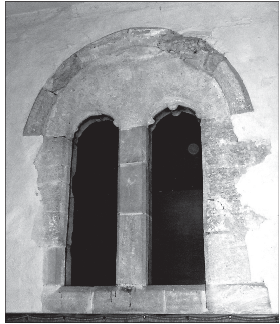
Figure 10. Original exterior face of the first-floor window in the east wall.
