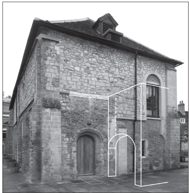
Figure 28. East gable with reconstruction of original arched stair platform.
