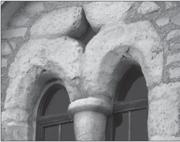
Top: Figure 23. Northern first floor window. Above: Figure 24. Detail of northern window, with crossed rib decoration to arched heads and pierced spandrel.
