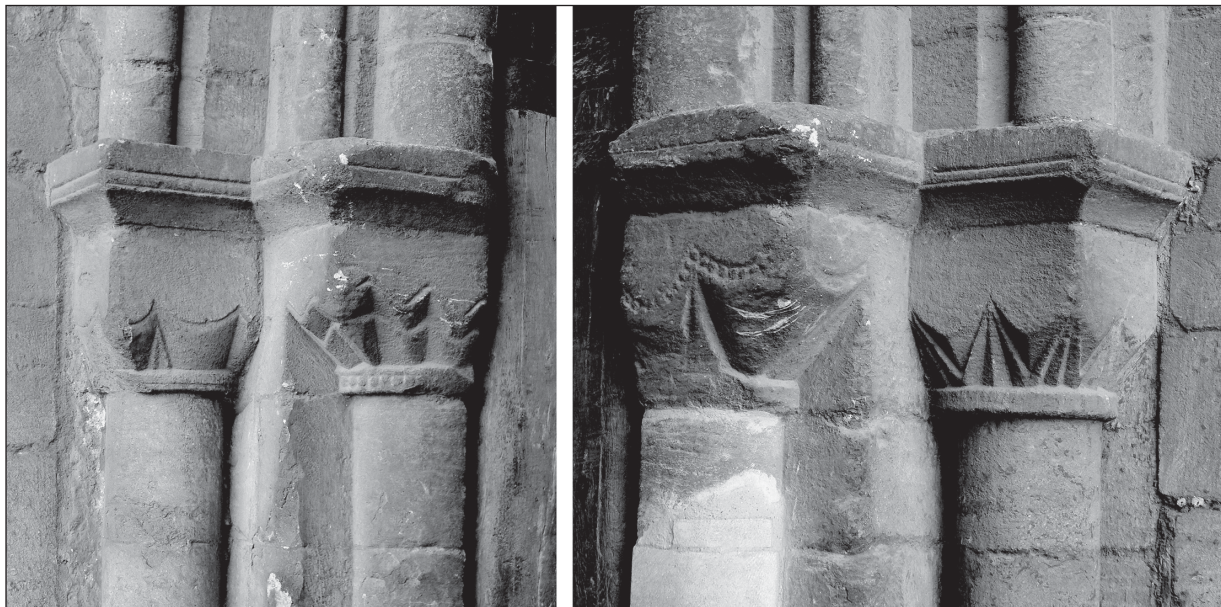
Figure 5. Scallop capitals on north and south jambs of the outer arch of the western gate-house of Peterborough Abbey. Photographs D Stocker.
