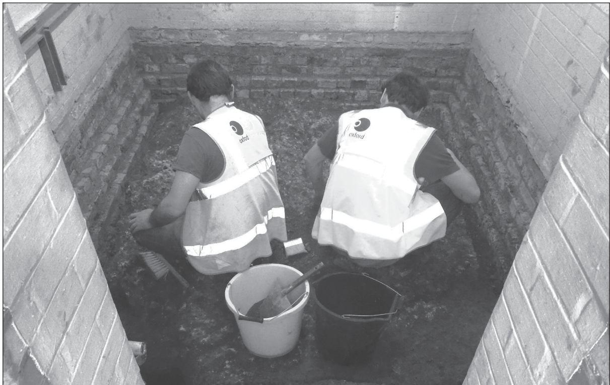
Figure 2. Excavation in the lift shaft.
