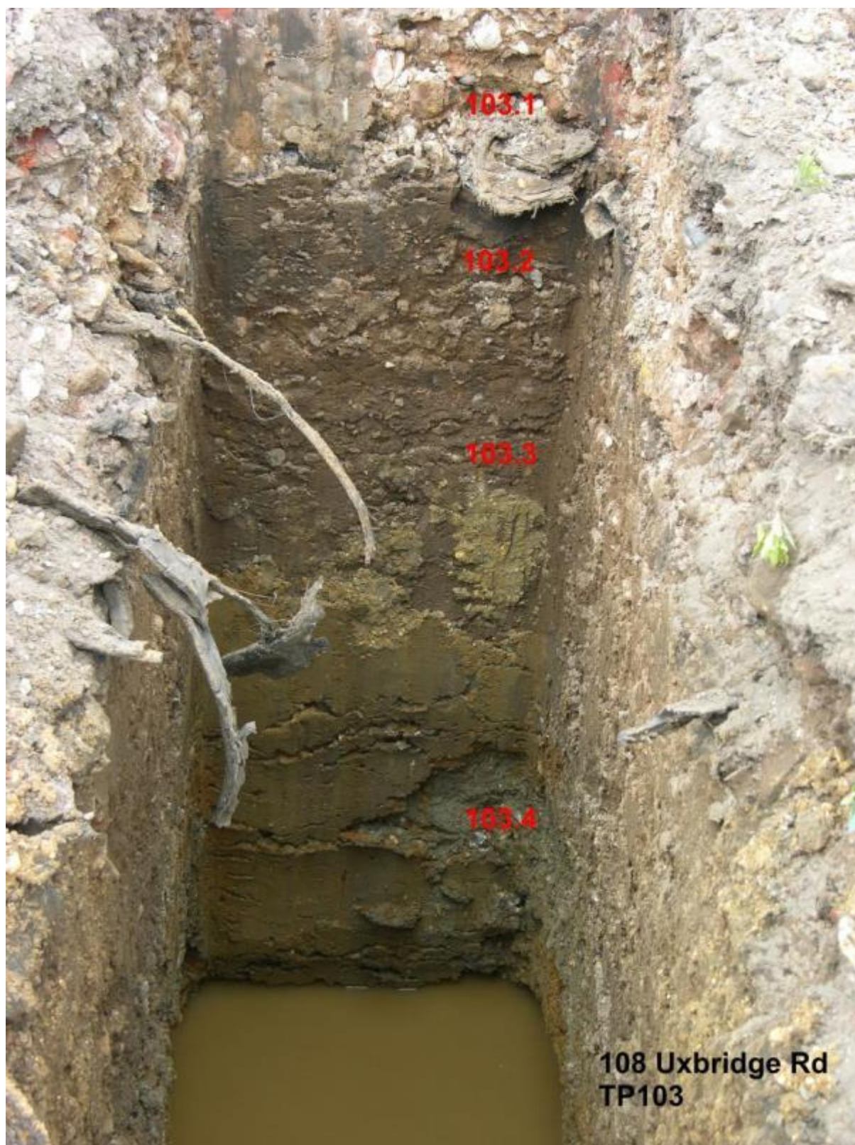
Figure 8: Trial pit TP103, annotated photograph.
