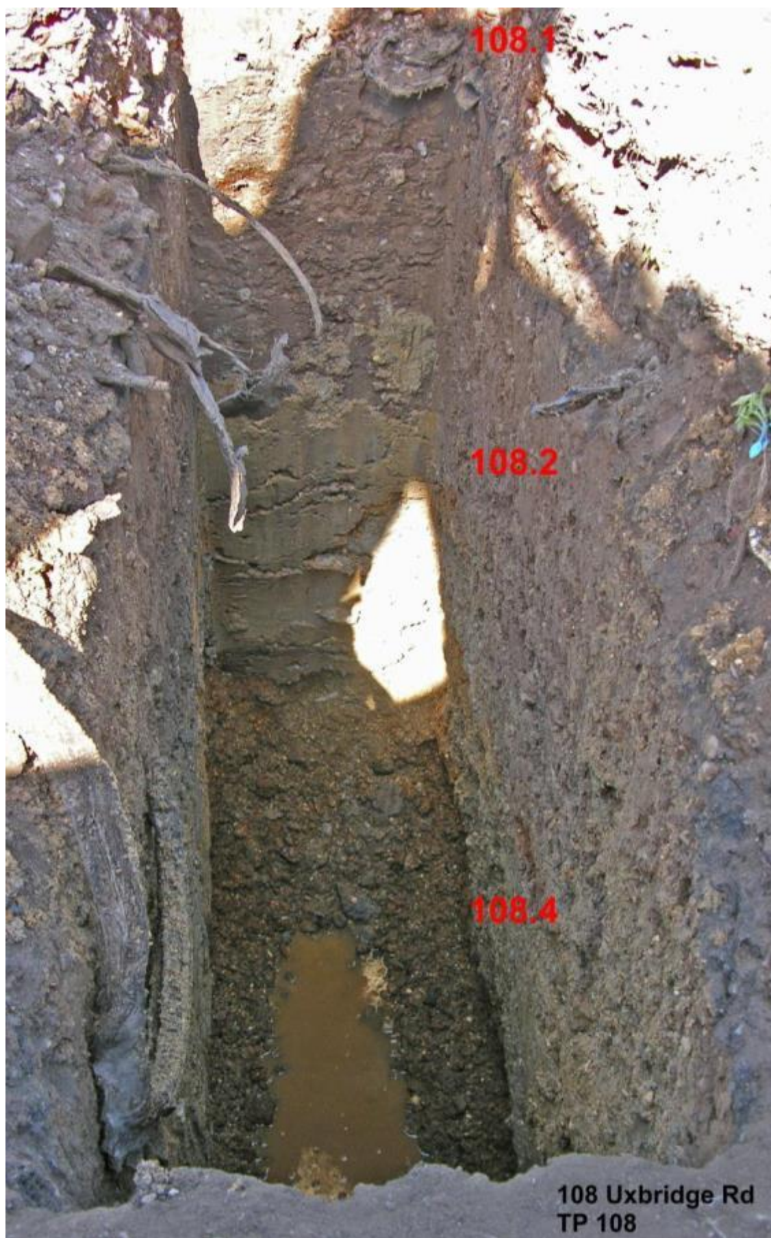
Figure 18: Trial pit TP108, annotated photograph.
