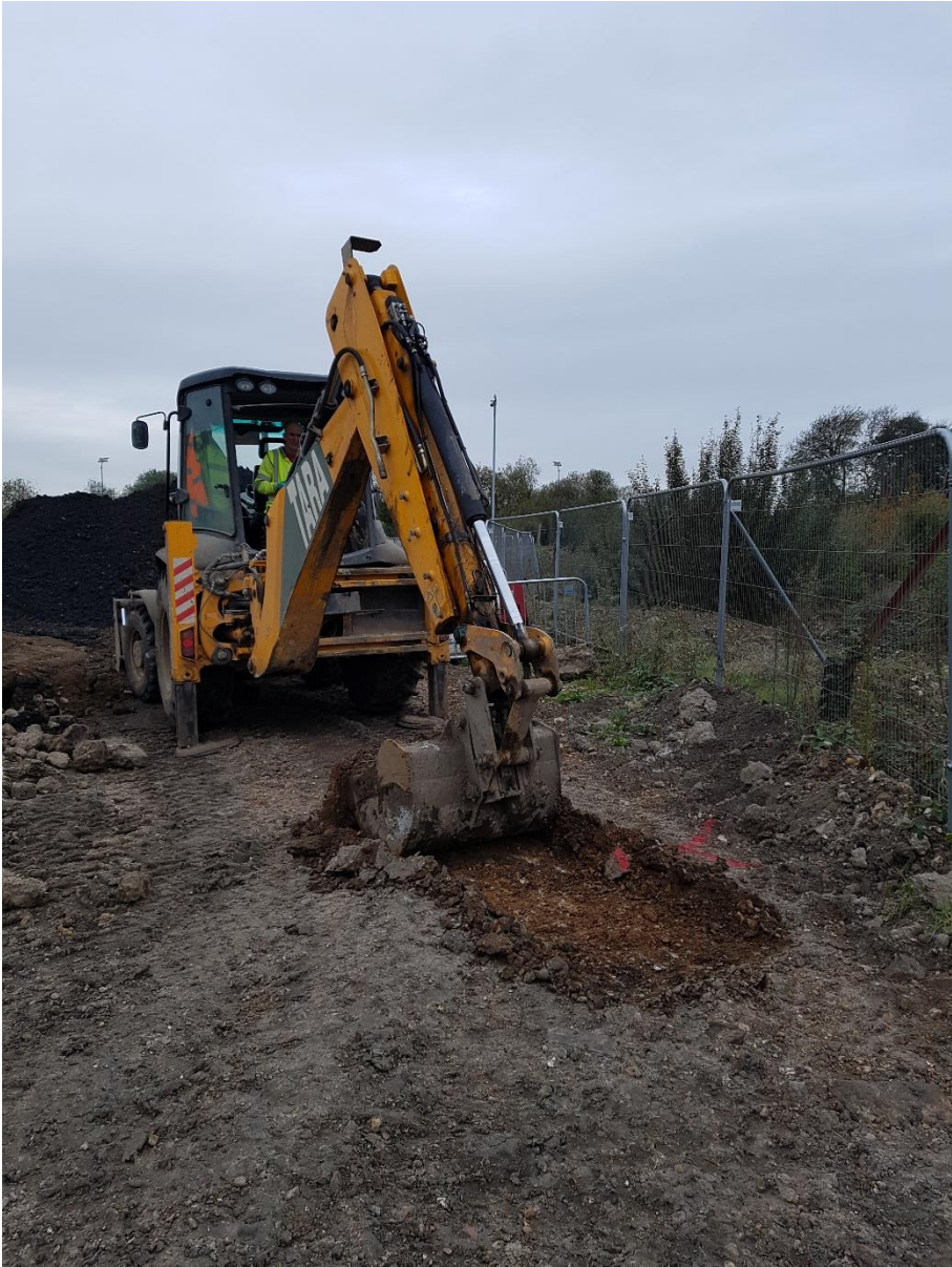
Figure 7: Photograph of Test-pit TP5, Southall Gasworks
