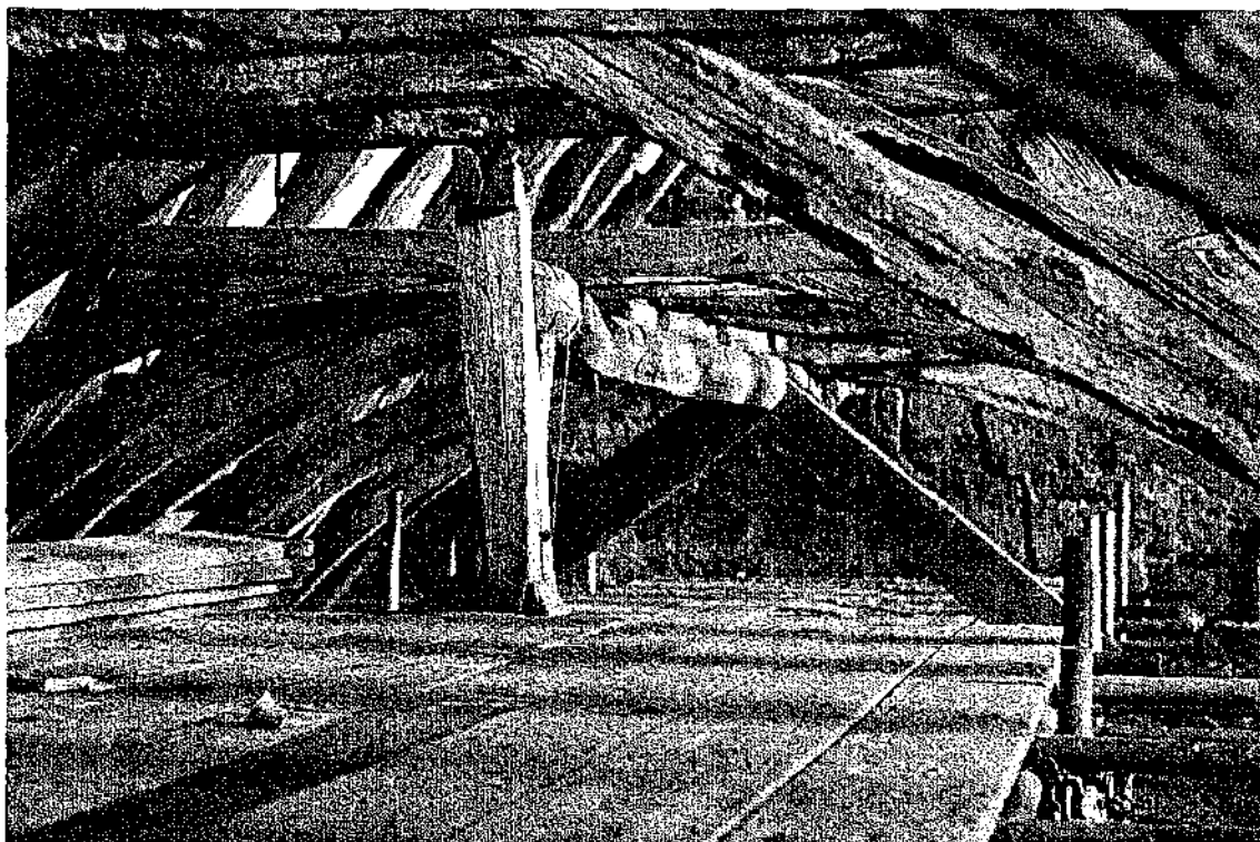
Plate 12 Structure 1, detail of the curved soulaces of the common-rafter roof (Stereberg).
