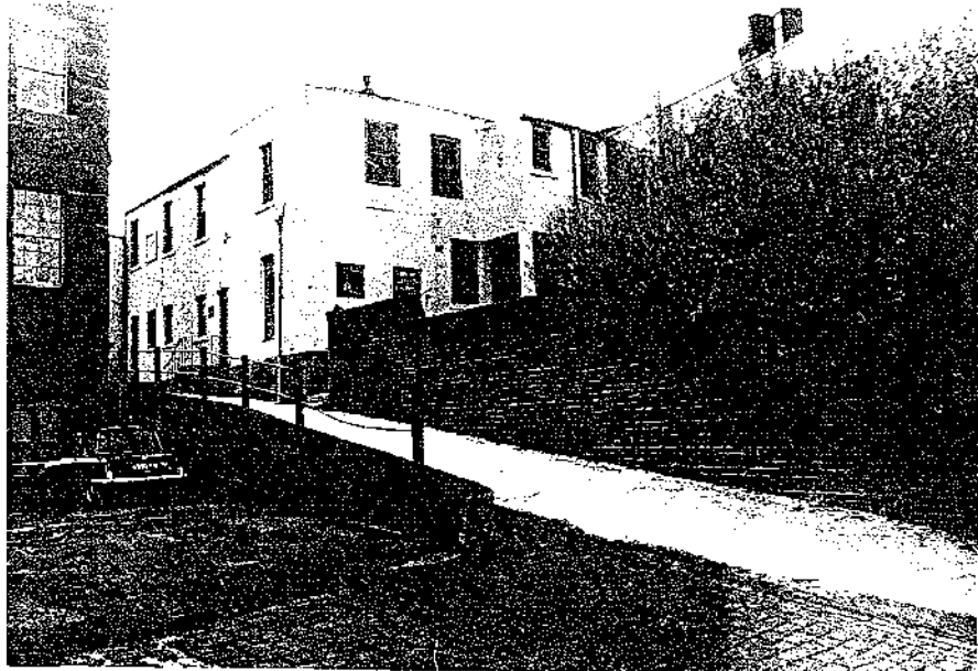
Plate 2 The demolished buildings, view south
