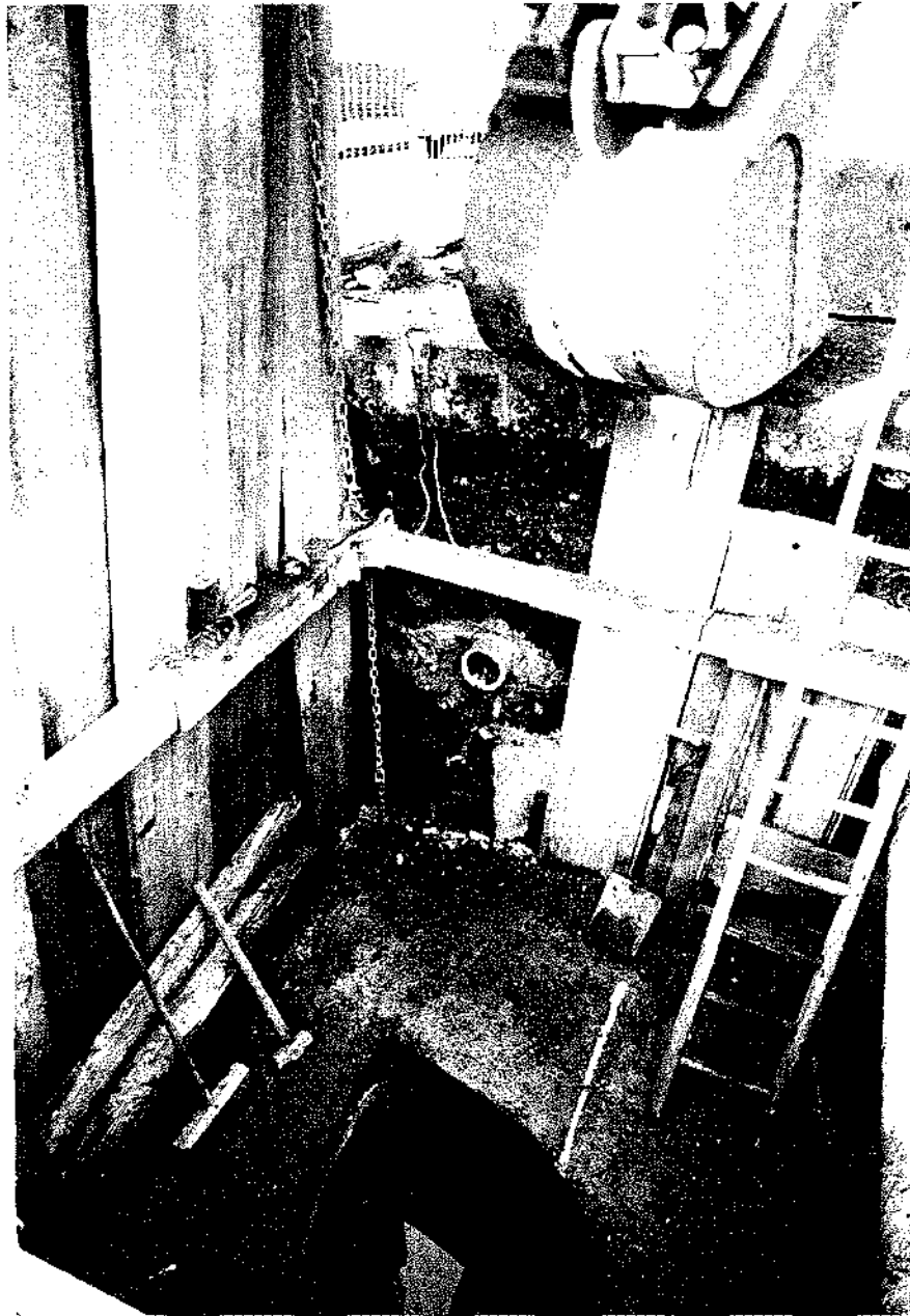
Plate - Manhole (M10) in Crown Street (Photo by E. Newton).
