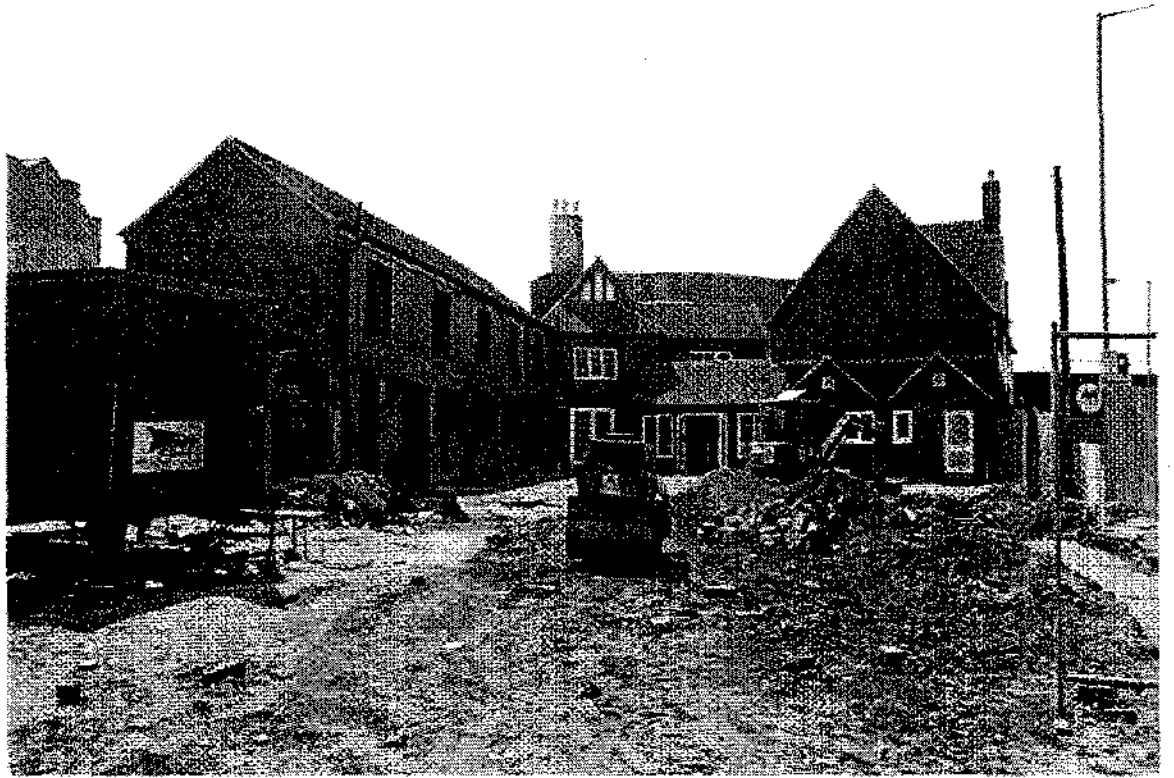
Plate 5: Removal of deposits overlying blue-brick pavement surface.
