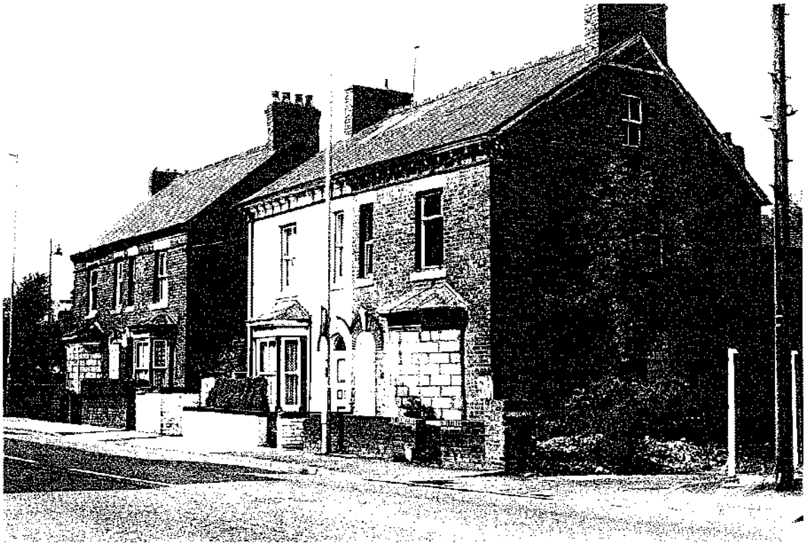
Plate 9: 47-53 Littleton Street West.
