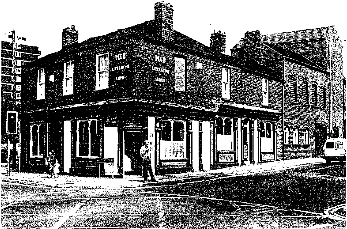
Plate 11: The Littleton Arms. Littleton Street East.
