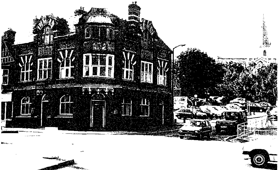
Plate 12: The Borough Arms Ablewell Street/Upper Rushall Street.
