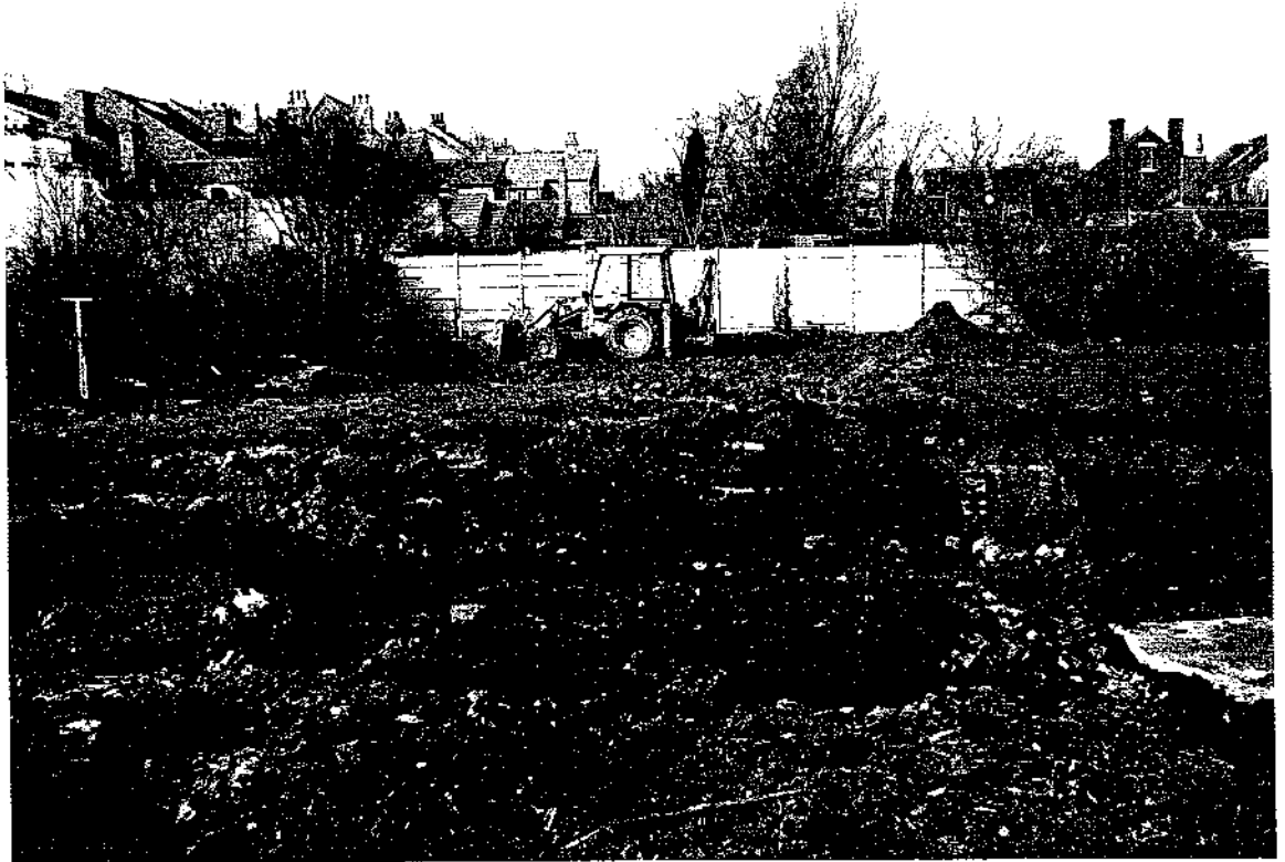
Plate 1: Topsoil Stripping in Areas 1 and 2.
