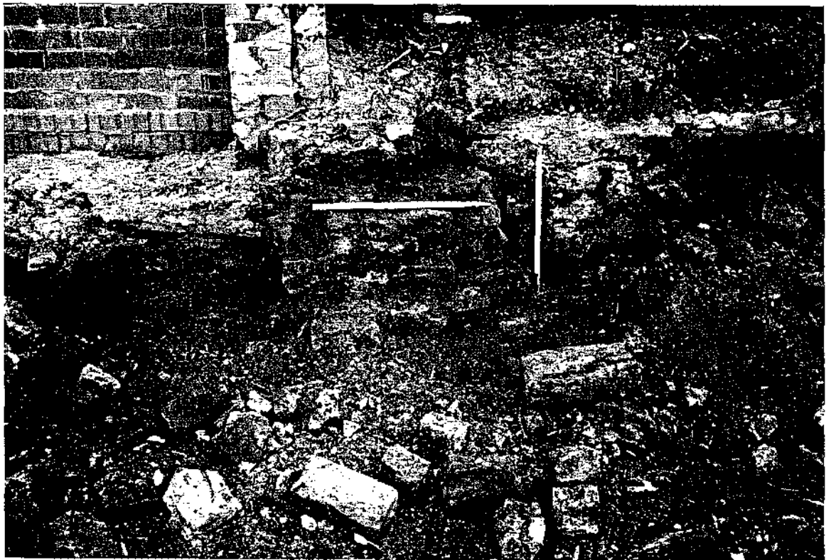
Plate 2: Section 3, detail of sandstone wall
