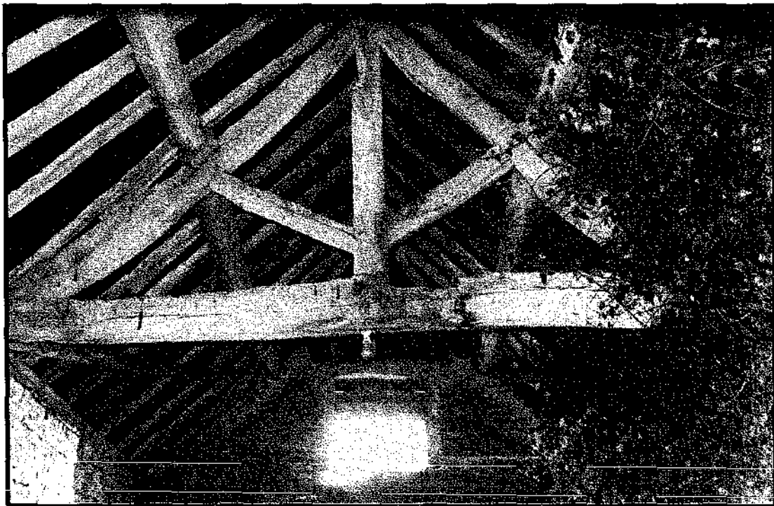
Plate 5 Barn 2, internal roof detail
