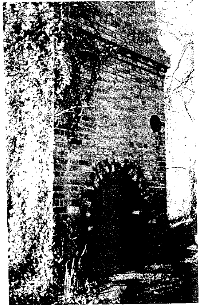
Plate 6: Detail of Chimney Flue Arch
