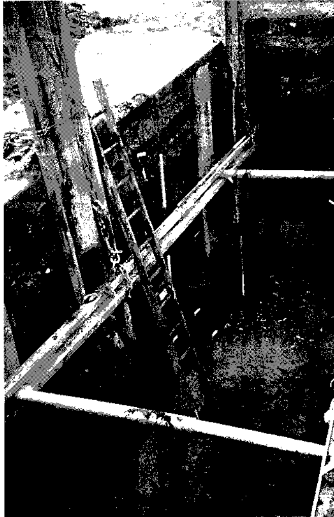
Plate 1. Trench 1. General view of south end of trench.
