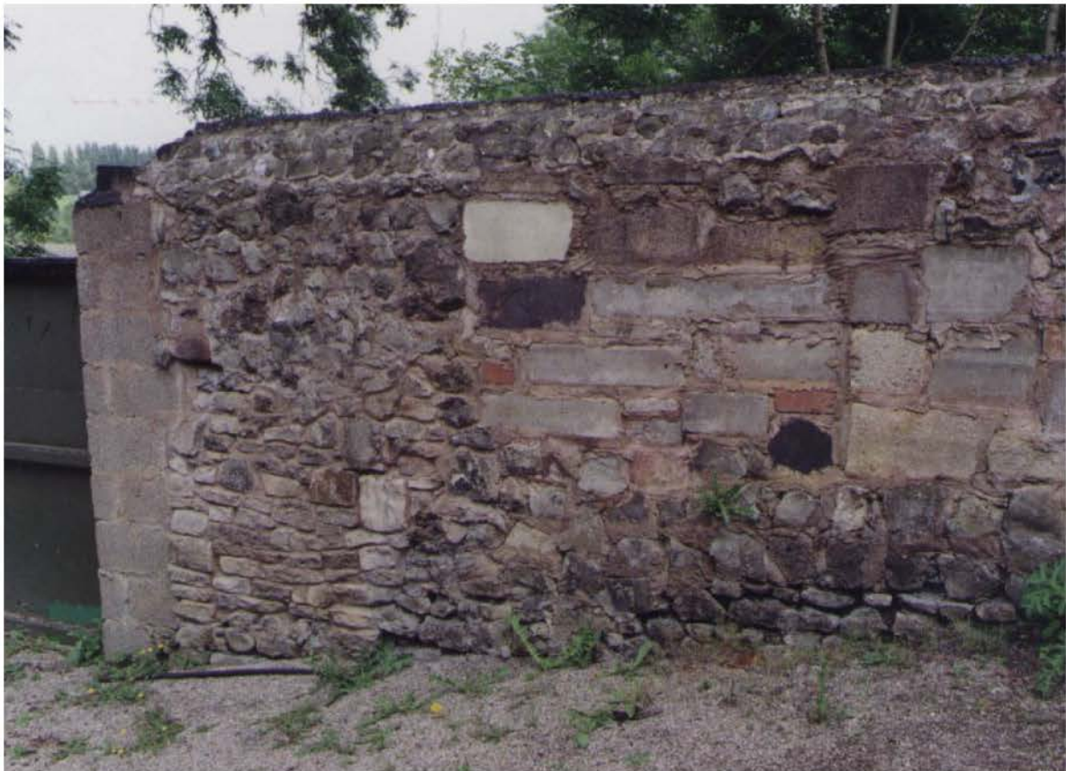
Plates 6 & 7 The heavily breached and patched section of original Castle Grounds' walling it is proposed to retain (Dr Paul Collins)
