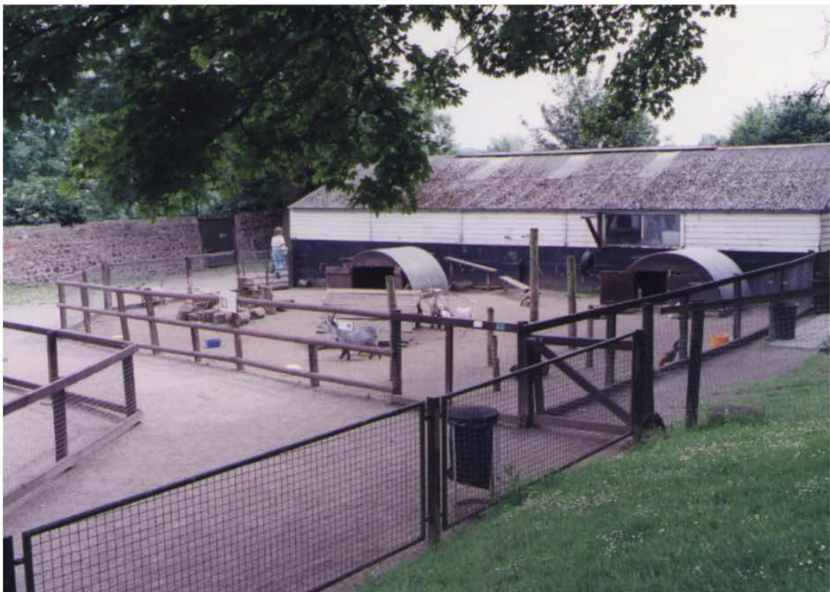
Plates 8 & 9 The 'Farmyard' buildings currently occupying the site of the proposed new Elephant House (Dr Paul Collins)
