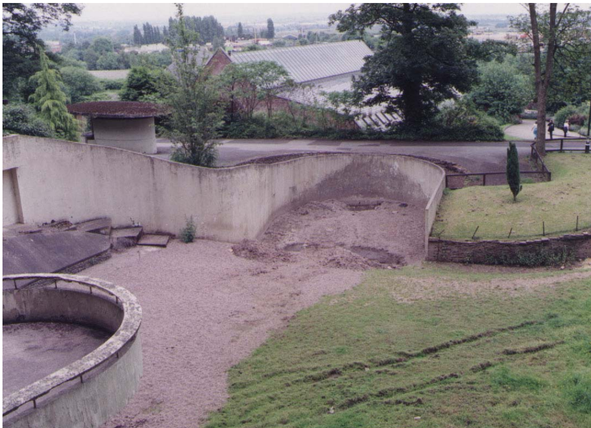
Plate 4 The original Bear Ravine pool was accommodated within the circular projection in the enclosure's perimeter walling. Its circular outline can be seen here (Dr Paul Collins)
