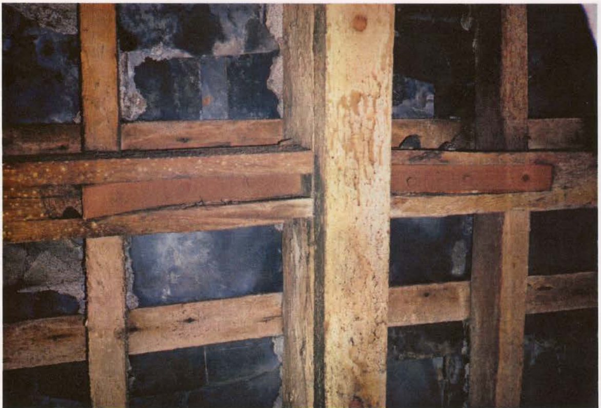
Plate 8 Detail of purlin tie, roof structure, Building F
