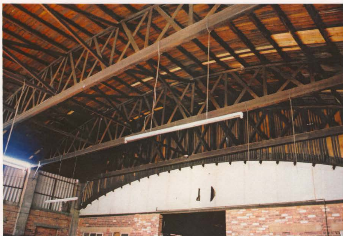
Plate 10 Belfast-truss roof, Building J
