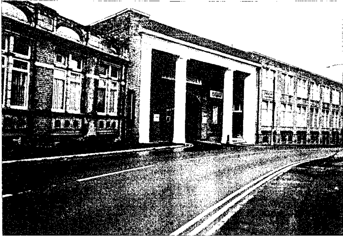
Plate 11 Gatehouse and office block (14) from the SE
